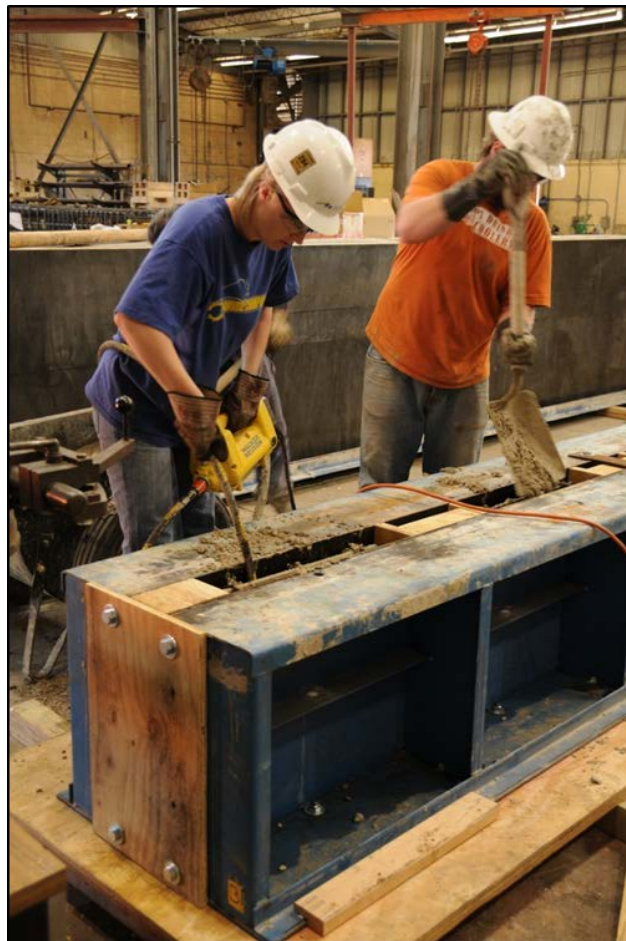
Figure 3-8: Panel Casting and Internal Vibration Procedure
