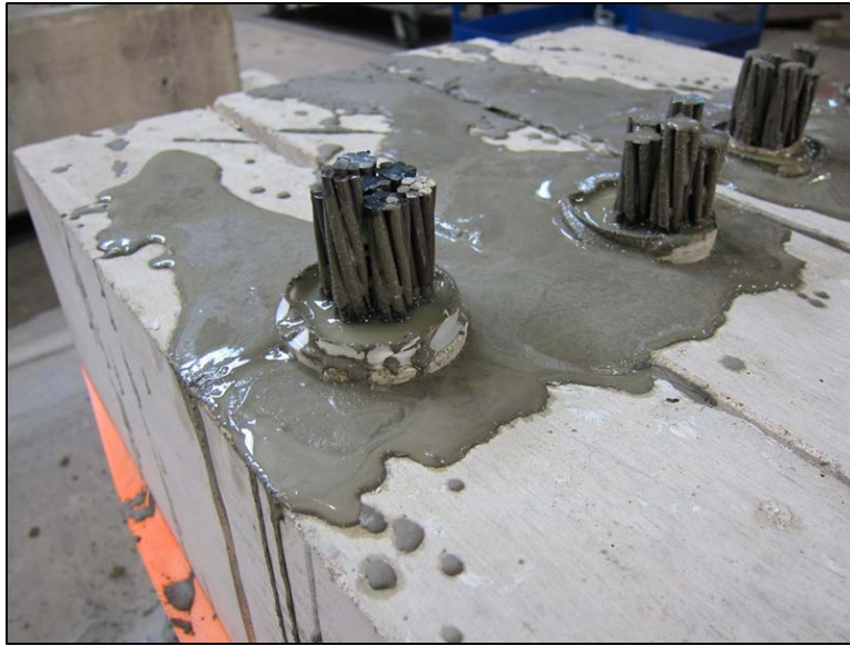
Figure 3-11: Duct Grouting Procedure
