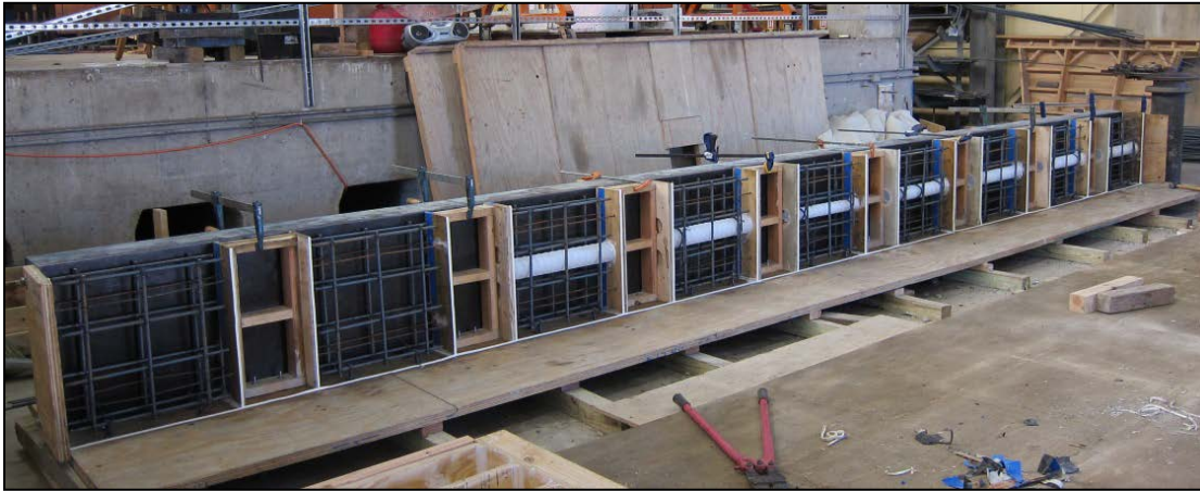
Figure 3-1: Formwork for Panel Casting
