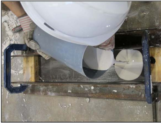
a) Placement of hydrostone
