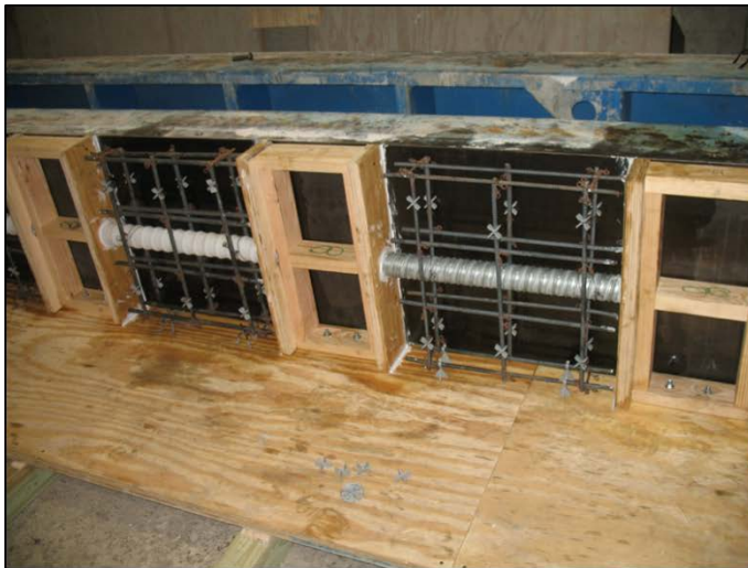
Figure 3-2: Panel Form Spacers
