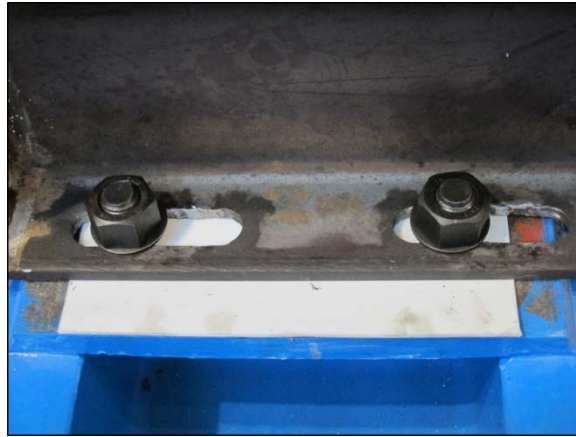
Figure 3-17: Connection Between Frame Beam and Brace Beam
