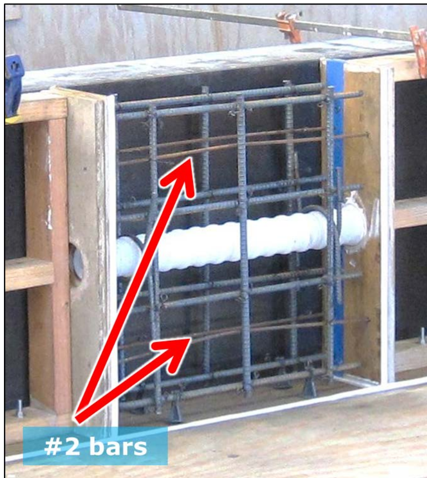
Figure 3-7: #2 Bars for Mesh Reinforcement Support
