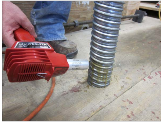
Figure 4-7: Application of Wax Bond Breaker to Steel Ducts
