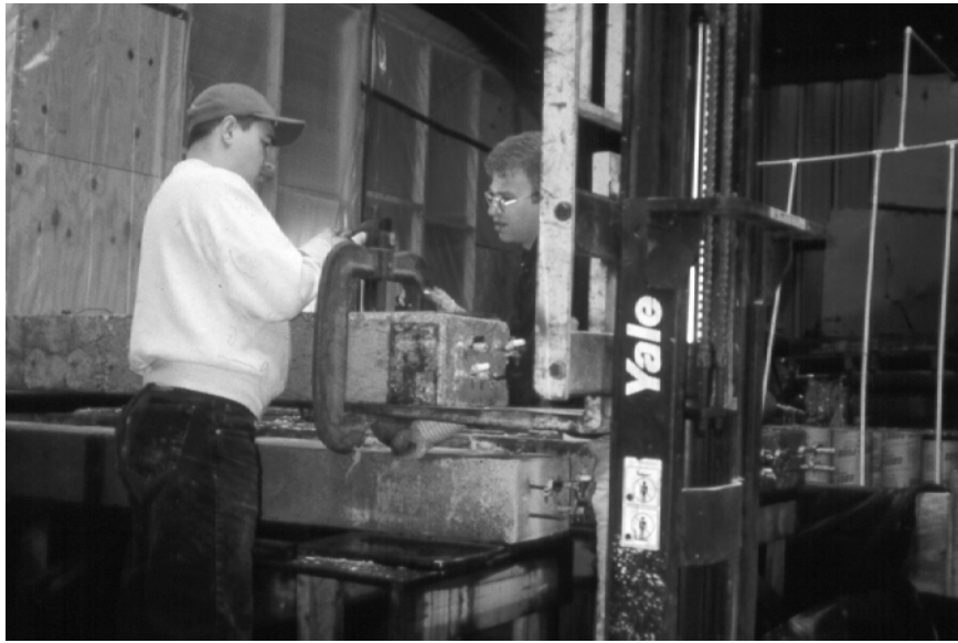
Figure 4.3. Placing the Beams on Wood Stands in the Retaining Pool.
