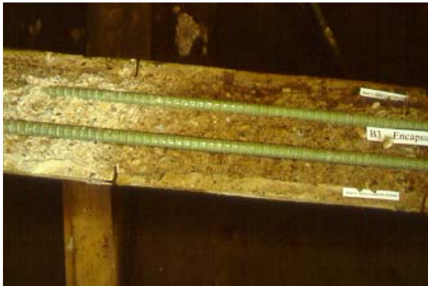
Figure 5.9. Difference in Appearance of Concrete in Beam 3.
