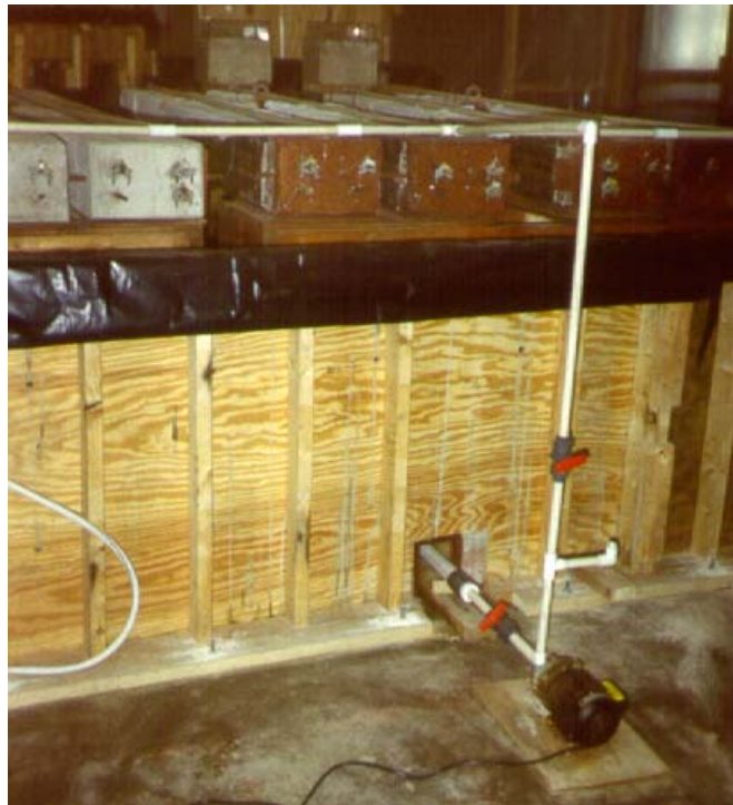
Figure 4.4. Retaining Pool, Recirculation Pump, and PVC Distribution Pipes.
