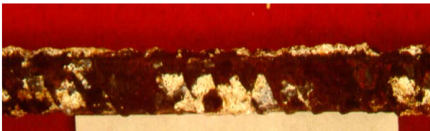
Figure 5.19. Corrosion Outside the Previous Exposed Region (Beam 30).
