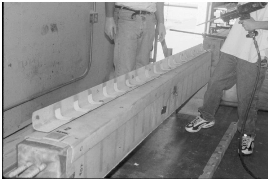
Figure 3.6. Installation of Angles.
