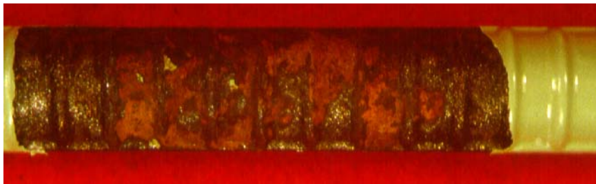
Figure 5.12. Rust Stains Underneath Coating on Epoxy Coated Bar (Beam 6).
