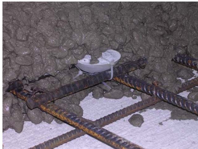
Figure 8-4 Placing of Concrete
