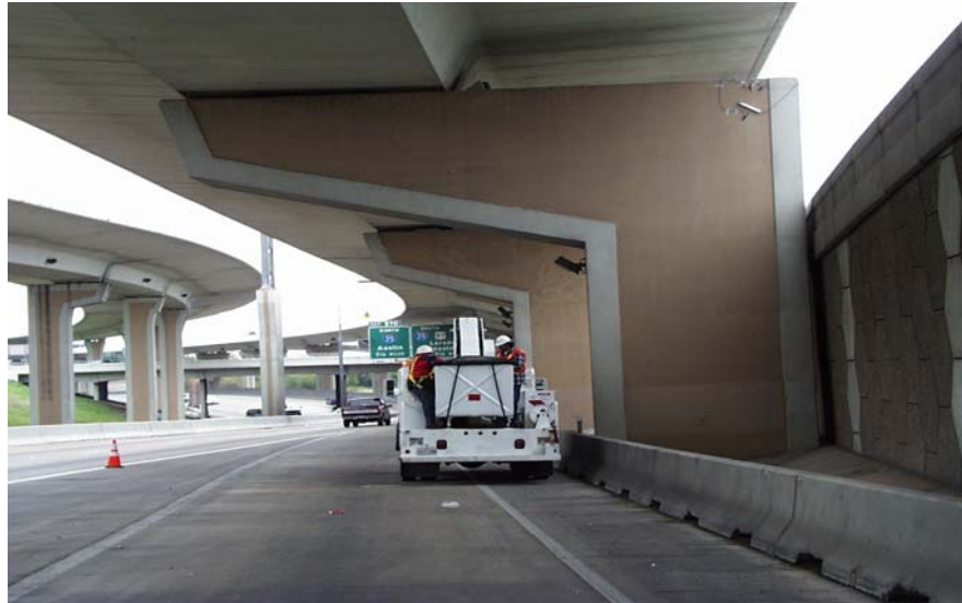
Figure 5.29 – Monitored Column in San Antonio, TX
