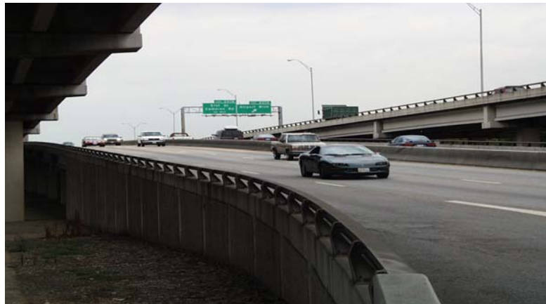
Figure 5.12 – I-35 Overpass U-Turn Lane near 41 st Street, Austin, TX
