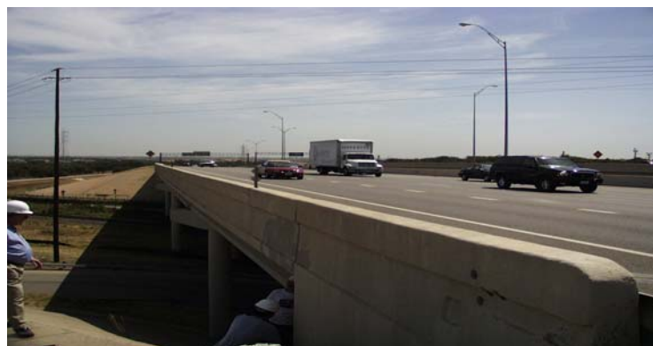
Figure 5.6 – Southbound Mopac Railroad Overpass between Braker and Burnet, Austic, Tx
