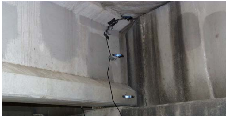
Figure 5.5 – Attached Sensor Location
