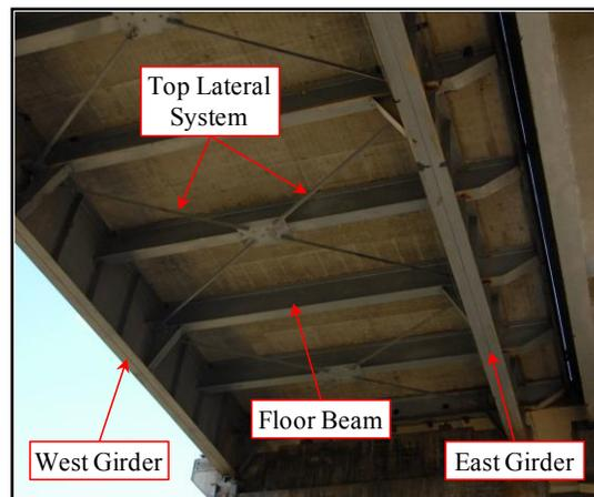
**Figure 3-9: Top lateral system of Bridge A**
