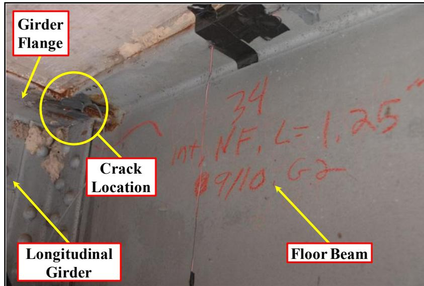
*Figure 3-11: Crack location*
