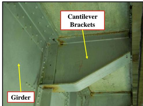
*Figure 3-2: Cantilever brackets*
