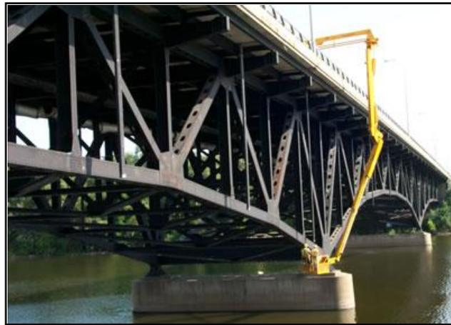
*Figure 1-1: Current inspection practices for fracture critical bridges*
