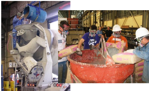
(c) Mix concrete
