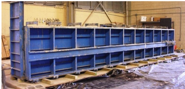
(b) Erect formwork, place cage inside
