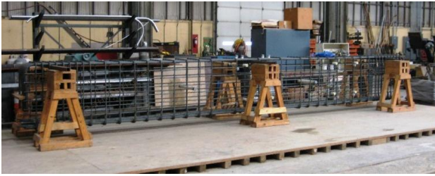
(a) Construct reinforcement cage
