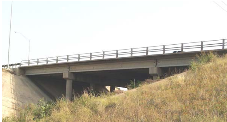
Figure 1.1: Typical AASHTO Girder Bridge
