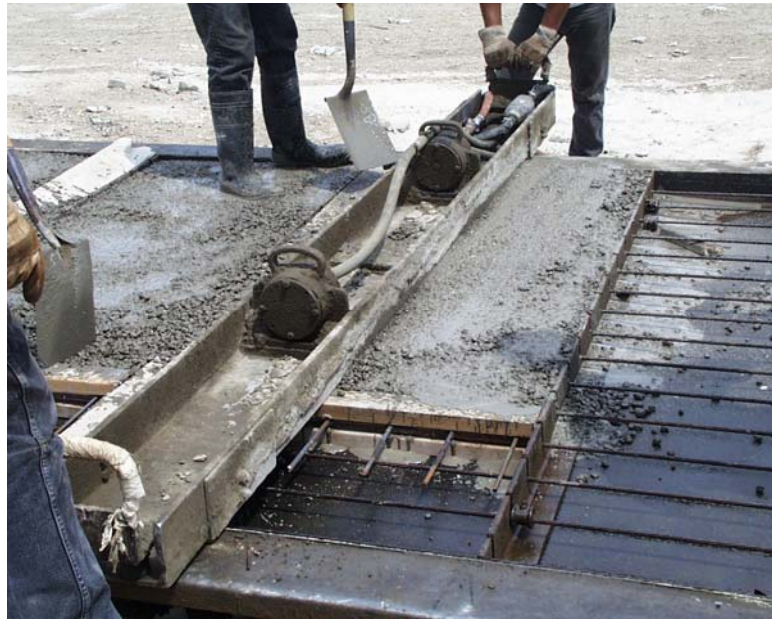
Figure 3.8: Lightweight Concrete Panel Casting
