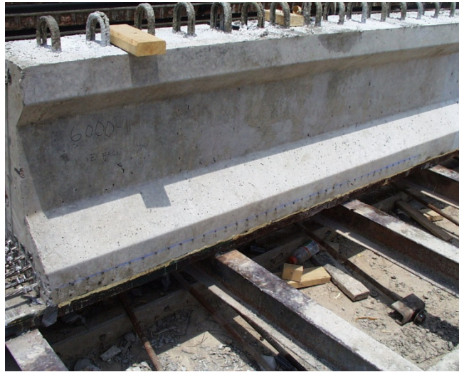
Figure 4.10 Finish of Girder Made with 6000 psi Mix Concrete
