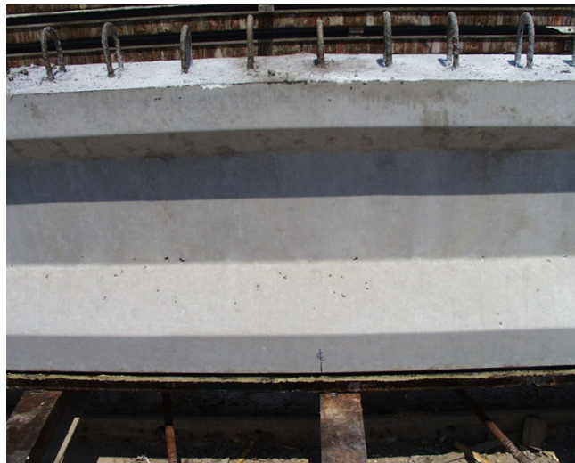
Figure 5.10 Finish of Girder with 8000 psi Concrete Mix
