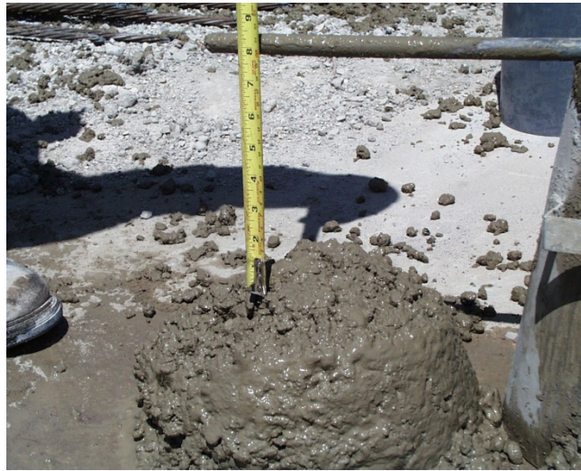
Figure 4.8 Slump of First Batch of 6000 psi Concrete
