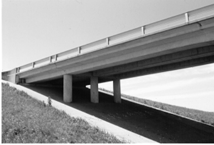
Figure 5.3 Individual columns used to support individual beams
