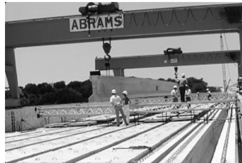
Figure 3.52b Placement of precast girders using straddle cranes
