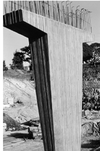
Figure 5.49 Vertical grooves give this wide pier a more slender appearance.
