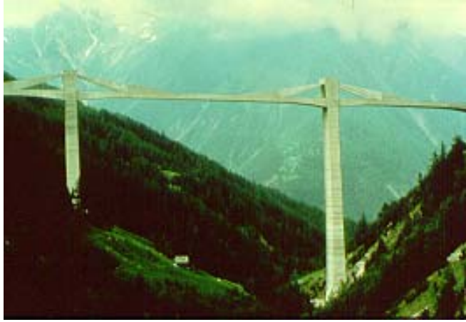
Figure 3.1 The Ganter Bridge, Switzerland
