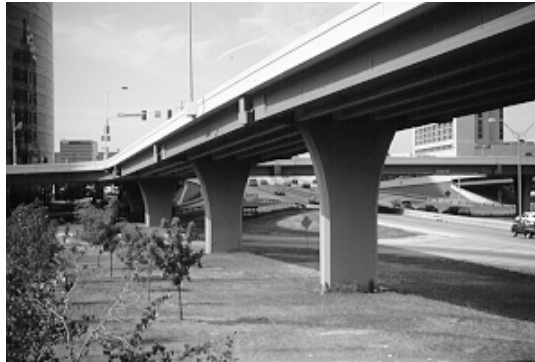
Bridges of similar superstructure and roadway width with a forest of columns (a) or a single elegant tapered column (b)
