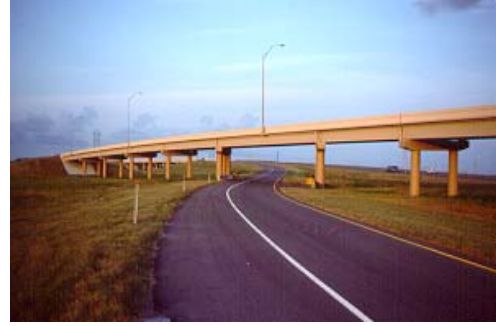
Figure 5.57 Concrete painted with an earthtone to integrate with the landscape.
