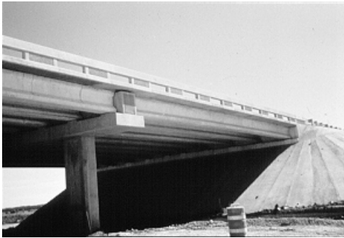
Figure 5.52 Similar formliner patterns used for the railing and the end of the bent cap
