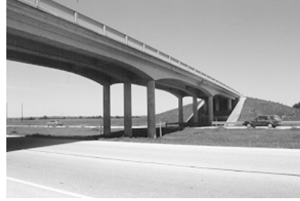
Figure 5.4 Individual columns supporting individual cast-in-place continuous beams
