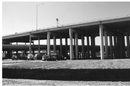
Figure 5.16 Cluttered multi-column bents create "forests" of columns
