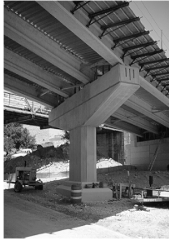
Figure 5.26 Attractive integration of the cap and column through simple column chamfers and cap tapers (a & b)
