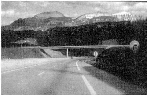
(b) A completed channel bridge
