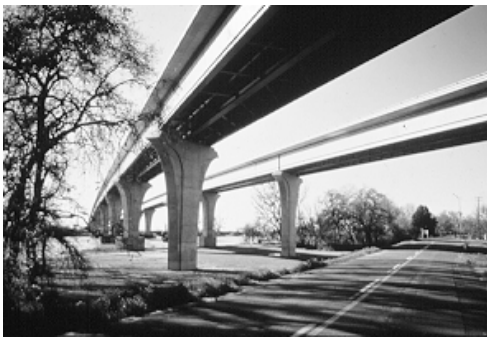
Figure 5.48 Vertical relief enhances the slenderness of this pier.
