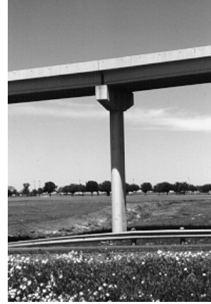
A rectangular column and prismatic cap (a) and a rounded column joining a prismatic cap (b).
