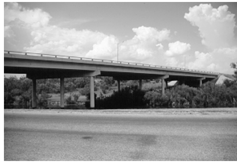
Figure 6.7 A precast prestressed concrete I girder bridge crossing the Concho River
