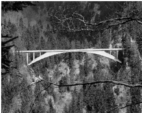
A vision of expressing the thinness possible with reinforced concrete in an arch form.
