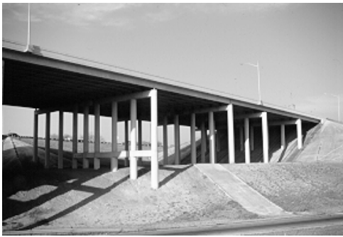
Figure 5.32 Cluttered multi-column bents (a) replaced with more open two-column frame bents (b)
