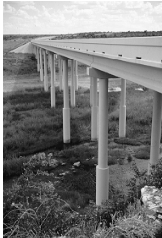
Bridges of similar superstructure and roadway width with a forest of columns (a) or a single elegant tapered column (b)
