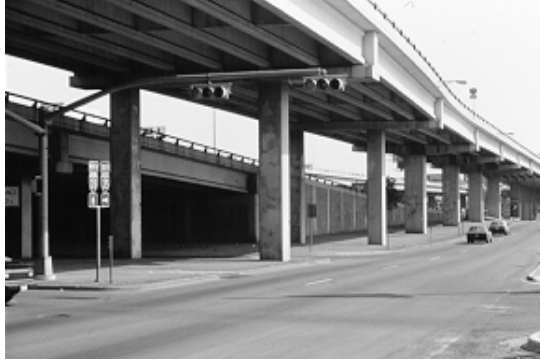
Figure 6.30 View of an I girder bridge from below
