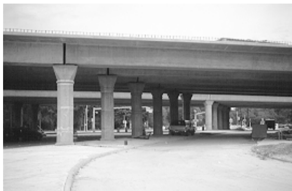
Figure 4.12 Precast piers for a grade separation in Houston, TX
