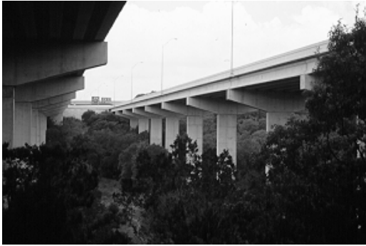
Figure 3.62 The even, repetitive single-column bents provide an attractive and well-balanced appearance.
