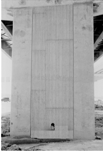
Figure 3.47 Use of internal drain pipes
