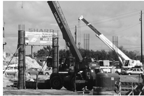
Figure 3.45 Repetitive cast-in-place columns requiring considerable on-site labor and space
