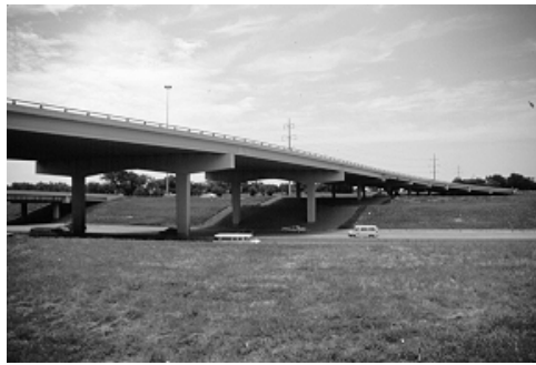
Figure 5.32 Cluttered multi-column bents (a) replaced with more open two-column frame bents (b)
