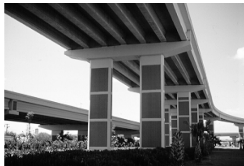
Figure 5.51 Horizontal accents give tall piers a stockier appearance.
