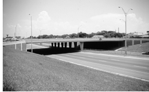
Figure 3.10 Attractive overall form and details of abutments and substructure
