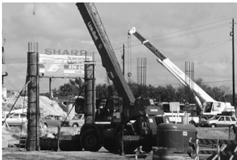
Figure 1.11 Extensive on-site equipment for cast-in-place multi-column bents.
