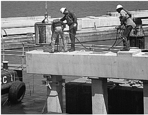
Figure 4.5 Precast pile caps for the Redfish Bay low water crossing
