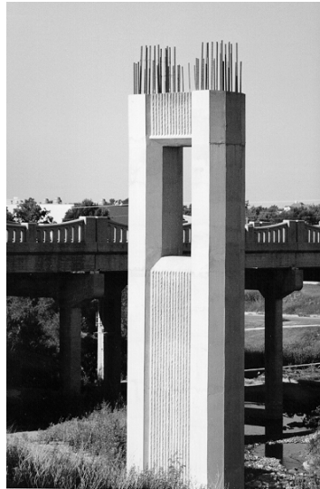
Figure 6.19 A windowed pier under construction for US 67
