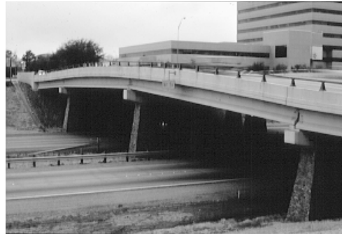
Figure 5.53 Concrete piers formed to appear like stone are foreign to the modern superstructure and urban location.
