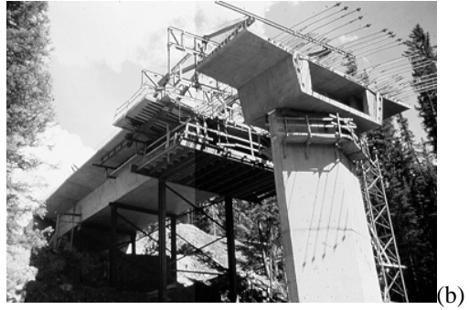
Figure 4.7 A schematic drawing (a) and the as-built view (b) of the precast concrete piers for Vail Pass in Colorado 30
