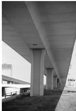
Figure 5.7 Individual columns supporting a single box girder bridge
