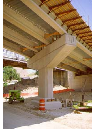
Figure 5.47 An attractive pier with a rubbed concrete finish
