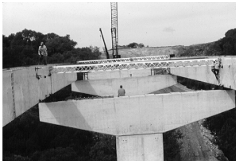
Figure 3.52a Steel girders positioned for straddle cranes
