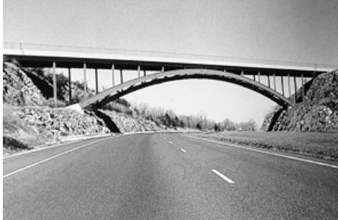
Figure 3.42 An arch bridge taking advantage of the natural abutments
