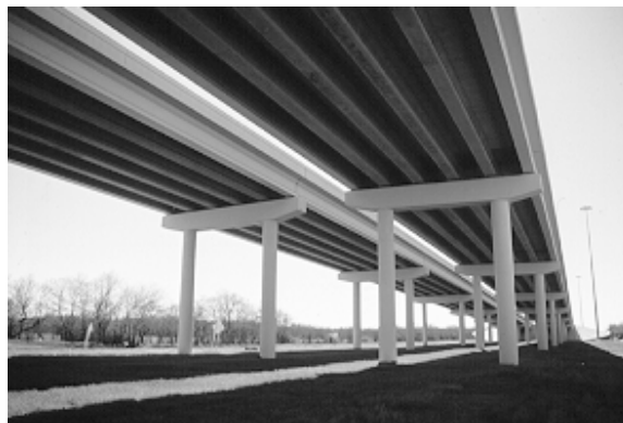
Figure 3.68b Splitting a wide bridge into two separate bridges allows more light to reach underneath
