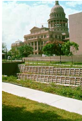
Figure 5.59 Low concrete retaining walls colored to match local building materials
