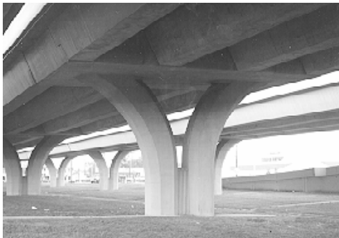
Figure 5.54 An attractively shaped pier showing off concrete's moldable quality
