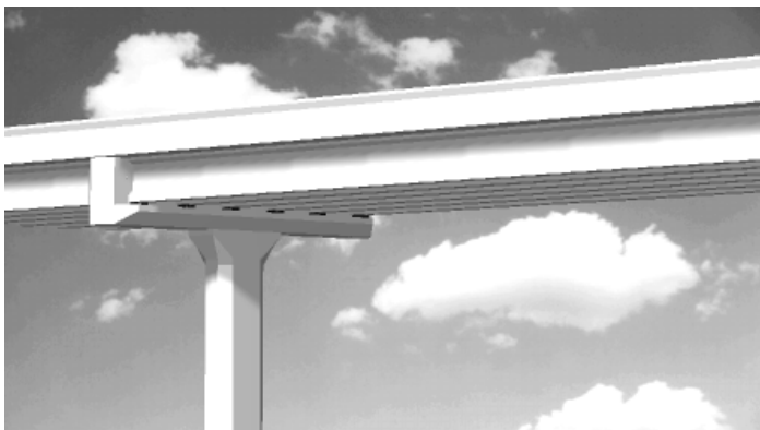
Figure 3.46 Precast concrete substructure systems can be efficiently fabricated and erected with attractive and durable results.
