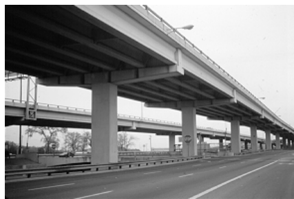
Partially integrated bent caps with rectangular columns and prismatic caps (a) or with round columns and prismatic caps (b)
