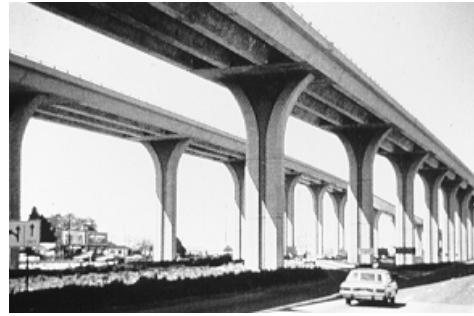
Accented joints give the appearance of a masonry structure (a). A smooth surface (b) shows off concrete's ability to perform its structural task in a flowing form.
