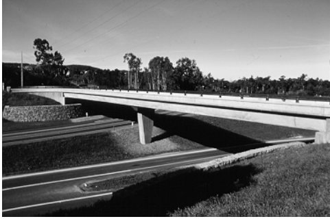
Figure 3.9 Attractive overall form and details of abutment, rail and substructure
