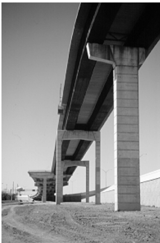
Figure 5.50 Horizontal grooves make concrete appear like masonry.
