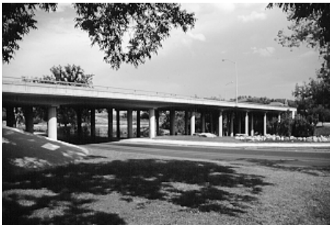
Figure 6.6 A cast in place slab bridge crossing the Concho River
