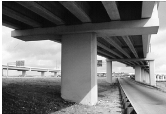
Figure 5.41 Small chamfers on a rectangular column
