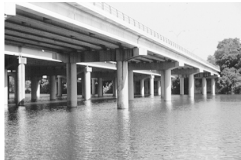
Figure 5.2 Typical cast-in-place substructure system in Texas
