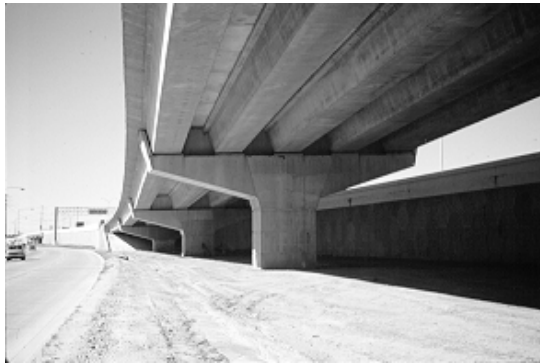
Figure 6.32 View of a U-beam bridge from below
