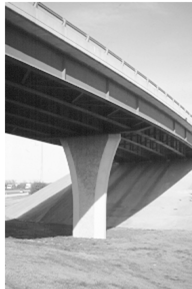
Figure 5.55 An elegantly tapered pier with exposed aggregate used to accent slenderness
