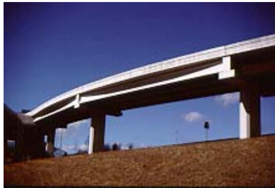
Figure 6.31 Scalloped shadows on curved bridges made up of straight girders
