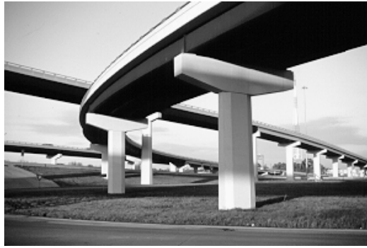
Figure 5.26 Attractive integration of the cap and column through simple column chamfers and cap tapers (a & b)
