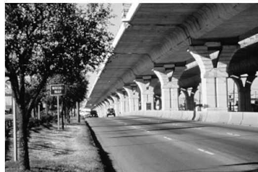
Segmental construction allowed for rapid construction and improved surface finish
