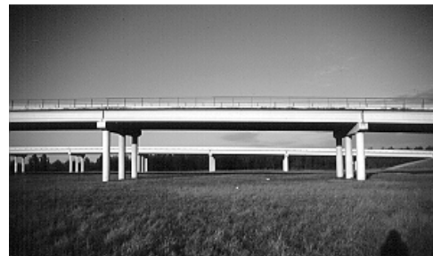
The development of standard precast prestressed I-girders has economically increased span lengths and reduced the number of required substructure units
