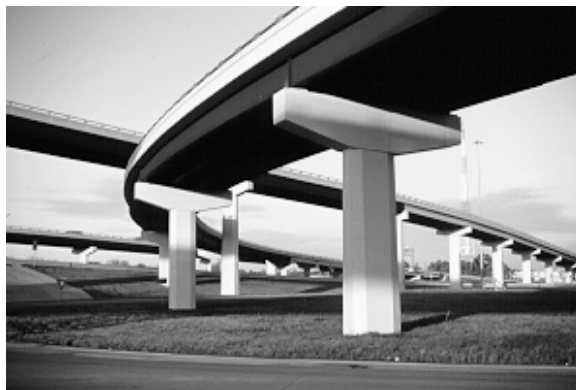
Figure 5.42 A large chamfer makes these rectangular columns appear slender
