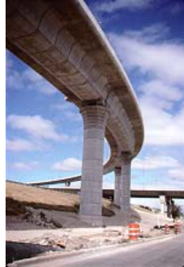
Figure 4.11 Precast segmental piers at US 183 in Austin, TX
