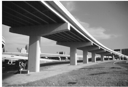
Figure 5.13 Hammerhead bents entirely underneath the superstructure
