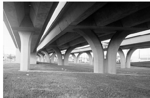
Figure 1.12 An attractive cast-in-place substructure.
