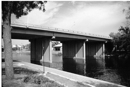
Figure 5.9a Wall substructure units for a water crossing
