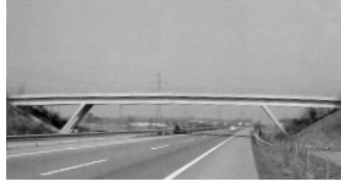
Figure 3.43 Angled strut piers decrease the clear span and superstructure depth while increasing clearance for traffic passing through (photo, Reference 23)
