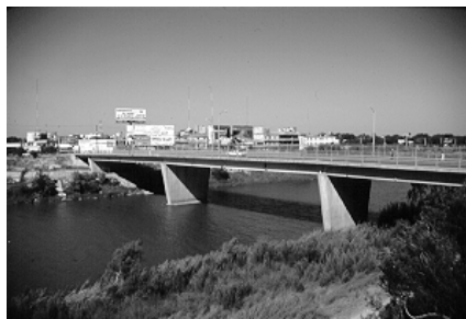
Two single tapered walls with long spans (a) increase visibility through the river crossing whereas multi-column bents with shorter spans (b) block visibility
