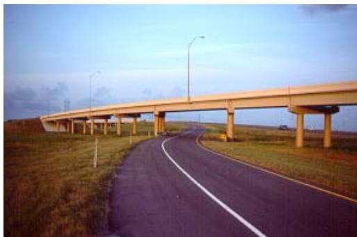
Figure 3.64 An attractive coat of paint does little to improve this awkward skewed layout
