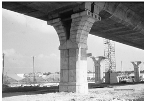
Figure 3.53 US 183 in Austin Texas during construction
