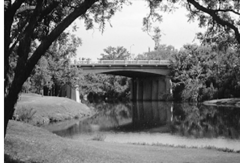
Figure 6.5 One of the older bridges crossing the Concho River in San Angelo
