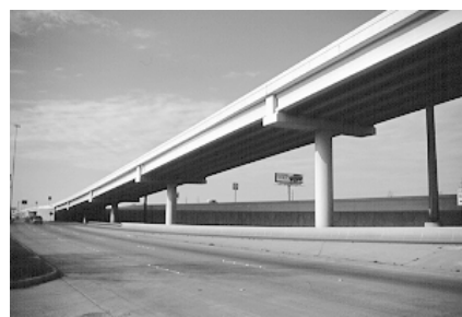
Partially integrated bent caps with rectangular columns and prismatic caps (a) or with round columns and prismatic caps (b)
