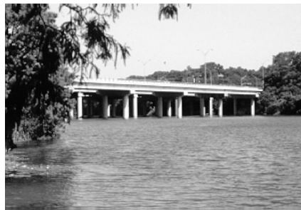
Two single tapered walls with long spans (a) increase visibility through the river crossing whereas multi-column bents with shorter spans (b) block visibility
