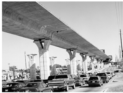
Accented joints give the appearance of a masonry structure (a). A smooth surface (b) shows off concrete's ability to perform its structural task in a flowing form.
