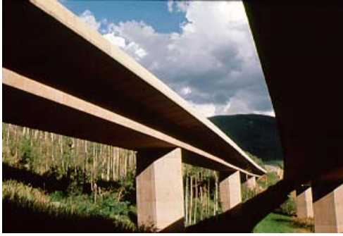
Figure 5.56 The concrete for these piers was stained to blend with the local rock coloring.
