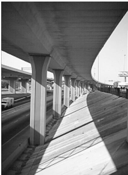
Segmental construction provided attractive and rapid construction for the highly visible and congested urban site
