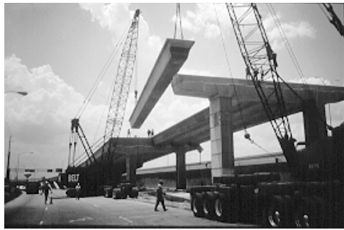
Figure 6.27a Two cranes are required to place precast concrete girders
