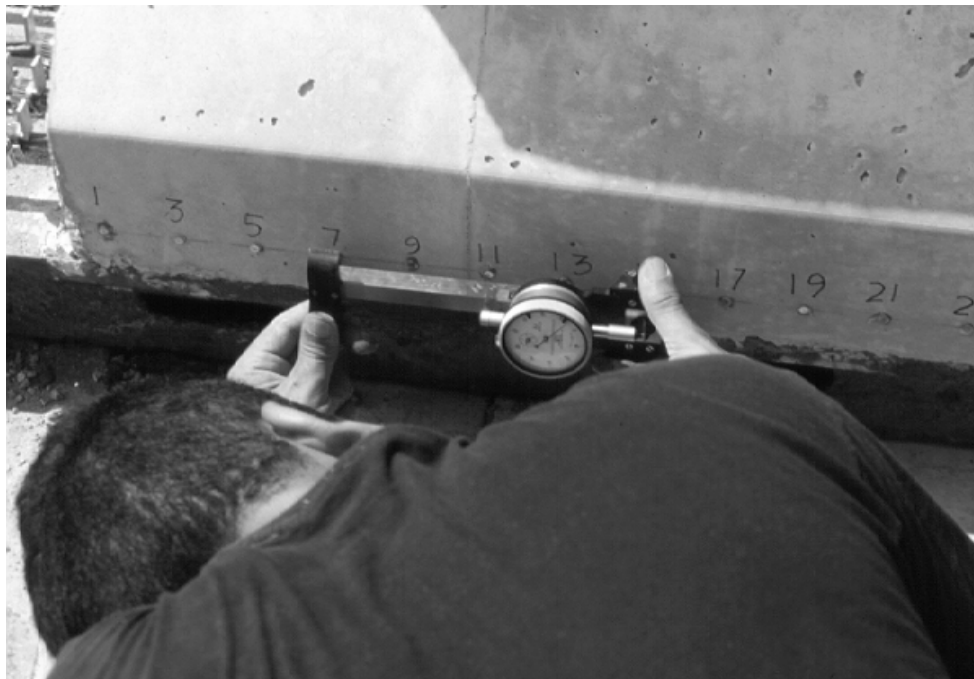
Figure 5.3: Performing a Measurement with DEMEC Gauge
