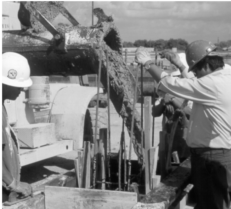
Figure 4.3: Casting Pull-out Test Block
