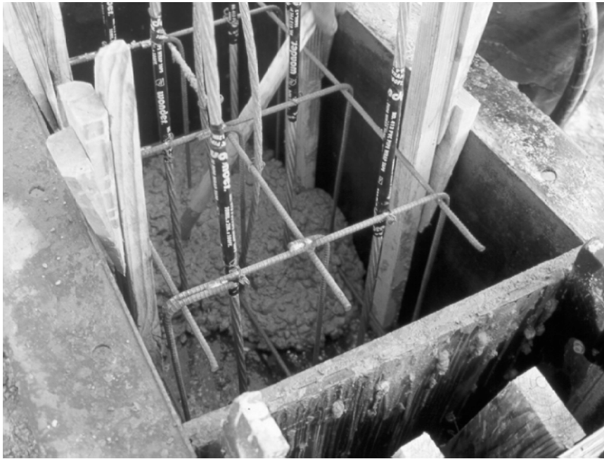
Figure 4.2: Pull-out Test Block at Onset of Casting
