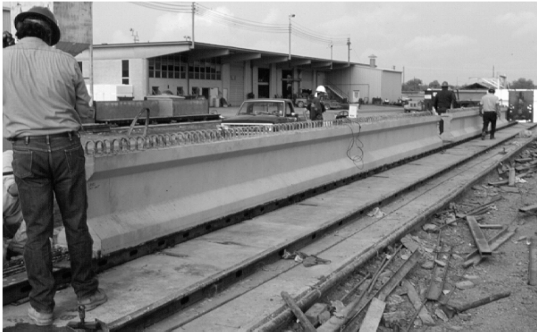
Figure 5.1: Pair of Beam Specimens after Side Form Removal
