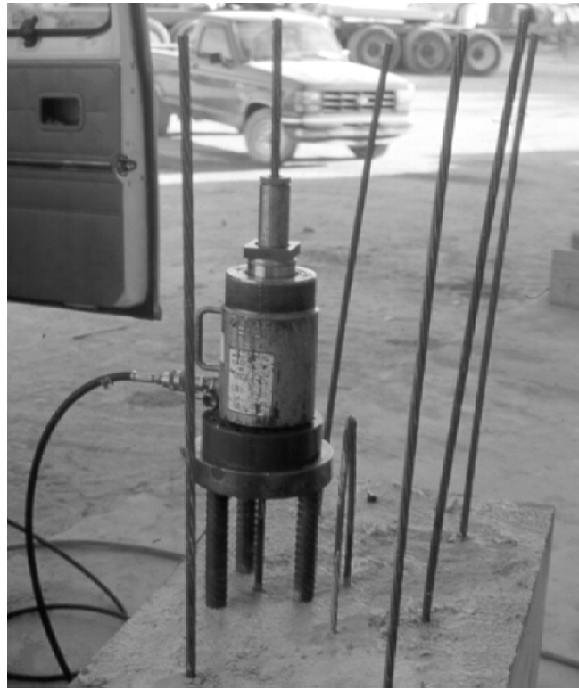
Figure 4.5: Pull-out Test in Progress
