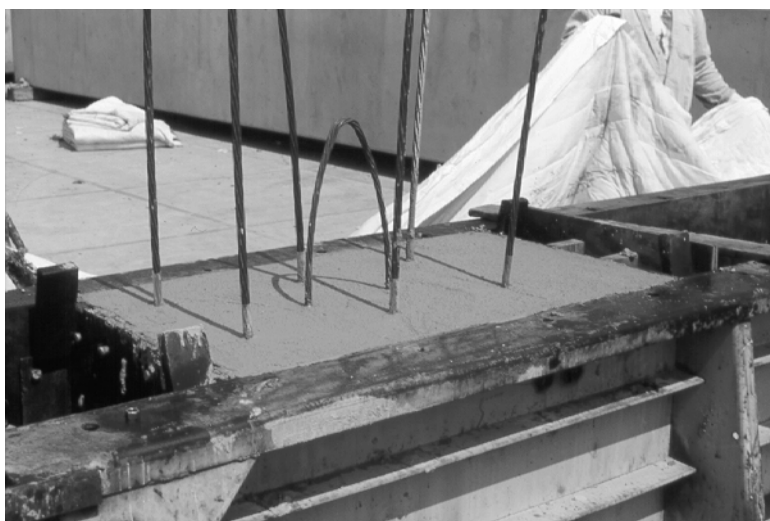
Figure 4.4: Finished Pull-Out Test Block
