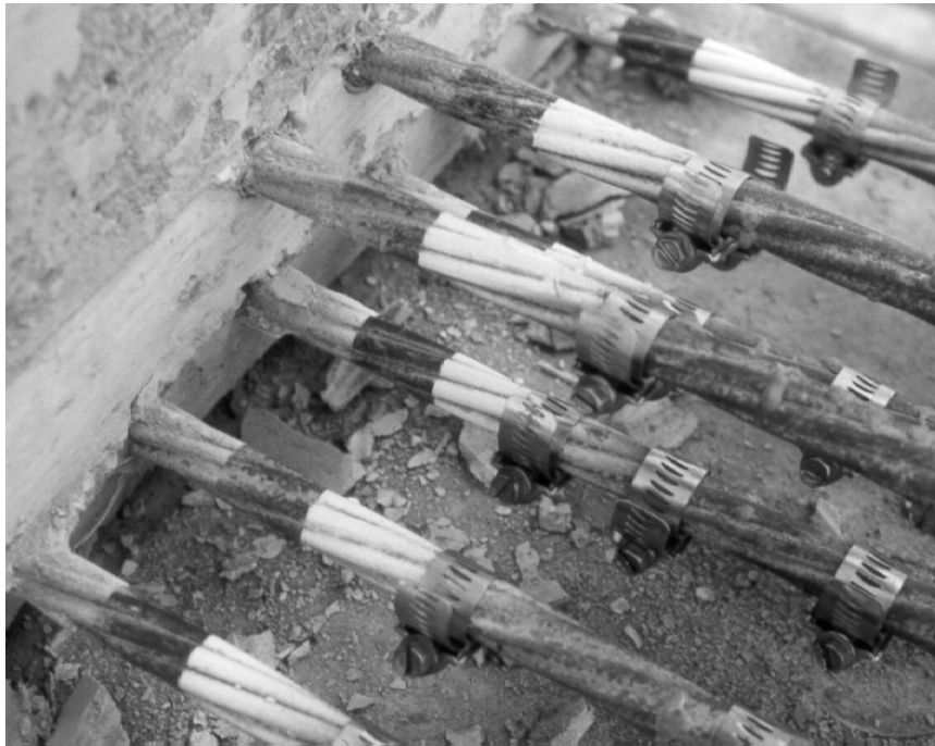
Figure 6.3: Strands Painted to Provide References for Draw-In Measurements
