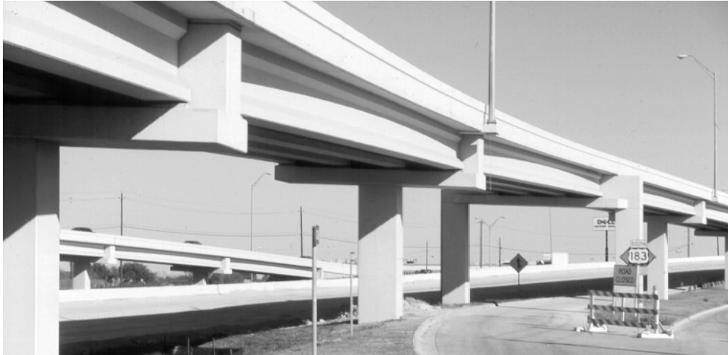
Figure 1.1: Highway Bridge Featuring Precast, Pretensioned I-Beam Superstructure
