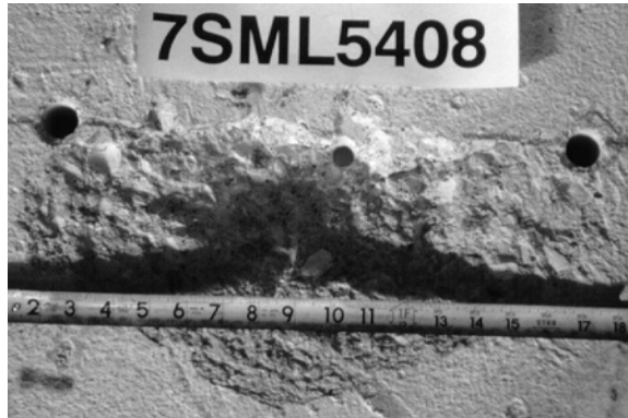
Figure 5.2 Typical Half-Cone Breakout of UC1 in 3/8-inch (10-mm) Diameter in Cracked Concrete
