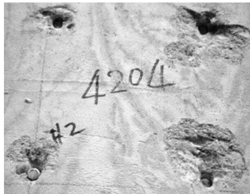
Figure 6.27 Concrete Spalling in Multiple-Anchor Connection with EAII Anchor in Dynamic Cyclic Loading
