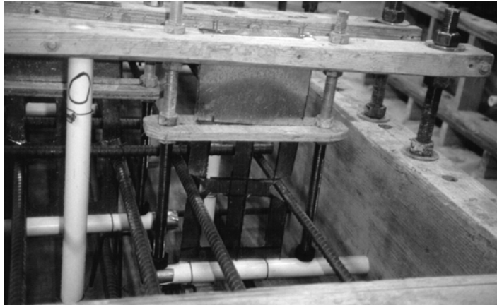
Figure 4.9 Cast-in-Place Anchors and the Steel Sheet in Between before Casting
