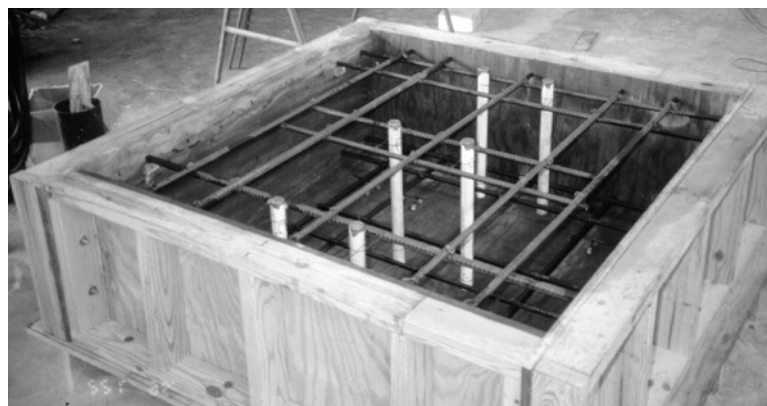
Figure 4.3 Formwork of Specimens for Task 4 Tests
