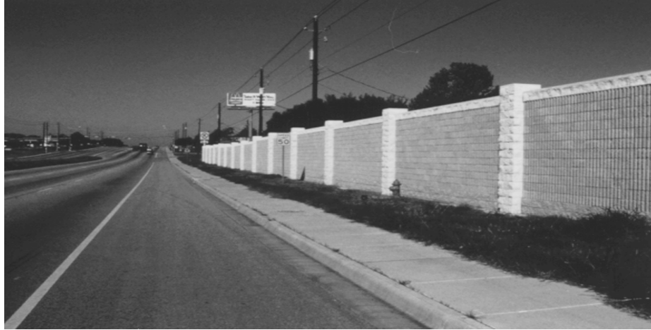
Figure A1.6 Constructed-in-place post-and-panel system (Austin District)
