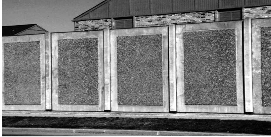
Figure A1.2 Example of prefabricated, separate post-and-panel system (Houston District)
