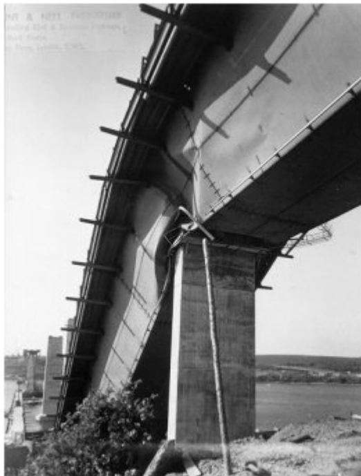
Figure 1.3 Failure of Milford Haven bridge in June 1970 (Flint, 2001)
