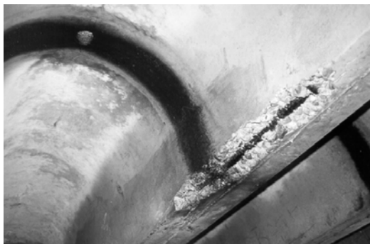
(a) Atmospheric Zone - Girder
