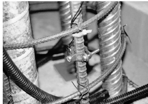
Ground Clamp to Attach Ground Wire
