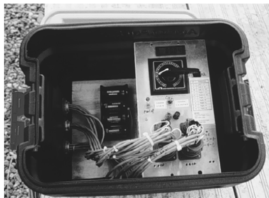
Figure 4.21 - Switching Box and Voltmeter for Column Half-Cell Potential Readings
