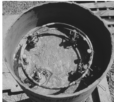
Top of Column Prior to Capping
