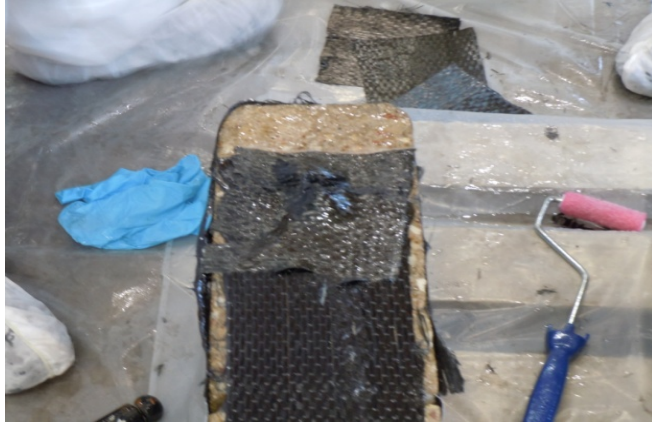
Figure 3-20 Applying the first patch
