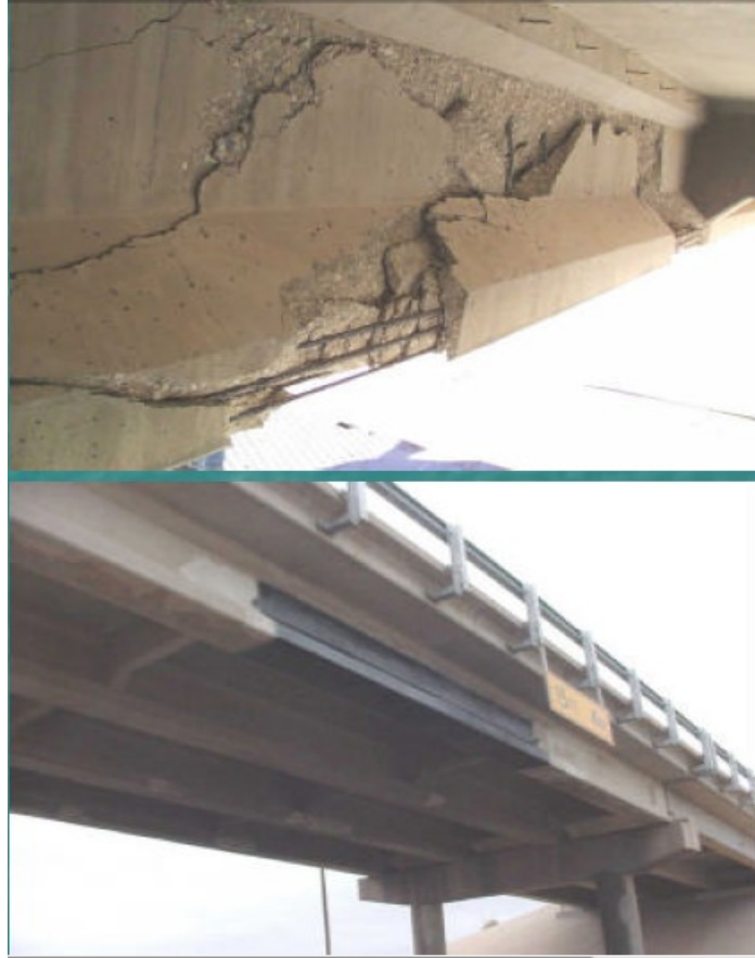
Figure 2-6 Application of CFRP material to repair IH 20 Bridge (D.Y. Yang, 2003)
