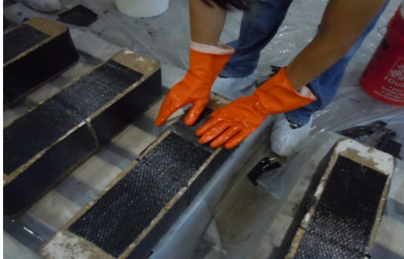
Figure 3-23 Applying the second patch
