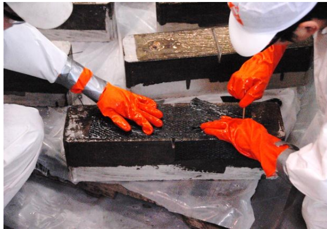
Figure 3-21 Inserting CFRP anchor
