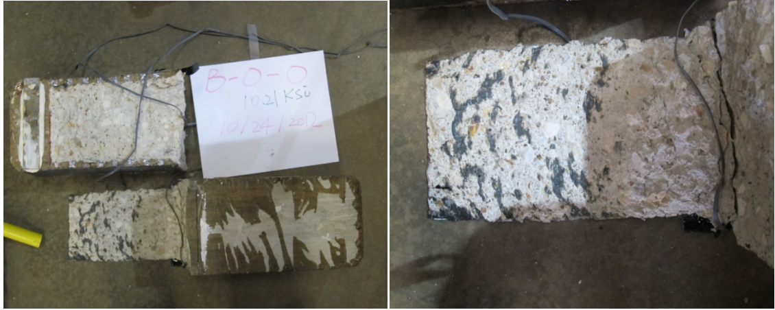
(a) Debonding failure
