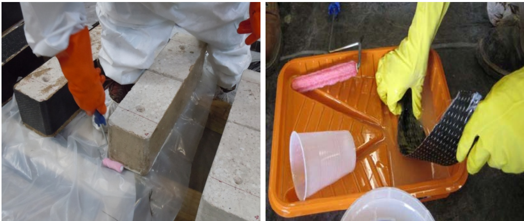
Figure 3-16 Saturating epoxy on concrete (left) and CFRP strip (right)
