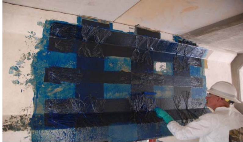
Figure 2-5 CFRP strengthening application
