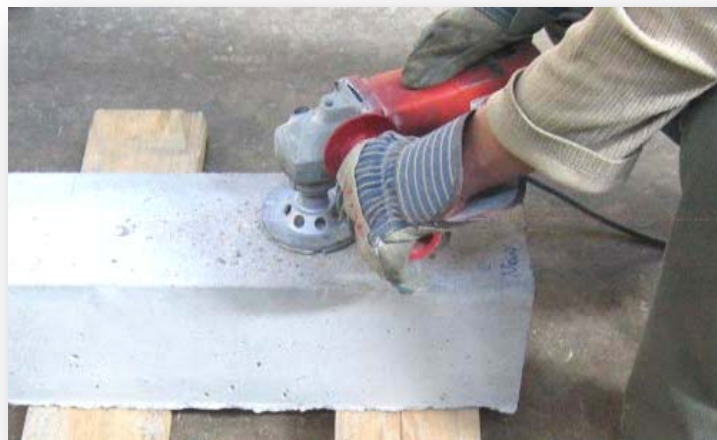
(a) Grinding concrete surface
