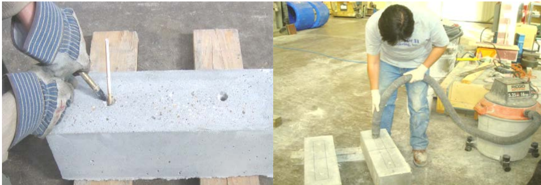
(d) Cleaning holes with compressed air or vacuum cleaner
