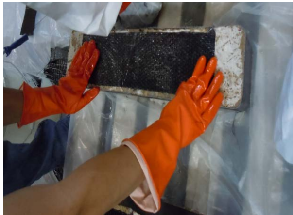
Figure 3-19 Applying CFRP strips
