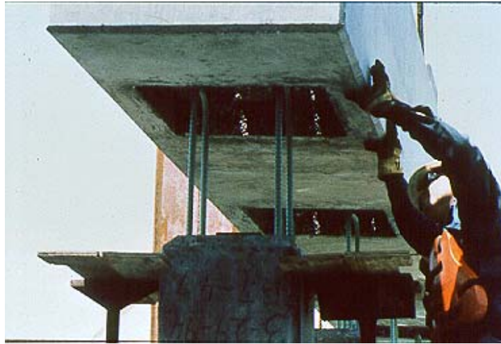
Figure 2.5: Erection of Red Fish Bay Precast Rectangular Bent Caps
