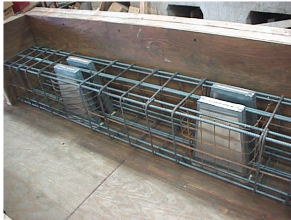
Figure 4.15: DLGP Confinement in Place
