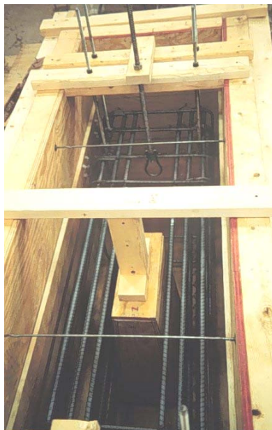
Figure 4.8: Completed Cage Ready for Casting
