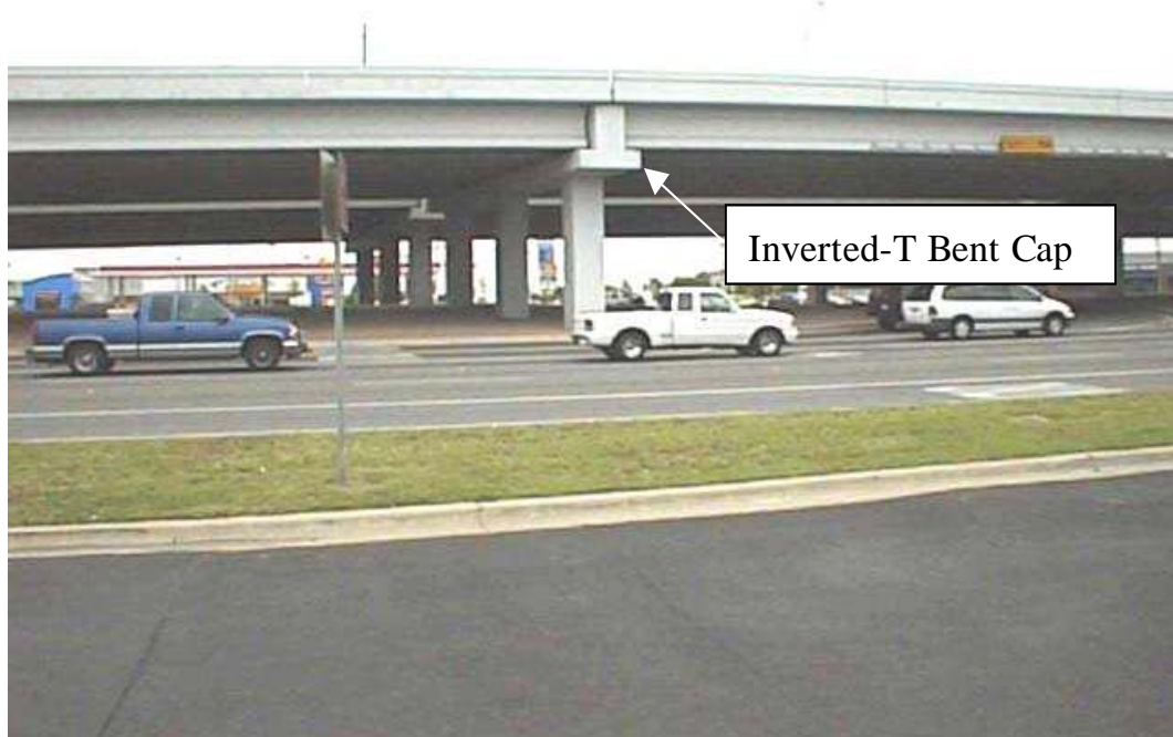
Figure 1.2: Typical Inverted-T Bent Cap
