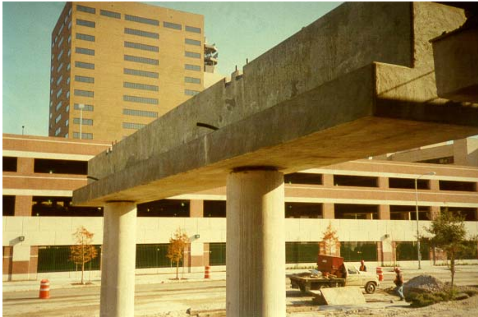
Figure 2.3: Precast Bent Cap Resting on Shims Prior to Grouting
