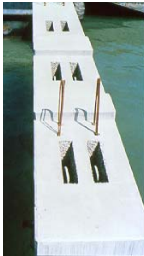
Figure 2.4: Grout Pockets
