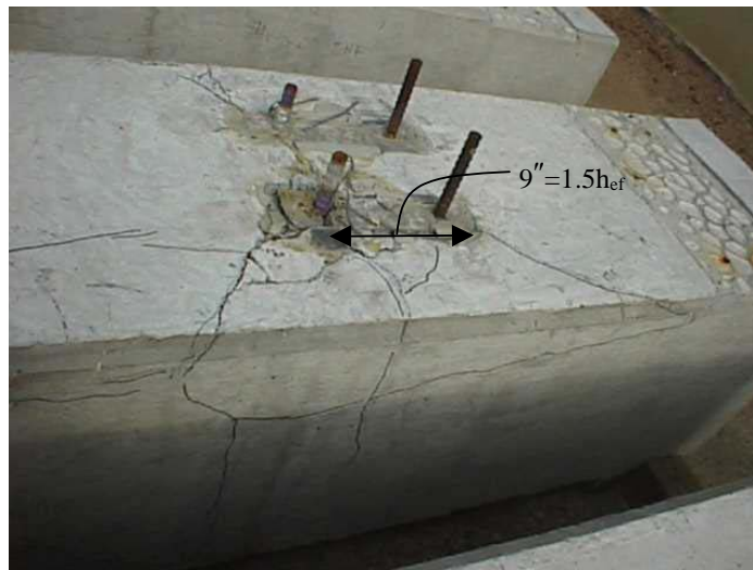
Figure 6.2: Failed Transverse Moment Specimen (DL01)
