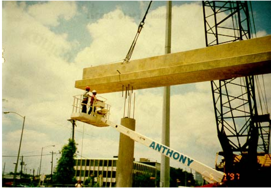
Figure 2.2: Erection of Pierce Street Elevated Precast Inverted-T Bent Cap
