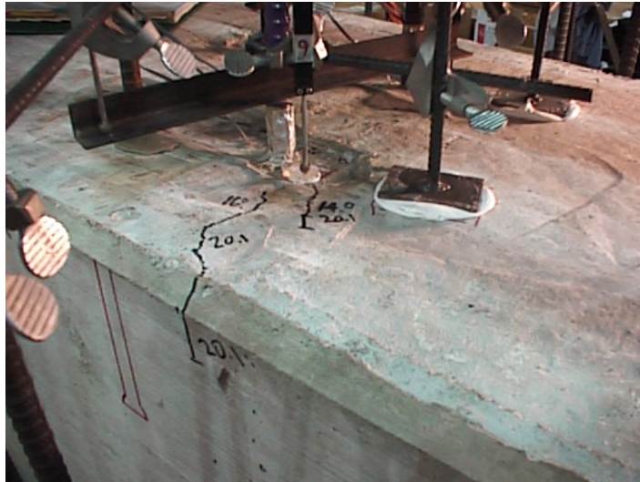
Figure 6.1: Splitting and Corner Cracks in DL01
