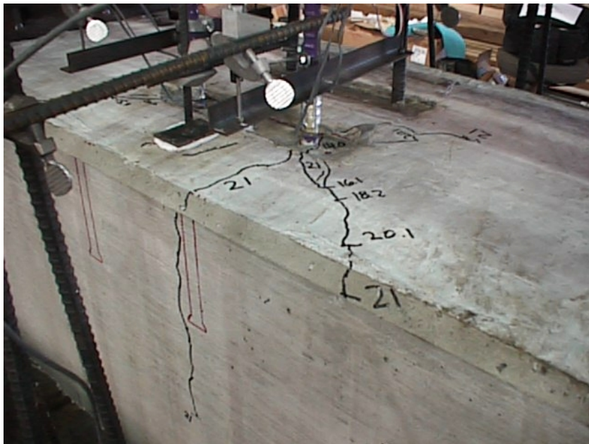
Figure 6.4: DL02 Cracking Near Failure
