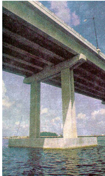
Figure 2.6: Edison Bridge Precast Bent
