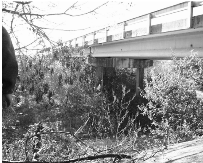
Figure 2.8 Willis Creek Bridge
