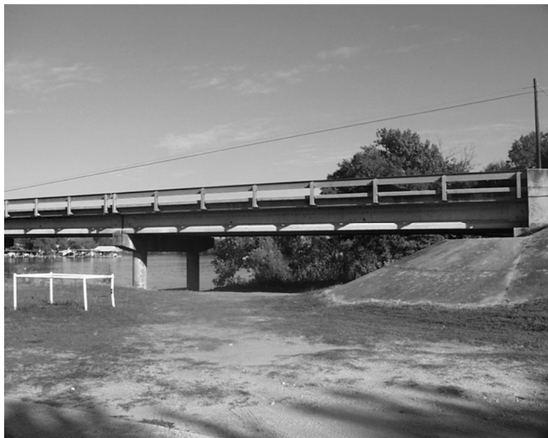
Figure 2.4 Lake LBJ Bridge
