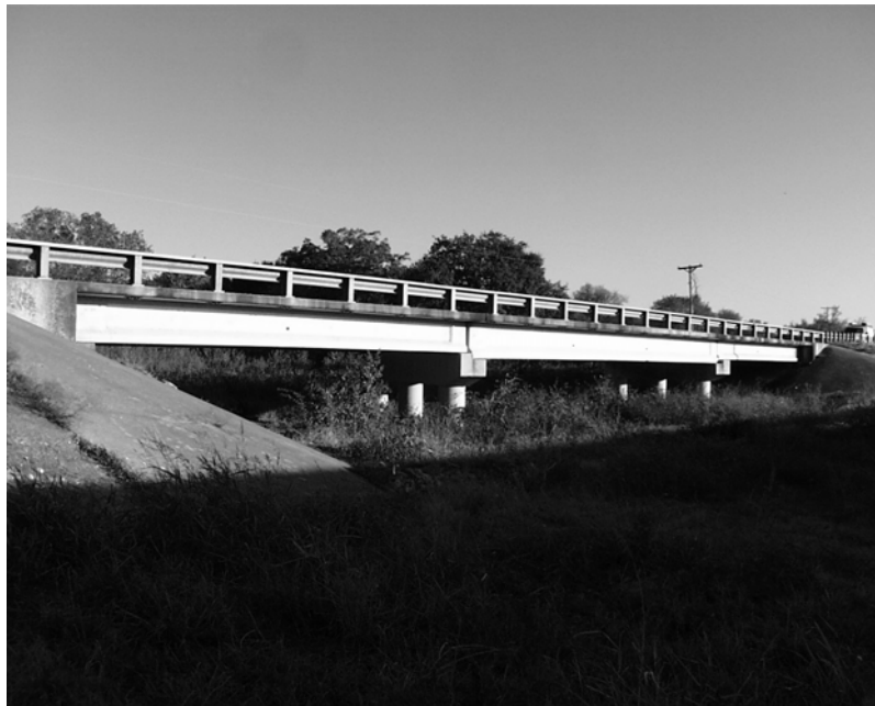
Figure 2.2 Chandler Creek Bridge
