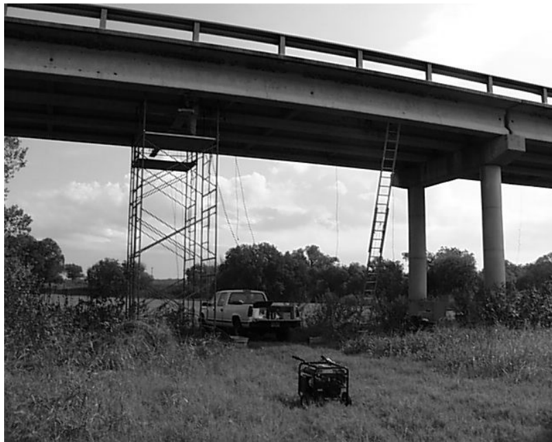
Figure 2.6 Lampasas River Bridge
