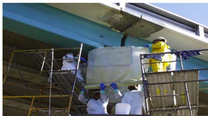
Figure 4.7 Application of Fibrwrap ® to endcap on Structure #2.
