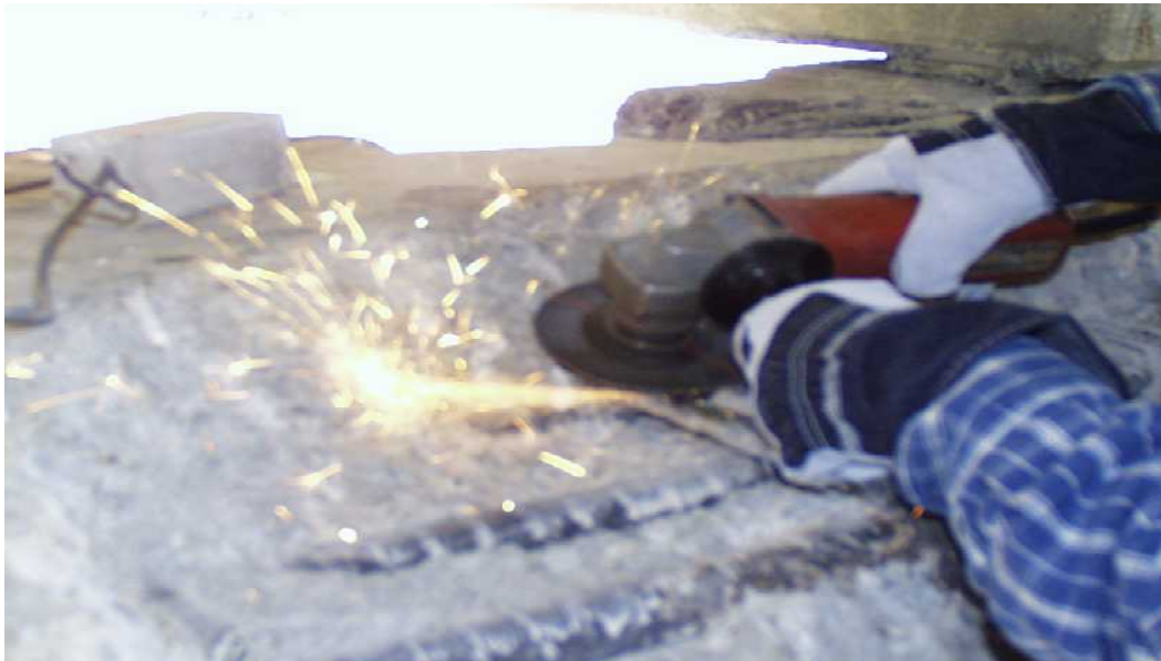
Figure 5.8 Grinding of the reinforcement to prepare for soldering.
