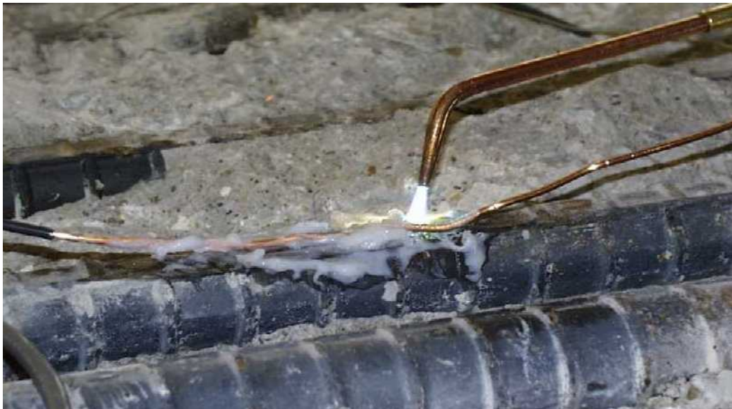
Figure 5.10 Application of flame to the copper-steel interface.
