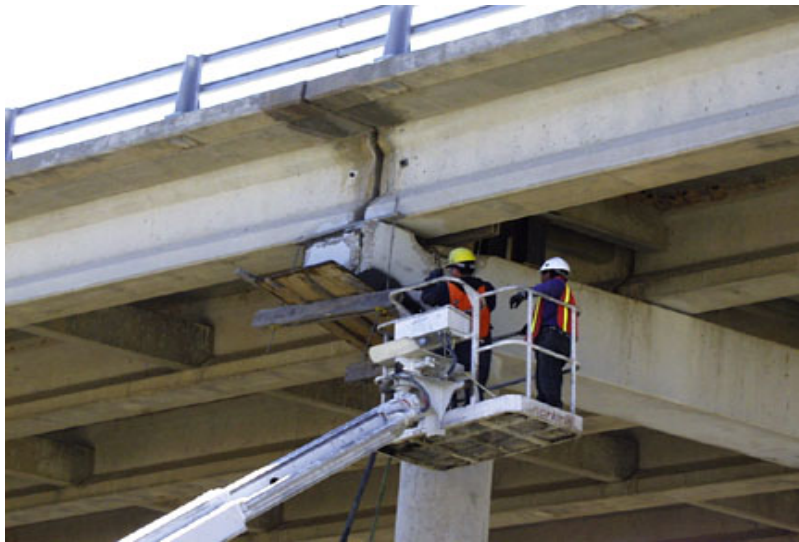
Figure 4.4 Application of Shotpatch ® 21F to Structure #3.
