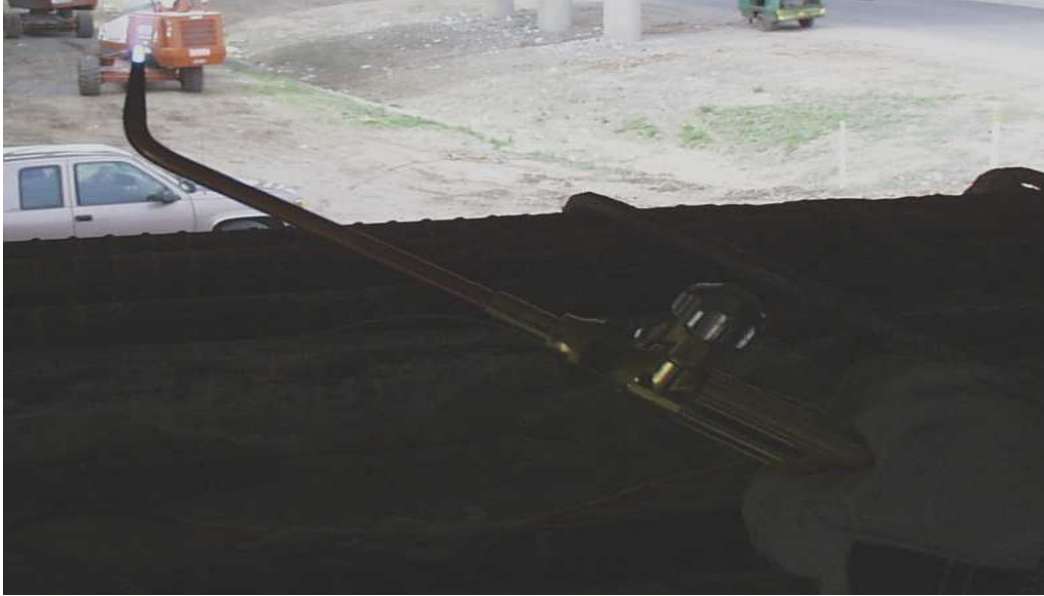
Figure 5.9 Torch flame for solder application.
