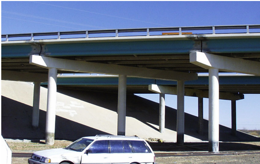
Figure 1.1 Structure wrapped with FRP.
