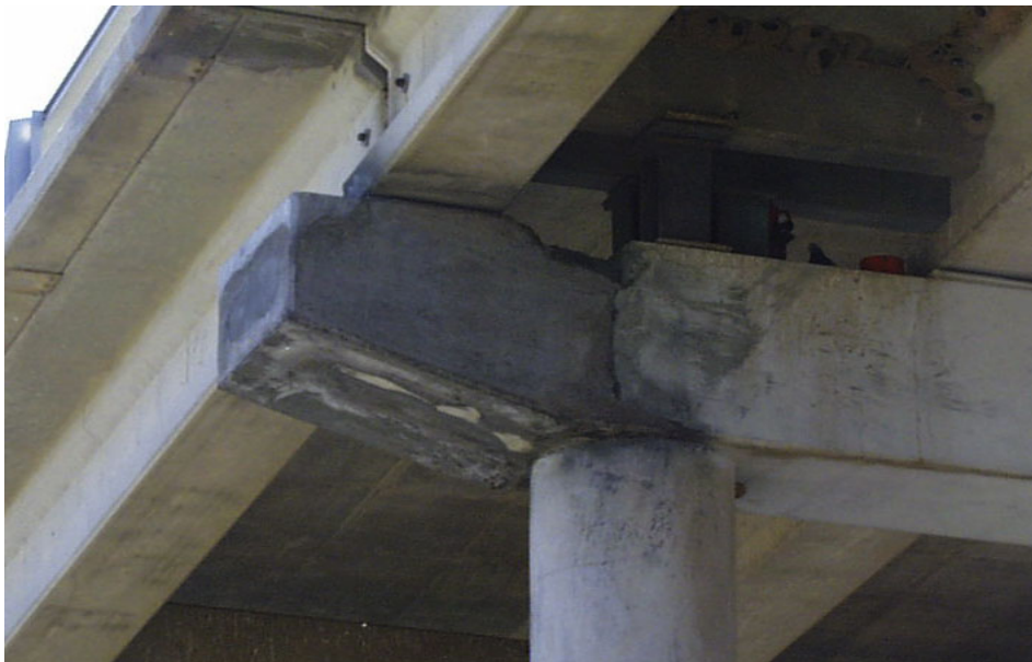
Figure 4.5 Endcap repair material on Structure #3.
