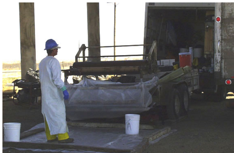
Figure 4.6 Saturation machine used by Delta Structural Technology, Inc.
