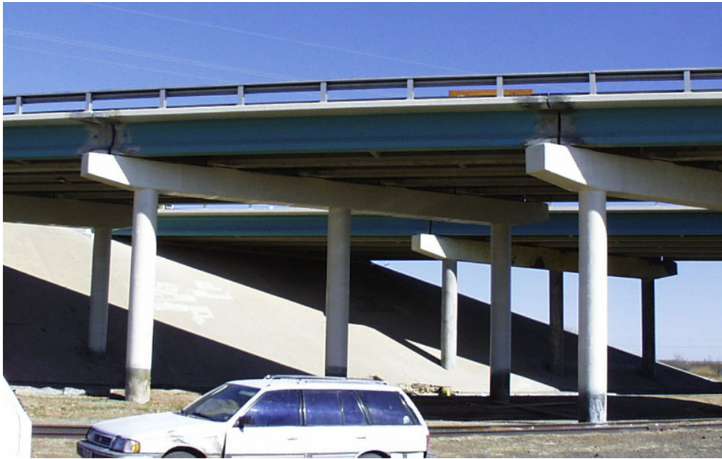
Figure 1.1 Structure wrapped with FRP.
