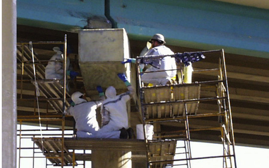
Figure 4.8 Removal of air pockets beneath a layer of Fibrwrap ® .
