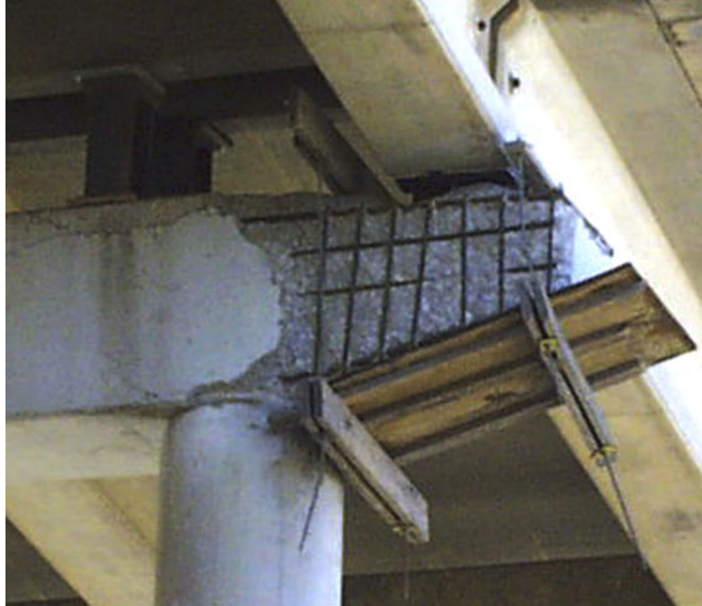
Figure 4.3 Endcap prepared for application of repair material on Structure #3.
