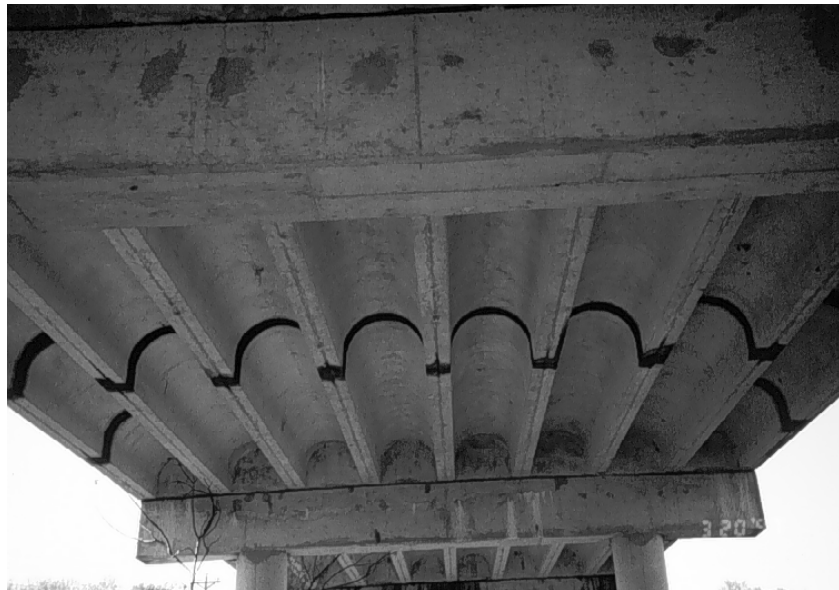
Figure 3.2 Instrumented Span Viewed from Below
