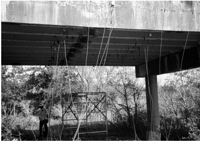
Figure 3.15 Cables Suspended from Bottom of Bridge
