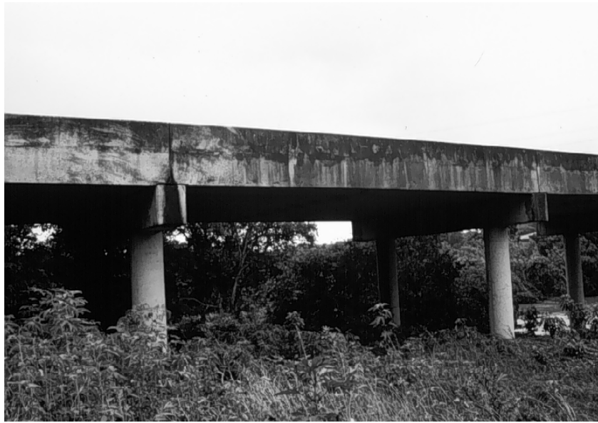
Figure 3.1 Instrumented Span Viewed from the South
