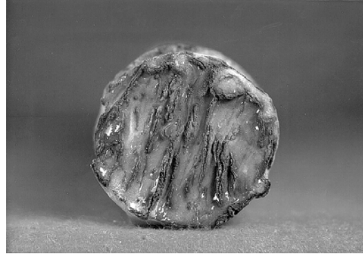
(b): Corrosion of patched end (torch-cut).
