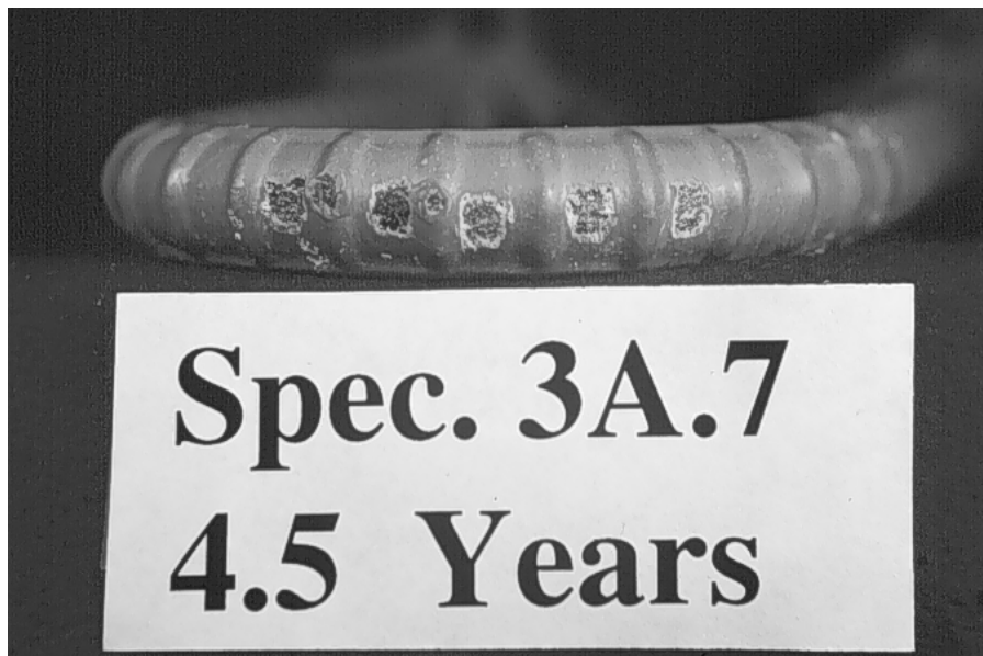
Fig. 8.26: Clean, uncorroded damaged areas after 4.5 years of exposure.
