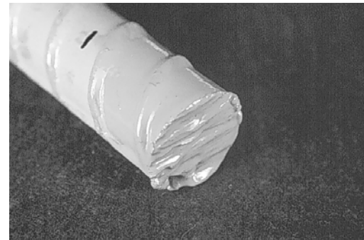
(b): Patched bar end (torch-cut).
