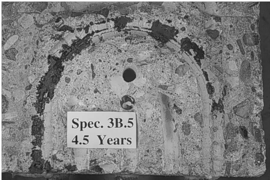
(b) Concrete below the bar.
