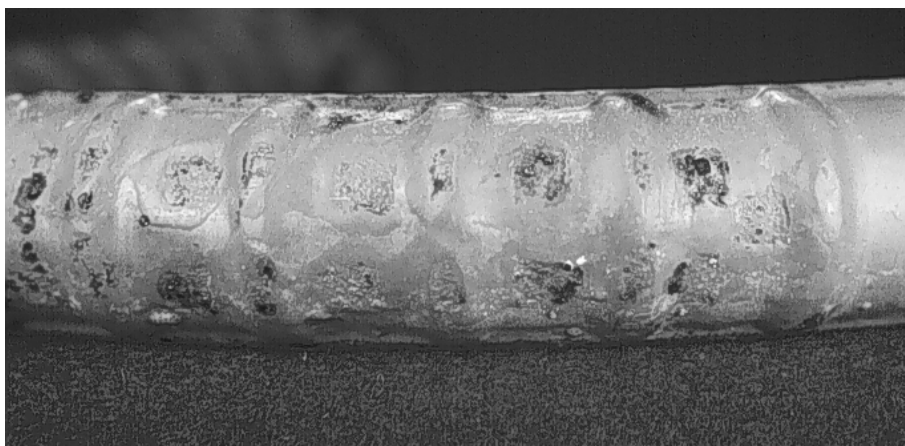
Fig. 8.29: Corrosion of patched areas at outside bend on bar 3B.4.
