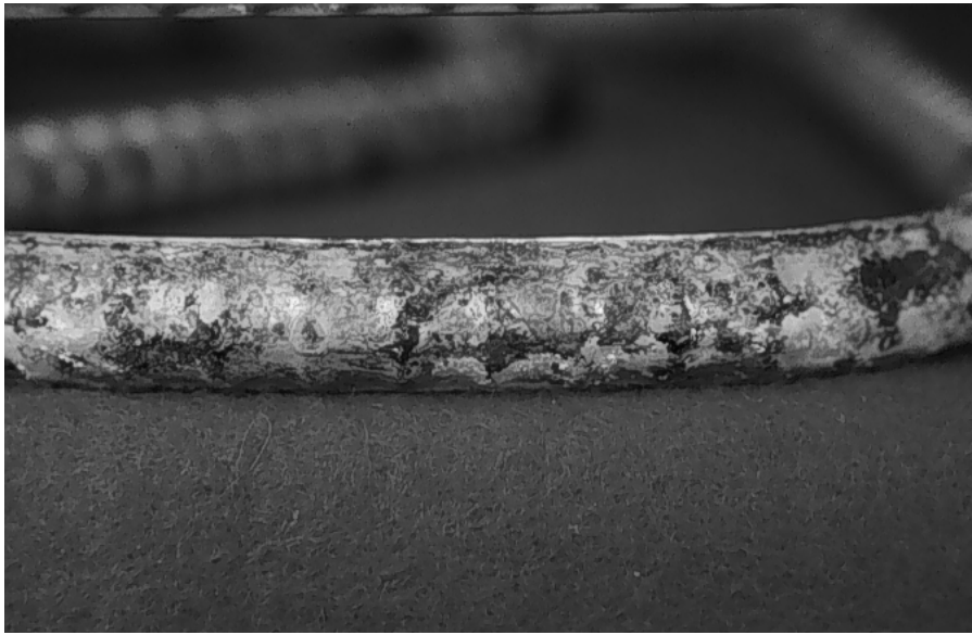
Fig. 9.59: Rust staining on a stirrup leg near the front beam surface (beam B32).
