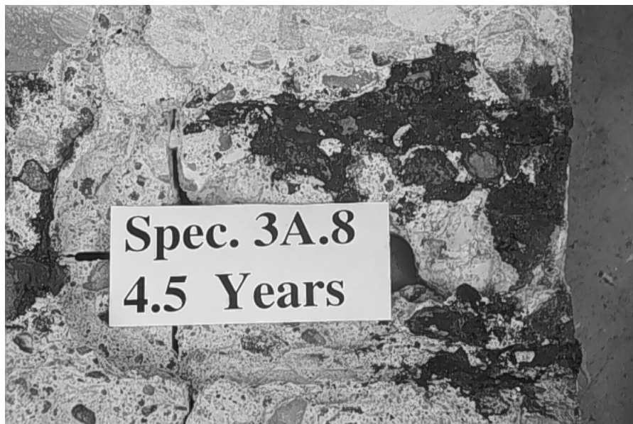
Fig. 8.41: Rust staining on surrounding concrete under uncoated bar 3A.8.
