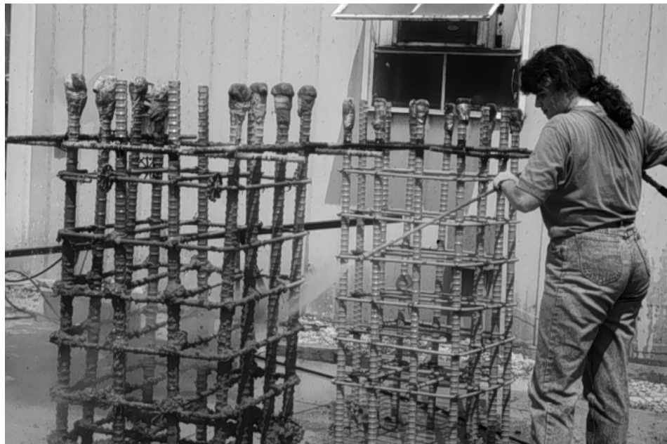
Fig. 7.4: Washing column cages after vibration.
