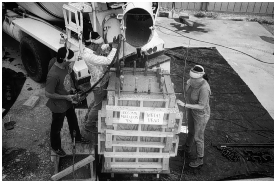
Fig. 7.2: Consolidating column specimen.
