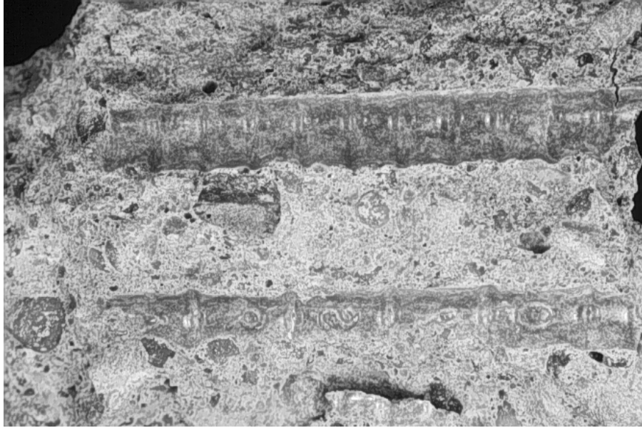
(a) Above epoxy-coated bars as in casting position.
