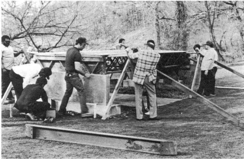
Figure 2.3. Virginia Footbridge. Set in Place (McCormick, 1986).
