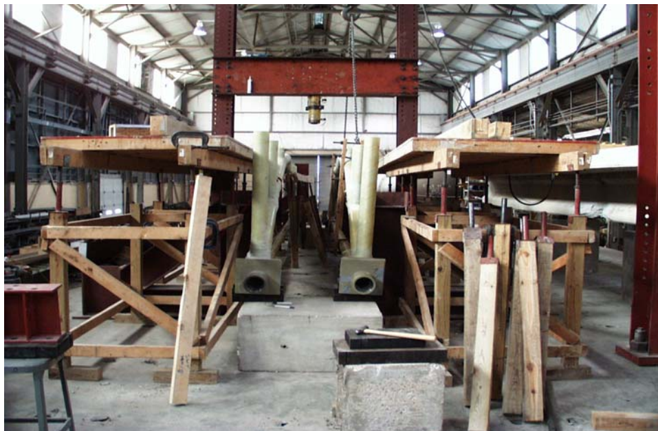
Figure 9.17. Arches in Place Prior to Completing Formwork for RC Deck.
