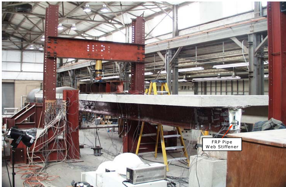
Figure 8.6. FRP Pipe Web Stiffener at South End.
