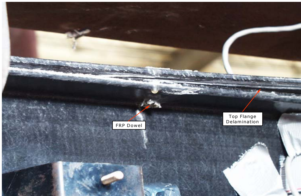
Figure 7.16. Specimen SW2 Top Flange Delamination.
