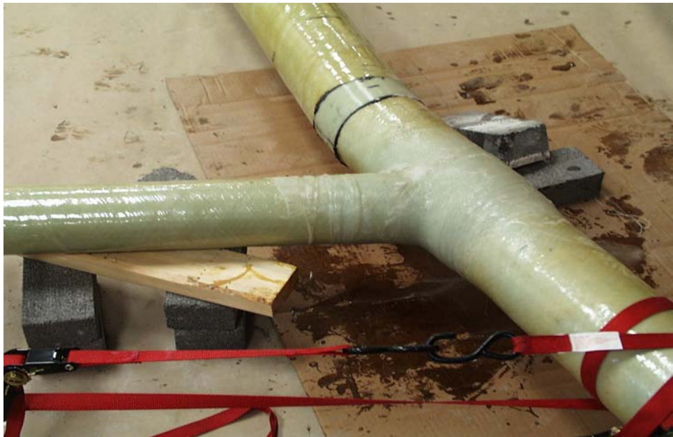
Figure 9.10 Finished Connection Type 2.
