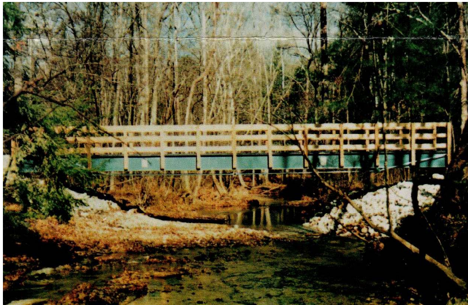
Figure 2.9. Daniel Boone National Park Footbridge (SPI, 1996).
