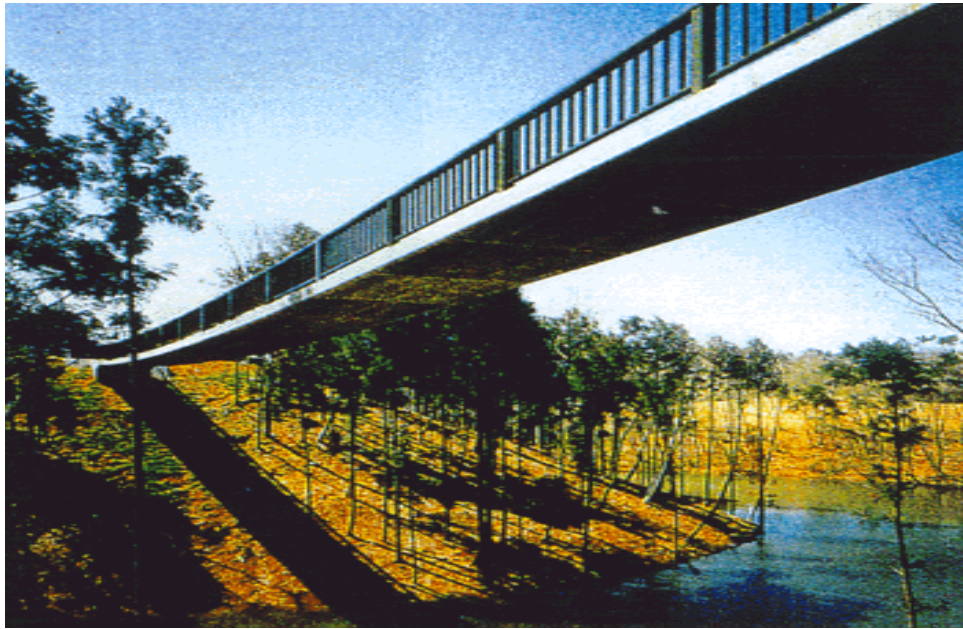
Figure 2.5. Birdie Footbridge (WTEC, 2001).
