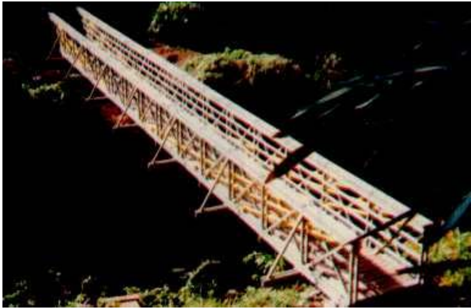
Figure 2.8. Haleakala Footbridge (Hull, 1996).
