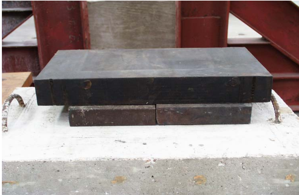
Figure 3.7. Elastomeric Bearing Support.
