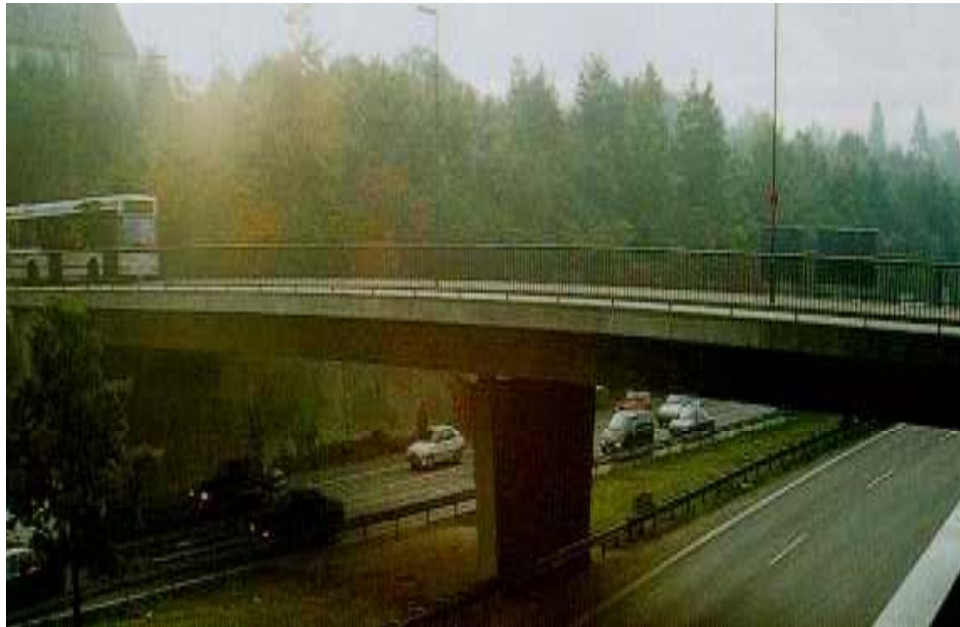
Figure 2.17. Ulenborgstrasse Bridge (FHWA, 1997) .
