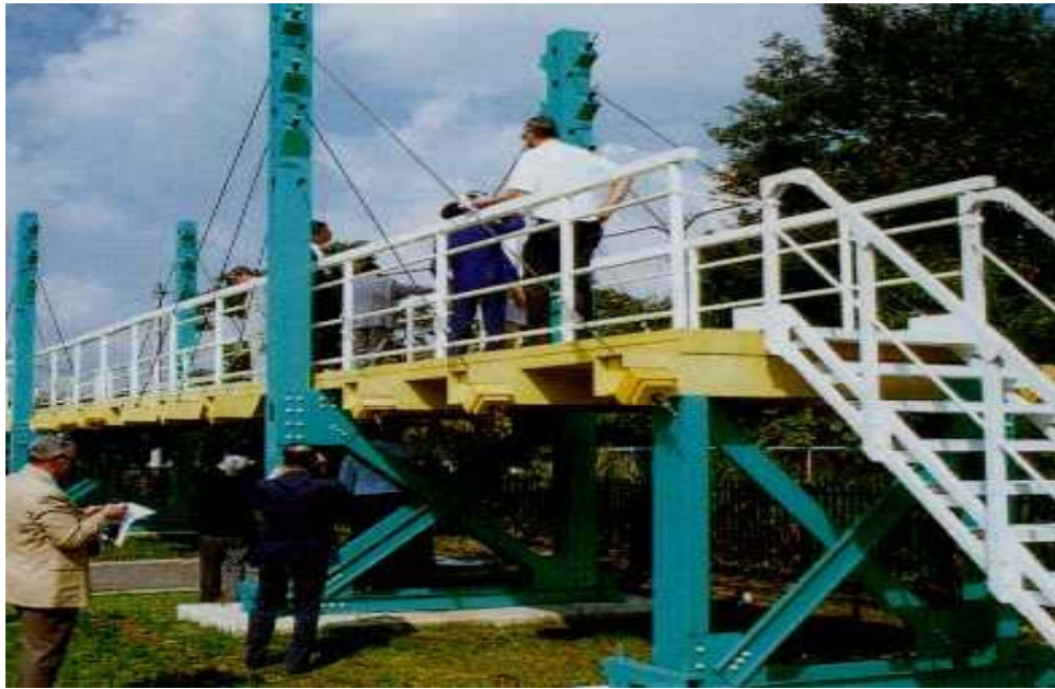
Figure 2.10. Tsukuba Public Works Footbridge (FHWA, 1997, CFI 1998).
