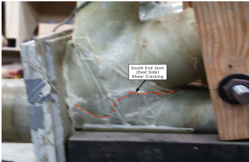
Figure 9.31. Wrap Shear Cracking at the South End Joint, East Arch.
