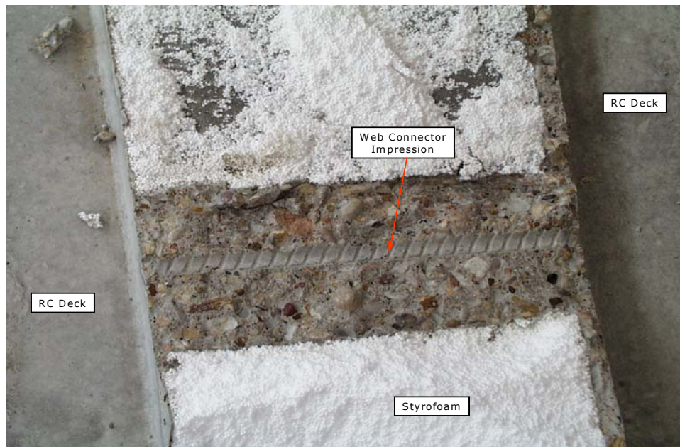
Figure 8.20. RC Deck Removed with Rebar Impression.
