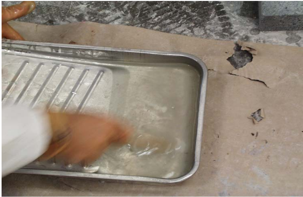
Figure 9.9. Wetting Fiberglass Fabric for Connection Type 2.
