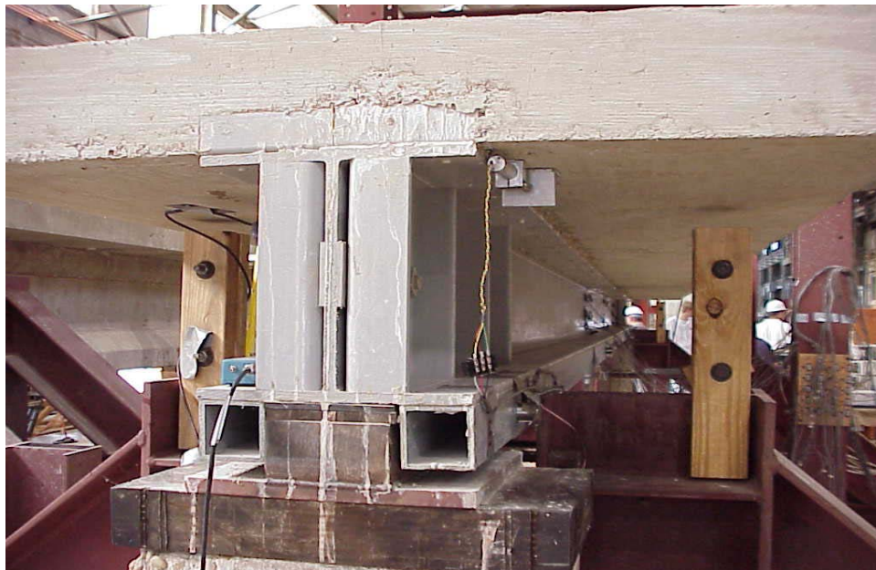
Figure 4.10. South End Support View.
