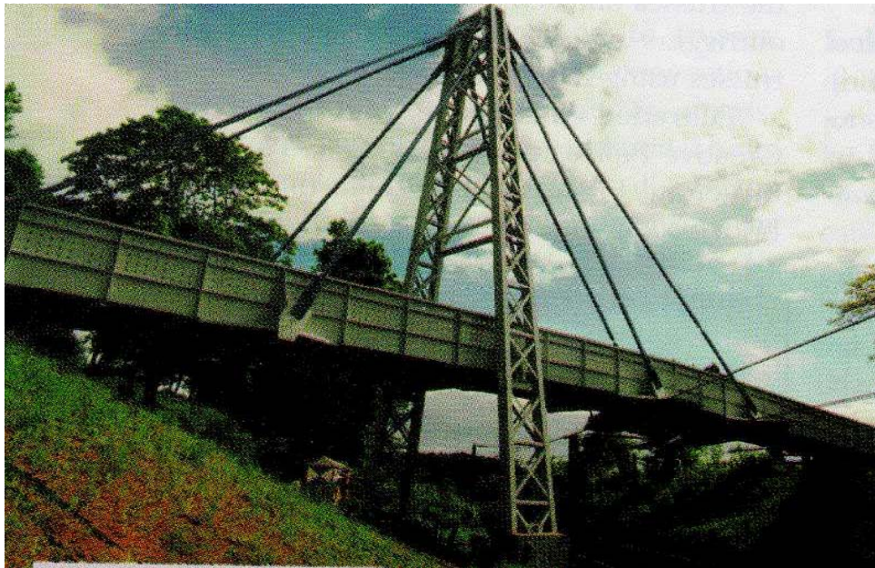
Figure 2.11. Kolding Bridge (CFI, 1998).
