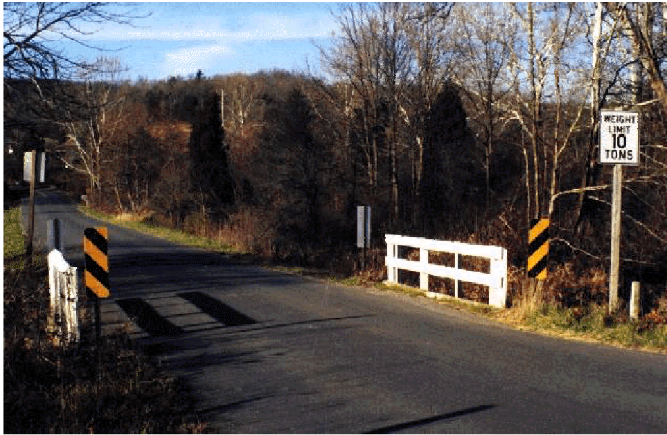
Figure 2.15. Tom's Creek Bridge (Before Repair) (Lesko, Hayes, 1998).
