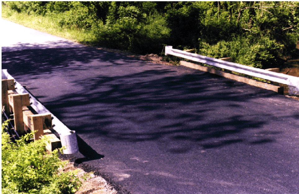
Figure 2.16. Tom's Creek Bridge (After Repair) (Lesko, Hayes, 1998).
