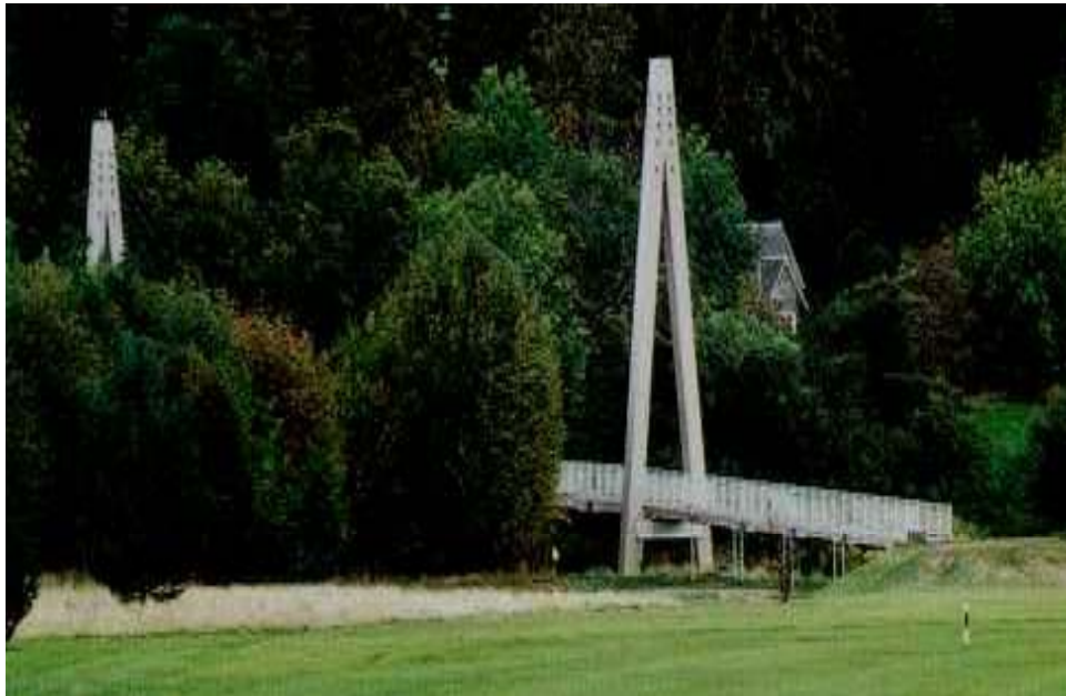
Figure 2.7. Aberfeldy Golf Club Footbridge (Johansen, 1995, FHWA, 1997).
