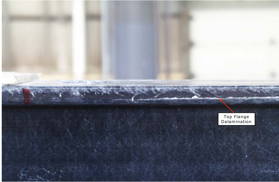
Figure 7.15. Specimen SW2 Top Flange Early Delamination.
