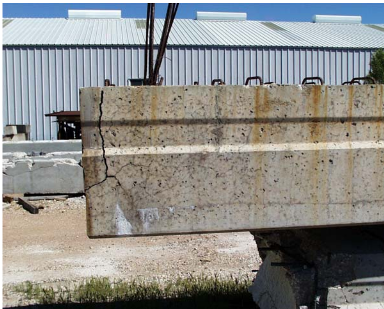
Figure 3.12 - Northwest end of BG4
