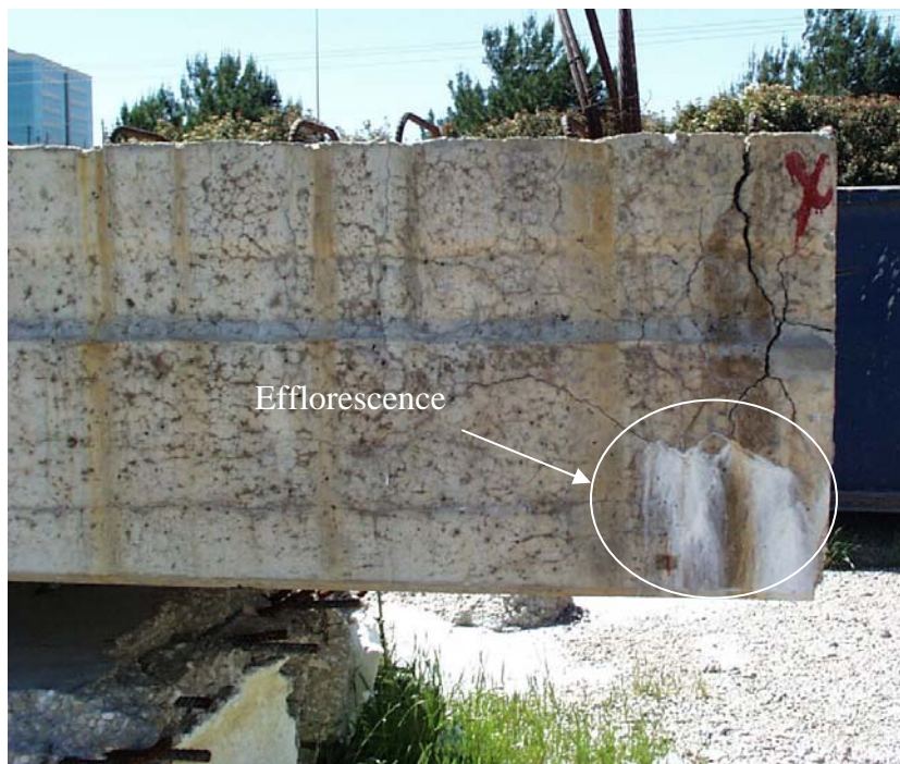
Figure 3.10 – Side View of A-End of BG4
