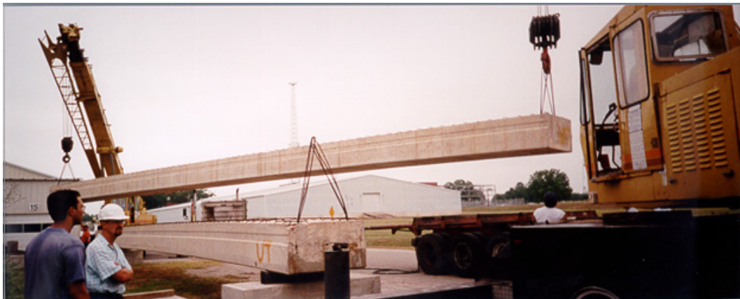
Figure 2.3 - Overall View of Box Girder
