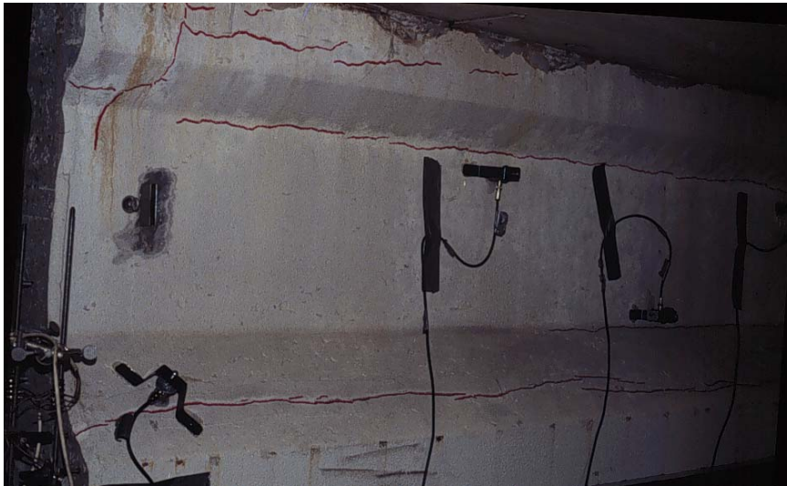
Figure 3.15 – East End of Girder 2
