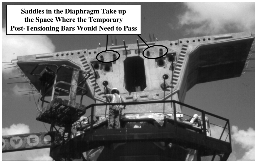
Figure 4.23 - The P16 interior anchorage segment after erection
