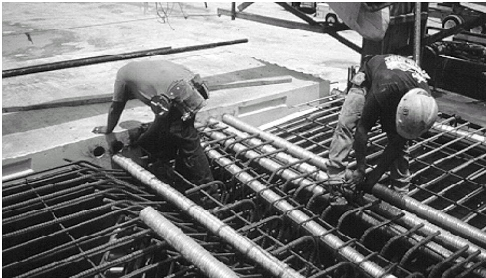
Figure 4.6 - Workers install post-tensioning tendon ducts
