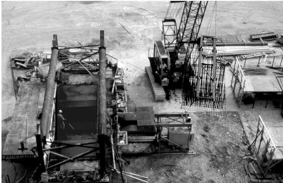
Figure 4.4 - Rebar cage is placed in the forms
