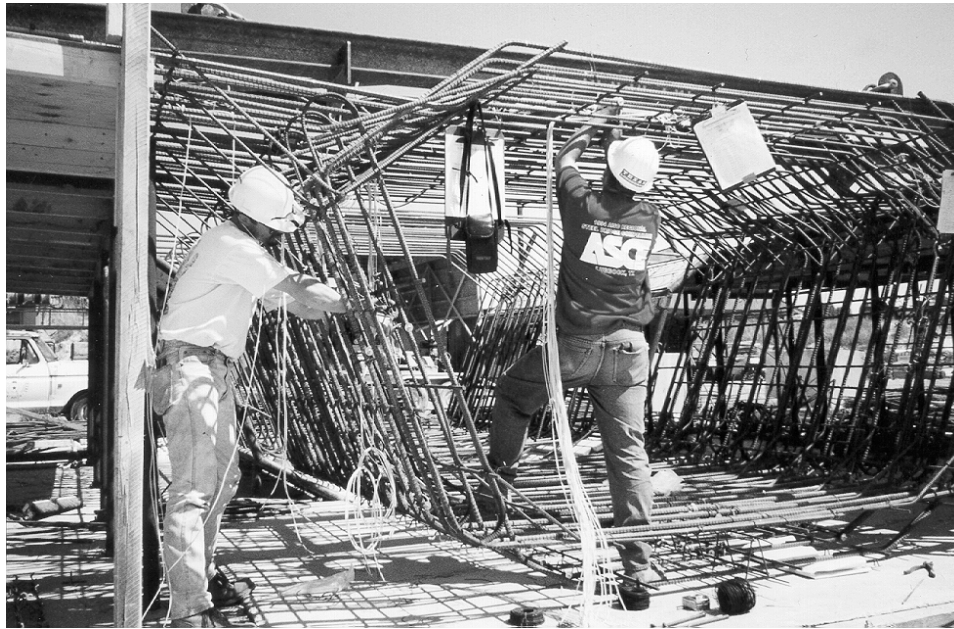
Figure 3.3 - Installation of concrete strain gauges
