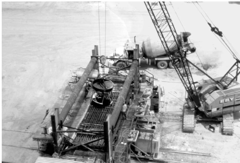
Figure 4.10 - A crane lifts a concrete bucket over the precasting bed
