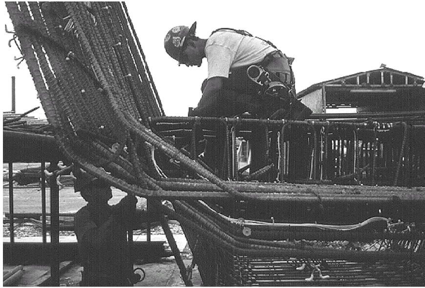
Figure 4.3 - Iron workers tie together a rebar cage
