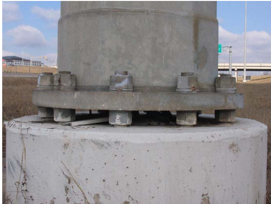
Figure 1.6 High Mast Double-Nut Base Connection (photo courtesy of Craig Rios)
