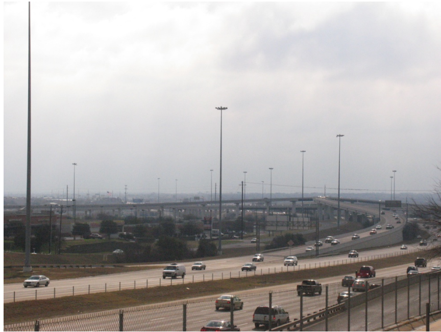
Figure 1.1 High Mast Towers at Highway Interchange (photo courtesy of Craig Rios)
