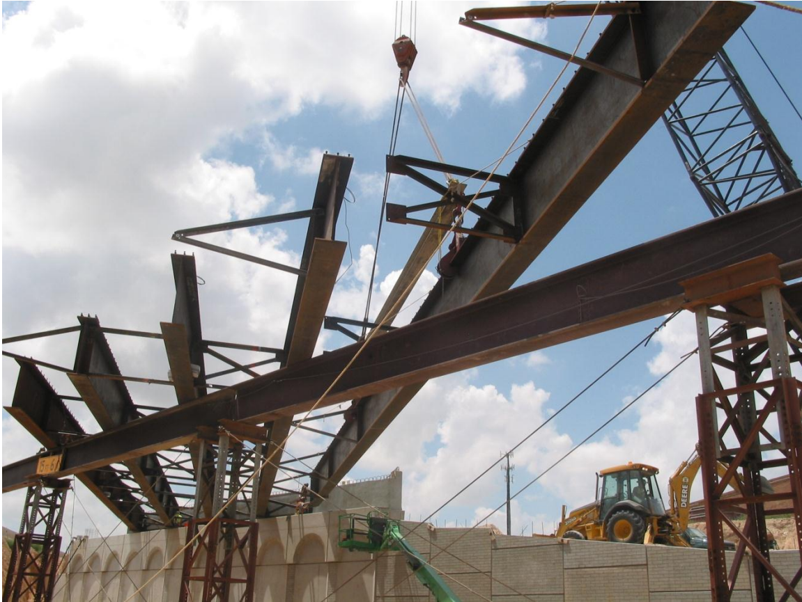
Figure 1-1: Cross-Frames during Construction of the Lubbock 19 th St. Bridge
