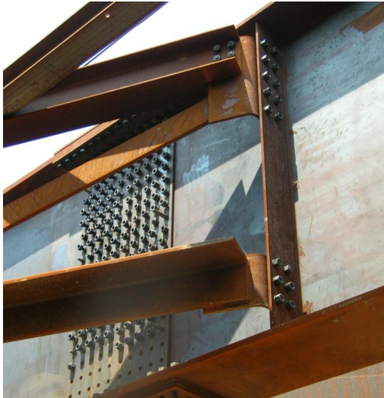
Figure 1-2: A Bent Plate Connection
