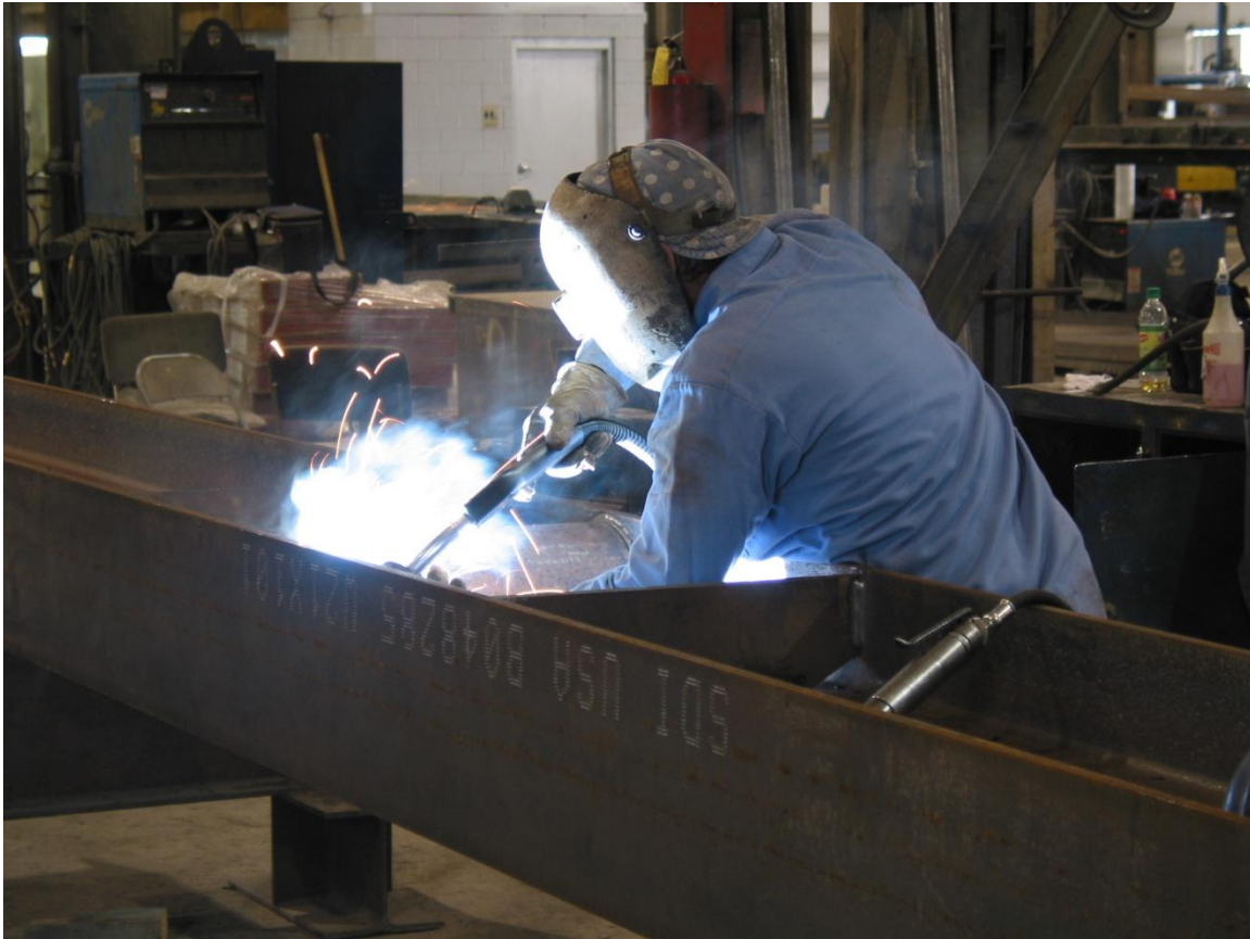
Figure 2-5: Welding Half-Pipe Stiffener to the Girder
