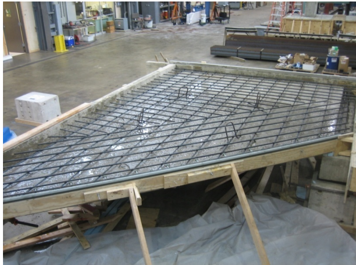
Figure 3.14 – Cast-in-Place Topping Reinforcement
