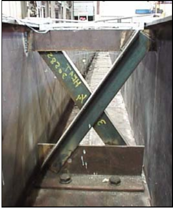
Figure 3.6 X-Brace at Support Location
