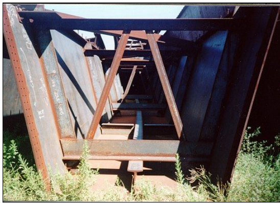
Figure 1.2 Cross-Section of U-Shaped Girder Segment (Gilchrist, 1997)
