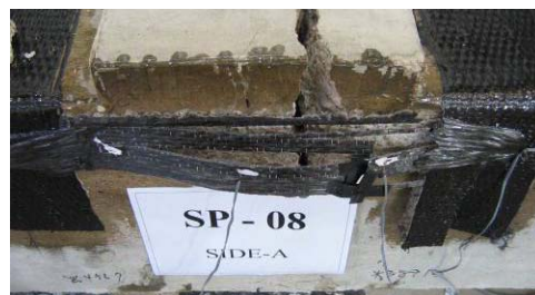
Figure 4.73 Failure Mode of Specimen No.8
