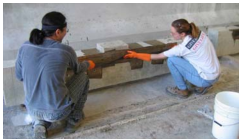
Figure 3.18 Placement of CFRP Materials
