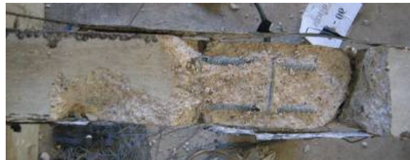
Figure 4.48 Failure Mode of Specimen No.6, After Removing Concrete Cover
