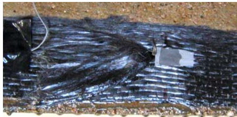
Figure 2.3 CFRP Anchor after Installation
