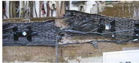
Figure 4.59 Failure Mode of Specimen No.7, Side-A, Fracture of CFRP Sheet
