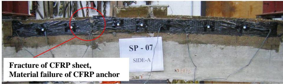
Figure 4.58 Failure Mode of Specimen No.7, Side-A
