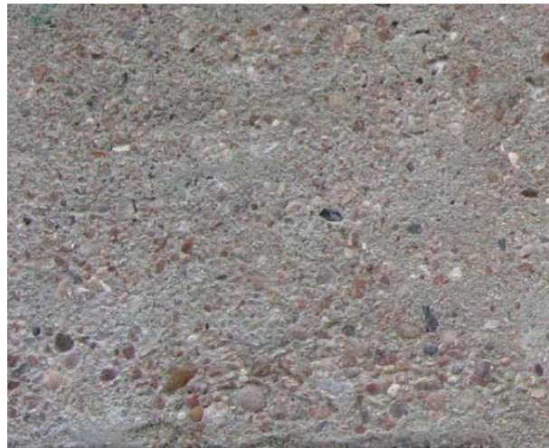
Figure 3.14 Over Blasted Surface
