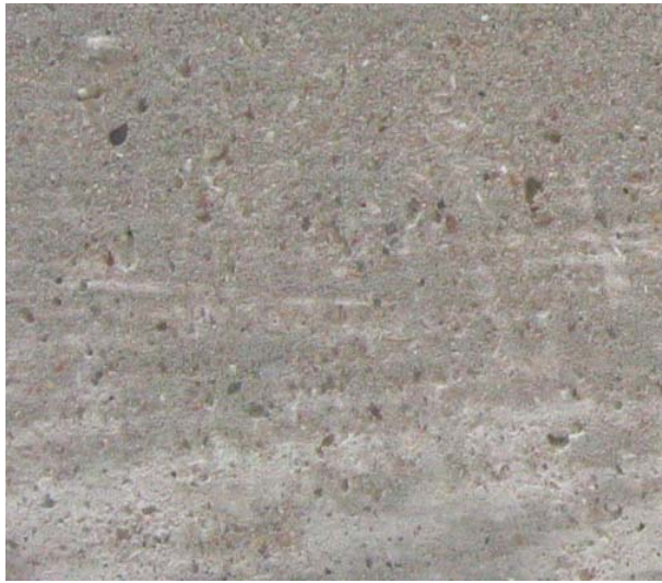
Figure 3.13 Regularly Blasted Surface
