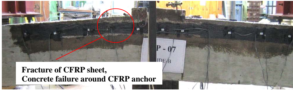
Figure 4.61 Failure Mode of Specimen No.7, Side-B
