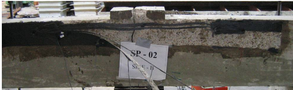
Figure 4.11 Failure mode of Specimen No.2, Side-B
