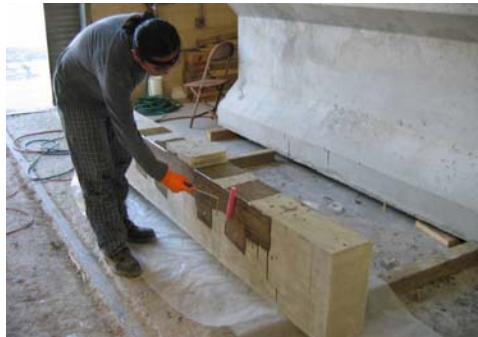
Figure 3.17 Saturation of Concrete Surface with Epoxy
