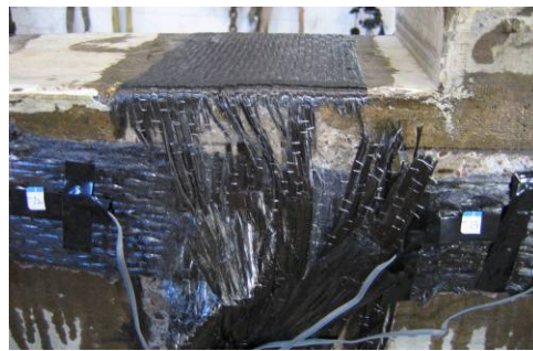
Figure 4.84 Failure Mode of Specimen No.9
