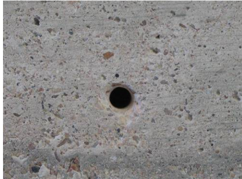
Figure 3.15 Hole for CFRP Anchor
