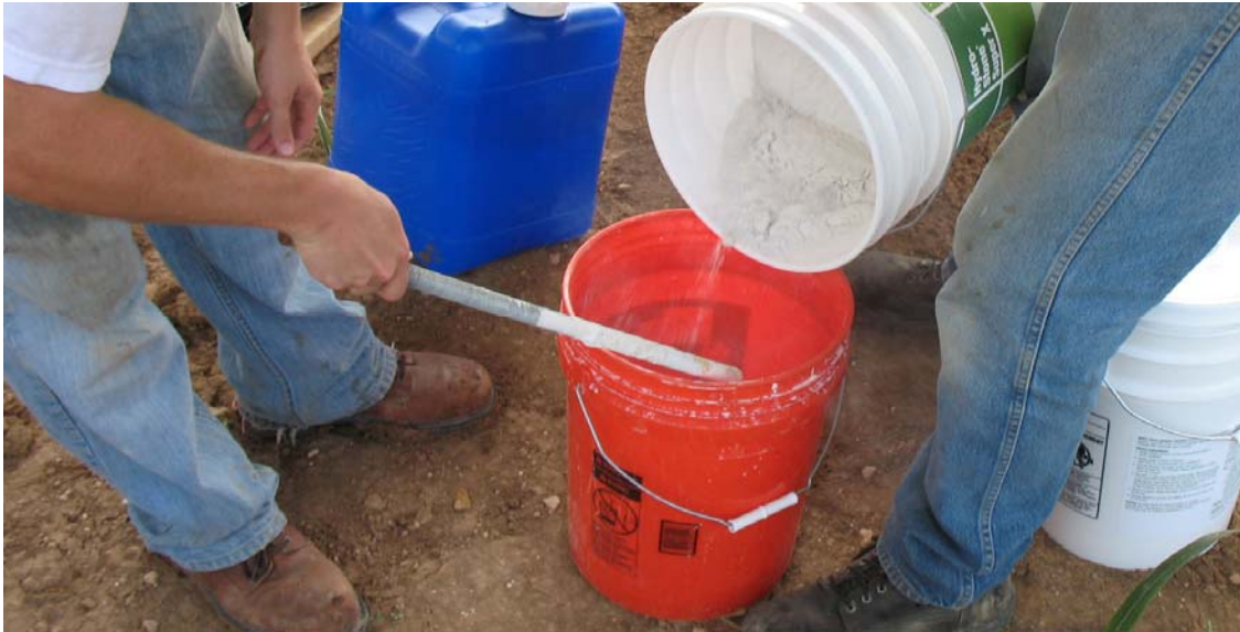
Figure 3-6 Mixing Hydro-Stone for Isolated Base
