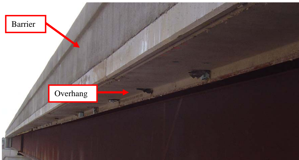
Figure 1-1 Bridge Deck Overhang
