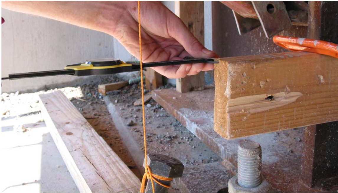
Figure 3-27 Control Rotation Measurement at Support of 19 th Street Bridge
