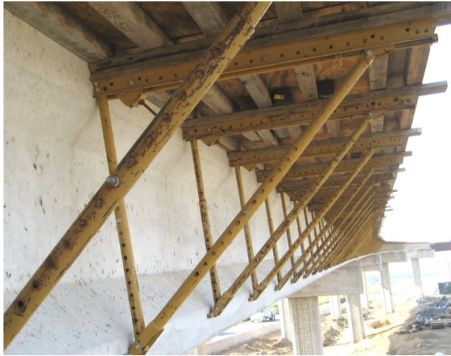
Figure 3-2 Overhang Brackets Used at SH 71-SH 130 Bridge
