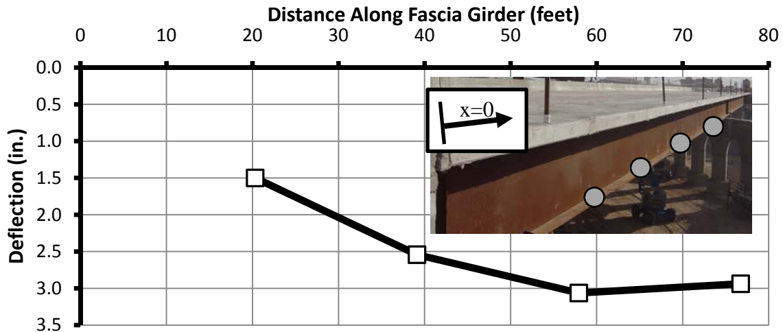
Figure 4-15 Vertical Deflection of Fascia Girder Due to Deck Pour
