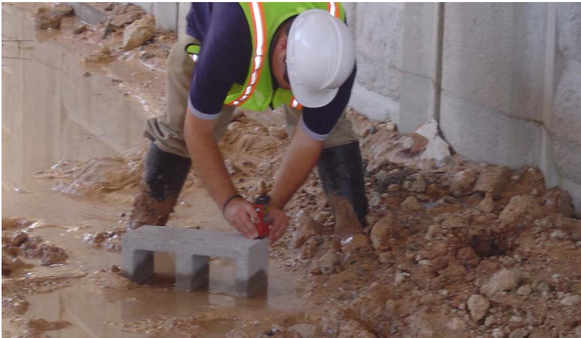
Figure 3-24 Vertical Deflection Measurement at 19 th Street Bridge
