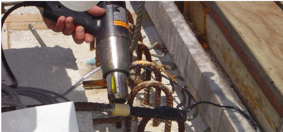
Figure 3-21 Heating Protective Tape on Top Bracing Bar
