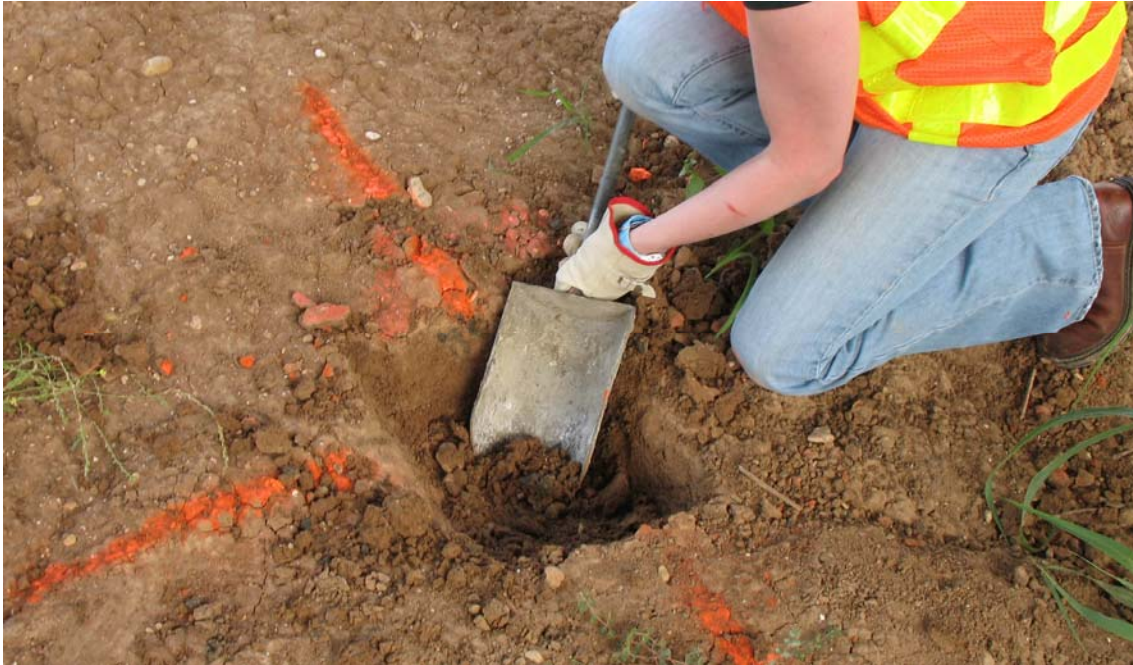
Figure 3-5 Hole for Isolated Base of Deflection Measurement
