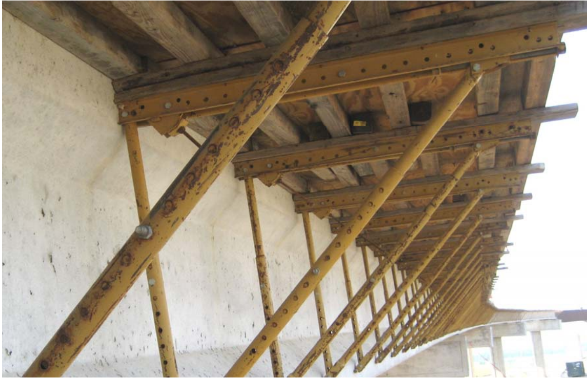
Figure 2-14 Overhang Brackets Used at SH 71-130 Bridge
