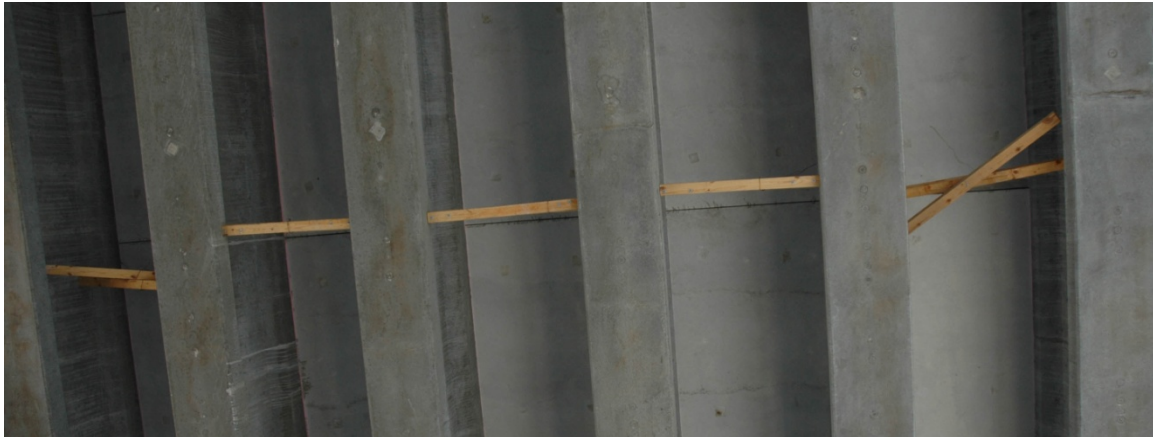
Figure 2-5 Effect of Twist on Timber Blocking
