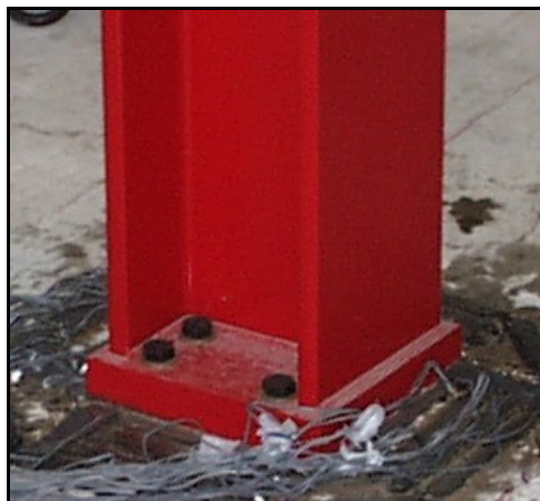
Figure 2.5 Steel Column to Concrete Slab Connection
