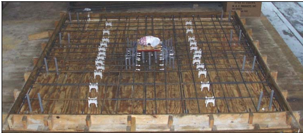
Figure 2.16 Upgrade Specimen B4-S, Prior to Casting Concrete
