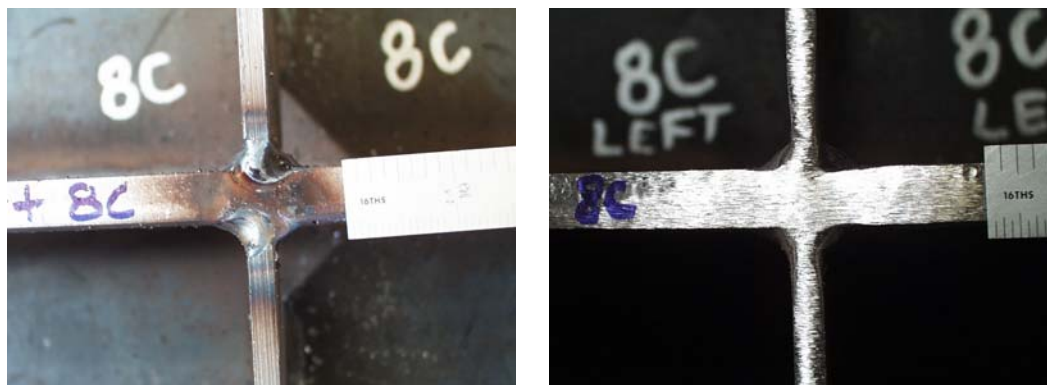
Figure 2-27: Before and After Flange Grinding
