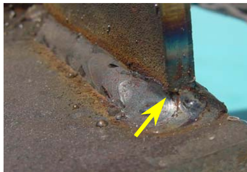
Figure 2-22: Specimen A Stiffener Undercut
