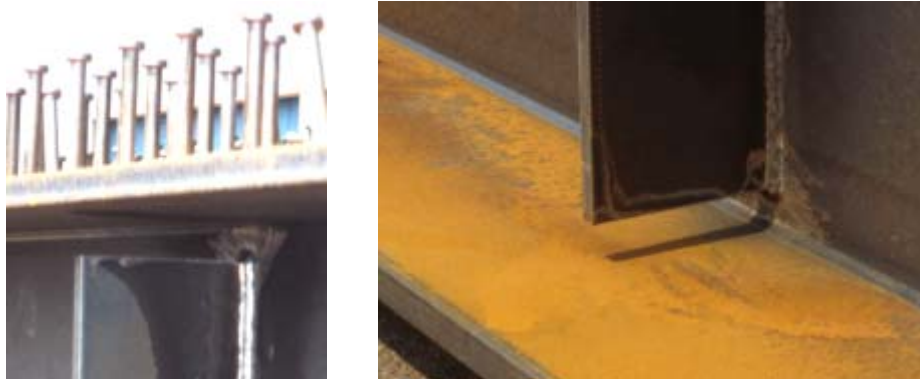
Figure 1-7: Wrapped Intermediate Stiffener Welds
