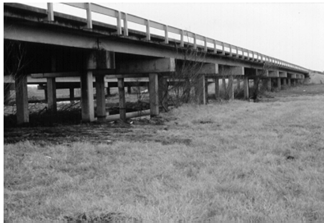
Figure 2-15 West Elevation of the Bridge
