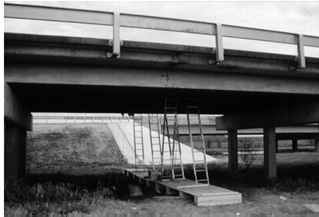
Figure 2-16 Platform Used for Accessing the Underside of the Bridge
