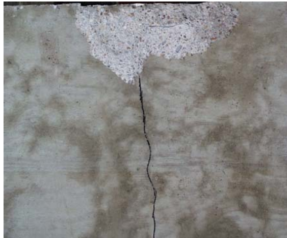
Figure 3.3 Failure Mode of Specimen S1-1
