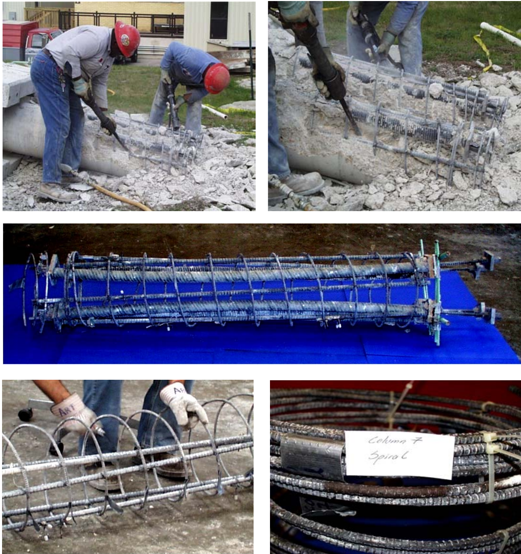
Figure 5.47 Concrete Removal and Reinforcement Dismantling.
