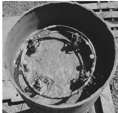
Top of Column Prior to Capping
