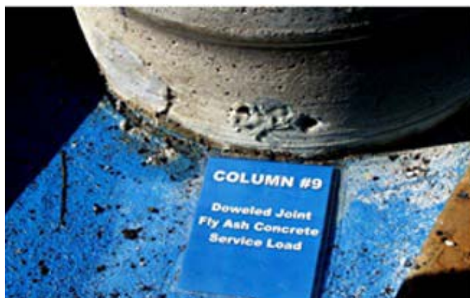
Figure 5.56 Condition of Specimen DJ-FA-S at the End of Testing.
