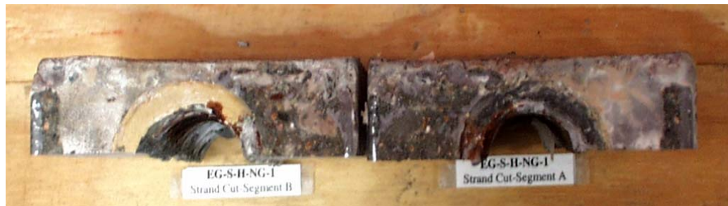
Figure 3.49 Incomplete Epoxy Coverage in Epoxy/Gasket Joint (EG-S-H-NG-1)
