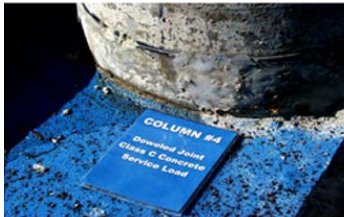
Figure 5.58 Condition of Specimen DJ-TC-S at the End of Testing
