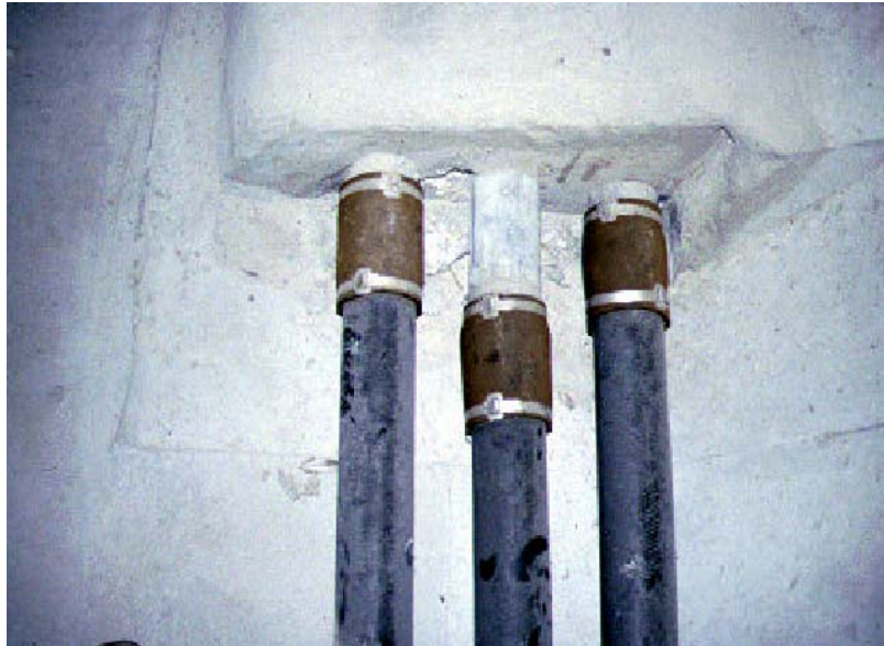
Figure 2.5 Plan View of Slipped Tendon at Deviation Saddle Niles Channel Bridge 2.10
