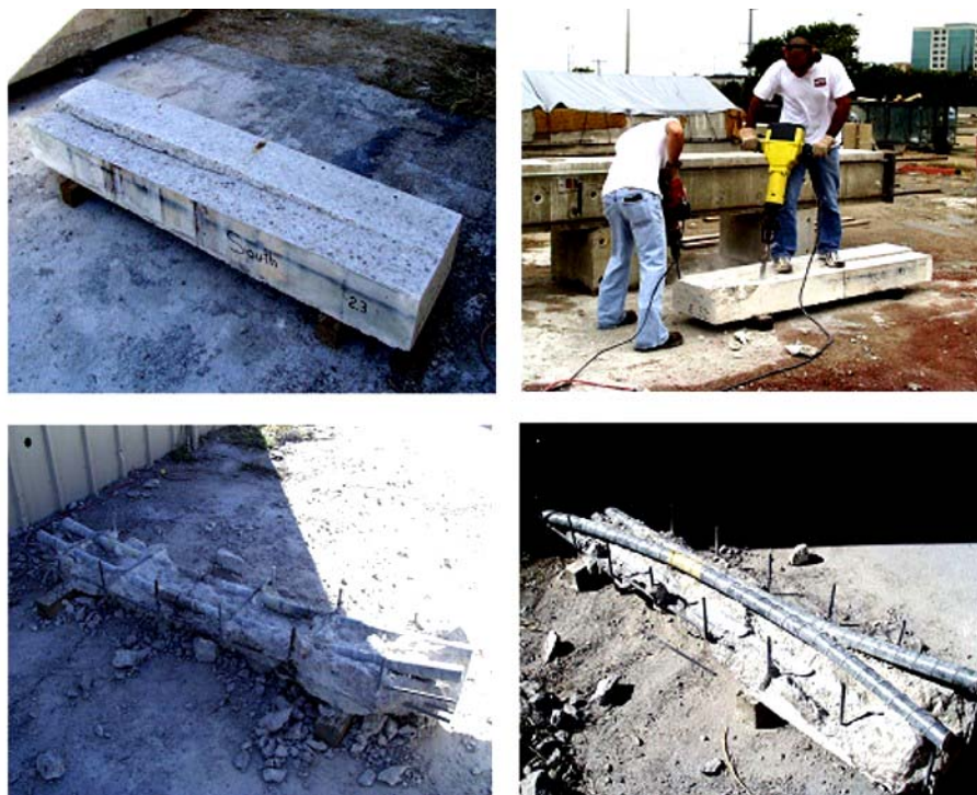
Figure 4.64 Concrete Removal to Expose Duct and Mild Steel
