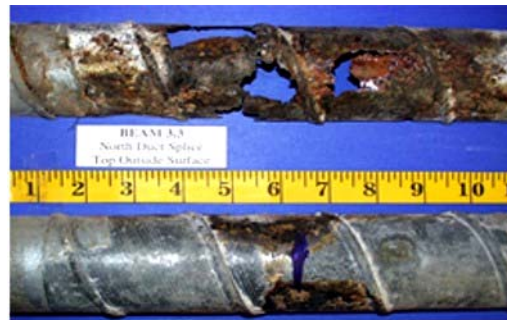
Figure 4.93 Specimen 3.3 – North Duct Splice
