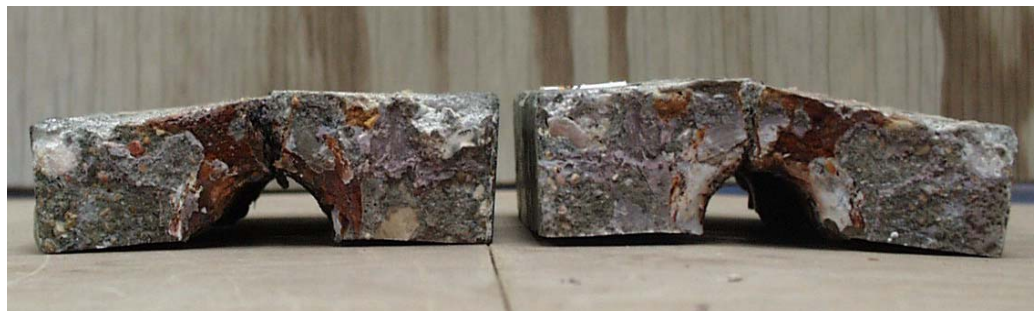
Figure 3.43 Incompletely filled Epoxy Joint (SE-S-M-CI-1)
