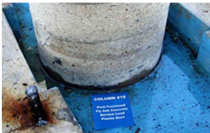
Figure 5.69 Condition of Specimen PT-FA-S-PD at the End of Testing
