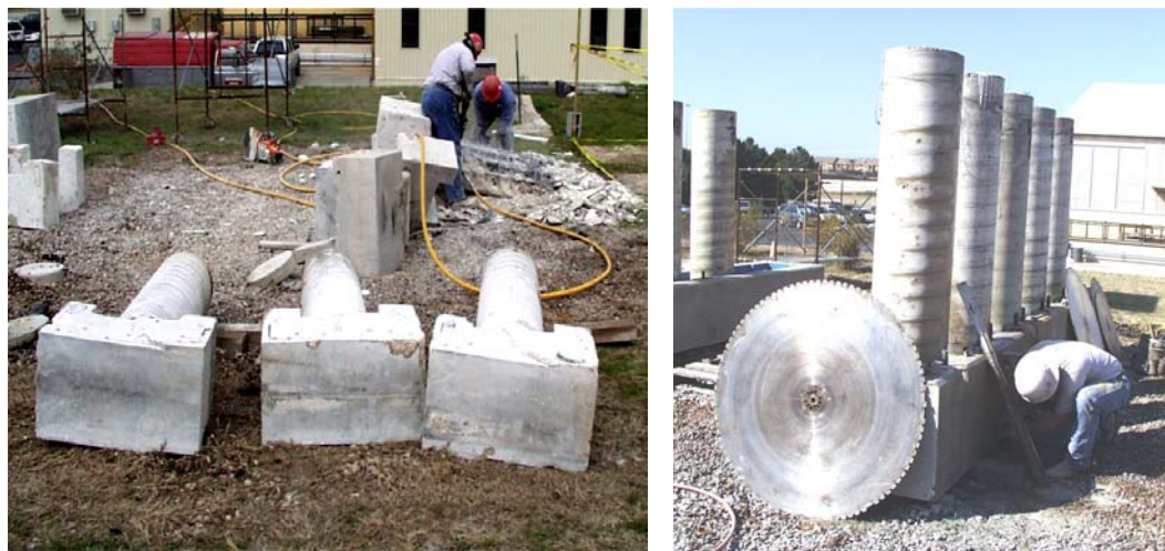
Figure 5.46 Saw Cutting of Column Foundation.
