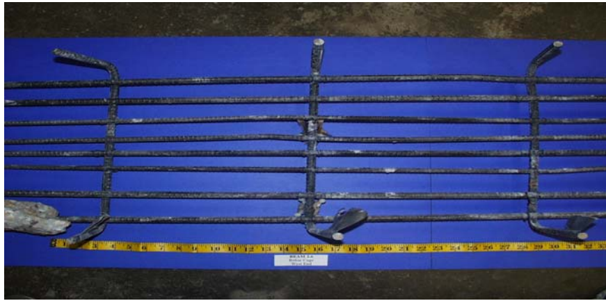
Figure 4.66 Mild Steel Reinforcement Cage
