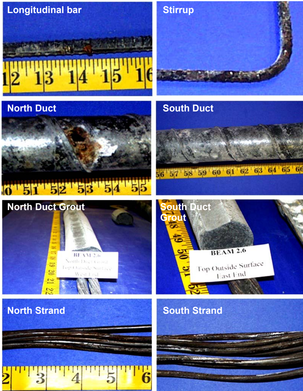
Figure 4.112 Specimen 2.6 – Reinforcing Elements
