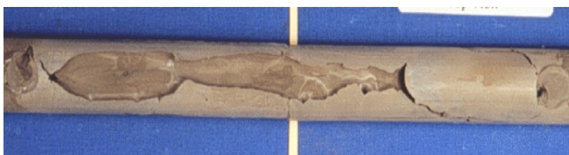
Void Caused by Entrapped Air, Bleed Water or Incomplete Filling (from Reference 3.8)
