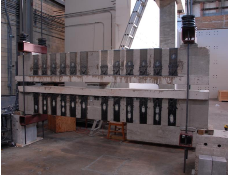
Figure 3-4 Long-term load test setup
