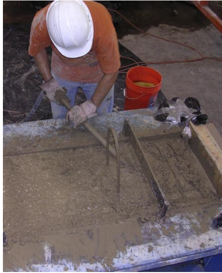
Figure 3-18 Vibrating the concrete
