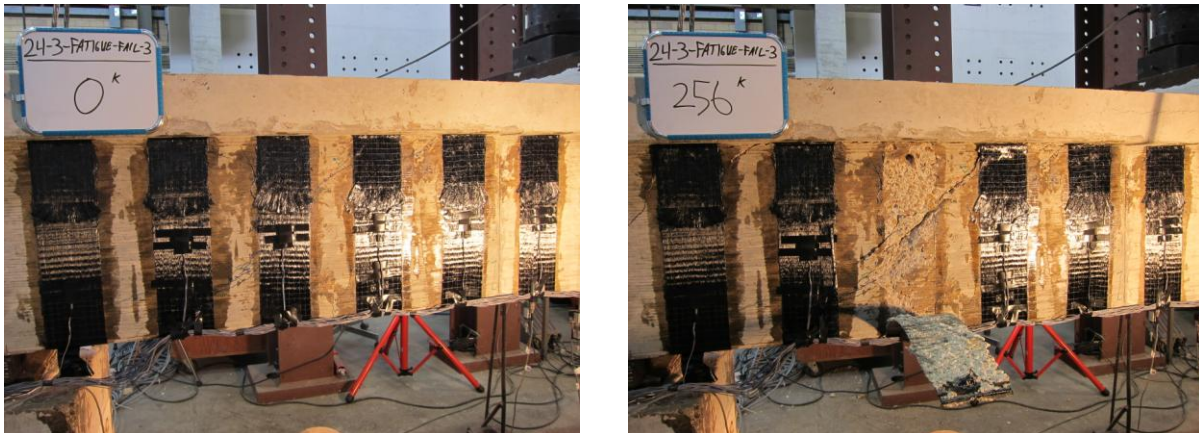
Figure 4-25 24-3-Fatigue-Fail-3 before (left) and after (right) loading
