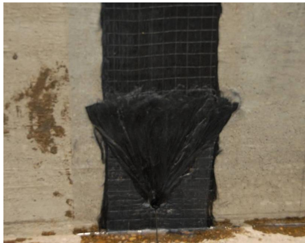
Figure 3-24 CFRP anchor with 60-degree fan angle
