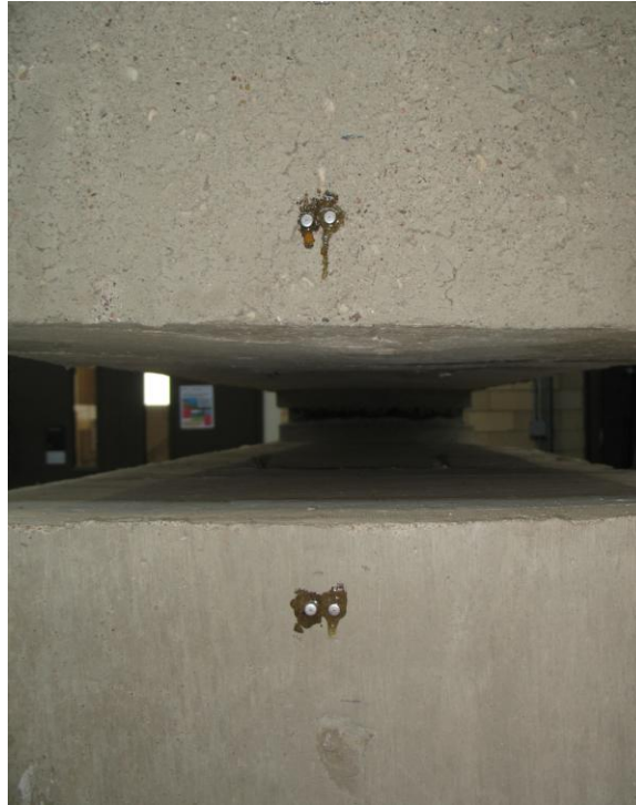
Figure 3-54 DEMEC points used to track changes in end displacements
