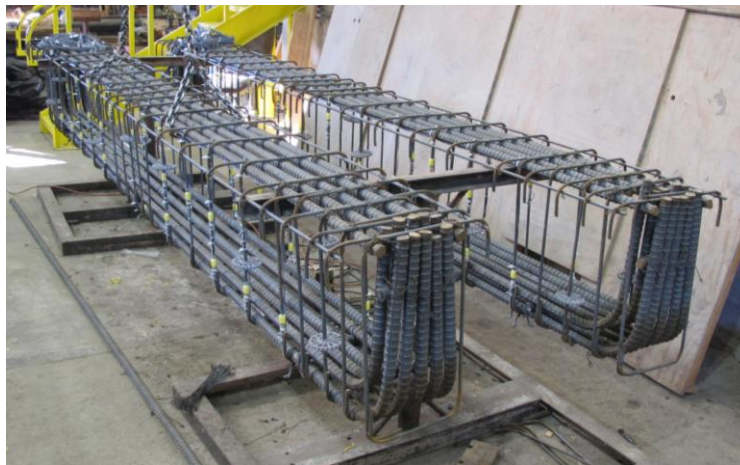
Figure 3-13 Steel reinforcement cage with stirrups spaced at 10-in.
