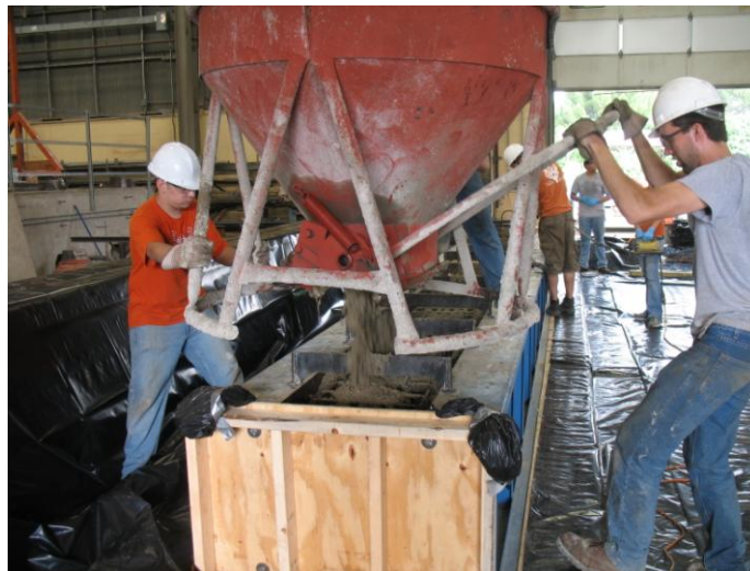
Figure 3-17 Placing of the concrete using 1 cubic yard concrete bucket
