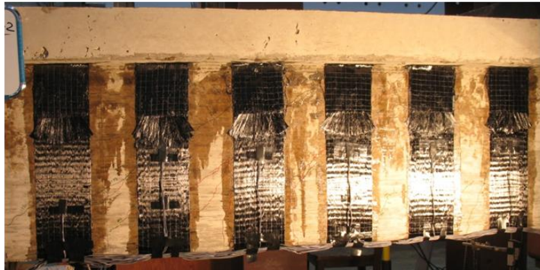
Figure 4-20 24-3-Fatigue-Fail-2 at 0-kips applied load (0-kips applied shear)
