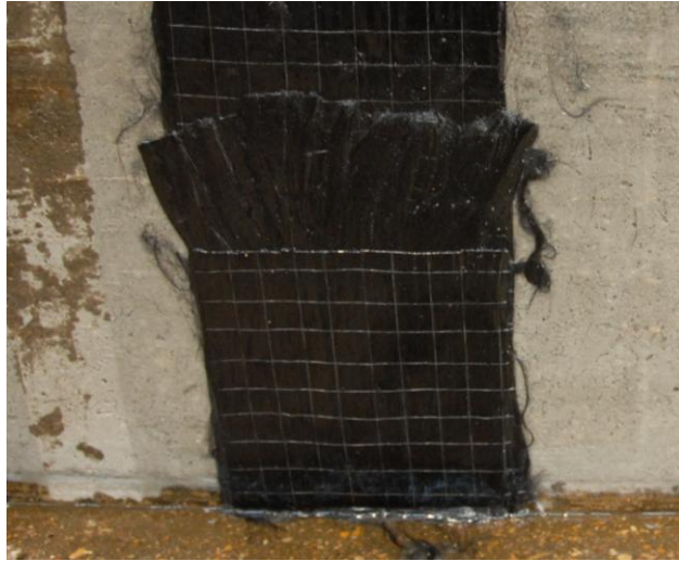
Figure 3-25 Completed CFRP anchor installation
