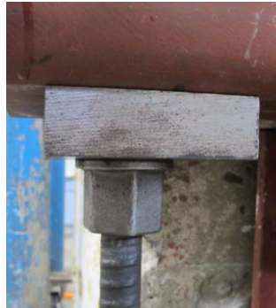
Figure 3-36 Dywidag anchorage system
