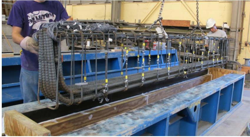
Figure 3-14 Placing of the steel reinforcement cage
