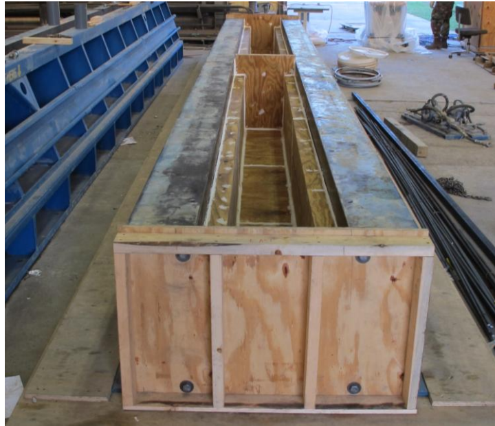
Figure 3-11 Assembled formwork for two specimens
