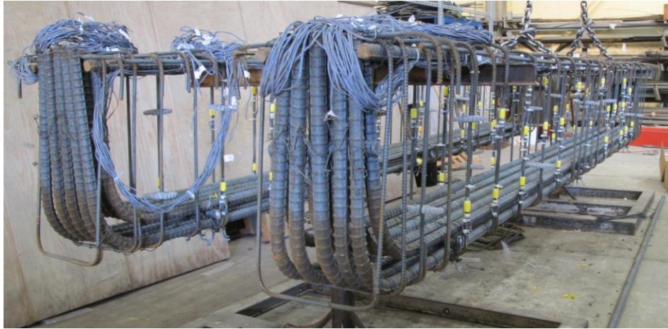
Figure 3-42 Reinforcement cages after installation of steel strain gauges
