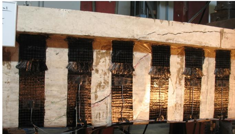
Figure 4-16 24-3-Fatigue-Fail-1 at 214-kips applied load (107-kips applied shear)
