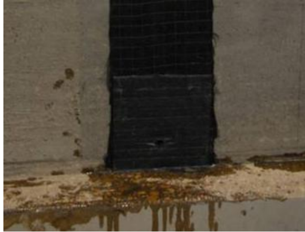
Figure 3-23 Placement of CFRP patch prior to insertion of anchor
