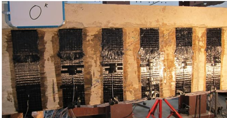
Figure 4-28 24-3-Fatigue-Fail-3 at 0-kips applied load (0-kips applied shear)
