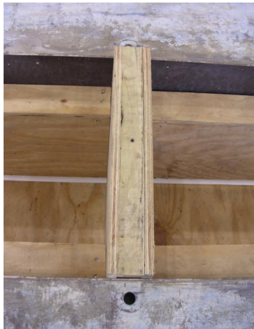
Figure 3-9 Internal form divider
