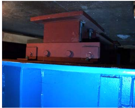
Figure 3.9 Buttress/Bulkhead Connections
