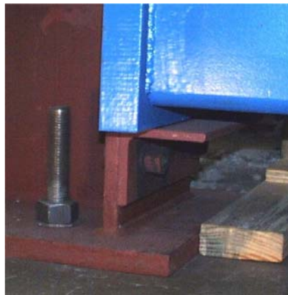
Figure 3.11 Column/Buttress Connection
