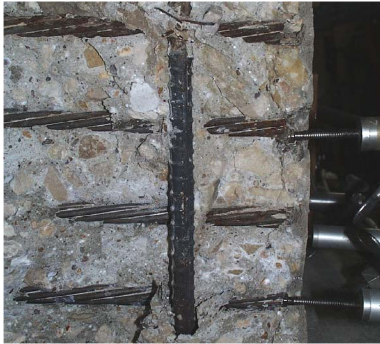
Figure 4.32 Slip of exterior prestressing strands after failure of BG3S
