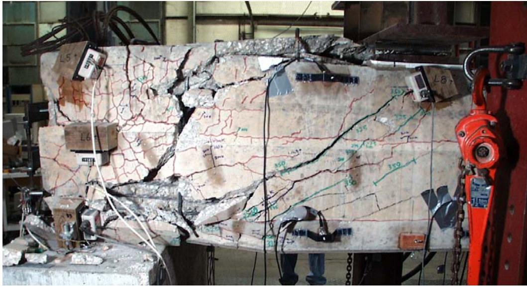
Figure 4.29 Failure of the east web of BG3S after 3,328,600 load cycles and a 365 kip (1620 kN) quasi-static load
