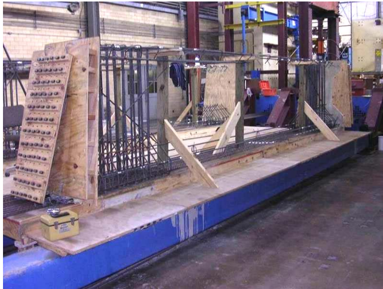
Figure 3.14 AASHTO Type IV beam during fabrication.
