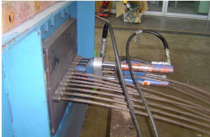
Figure 3.26 Single strand stressing operation.
