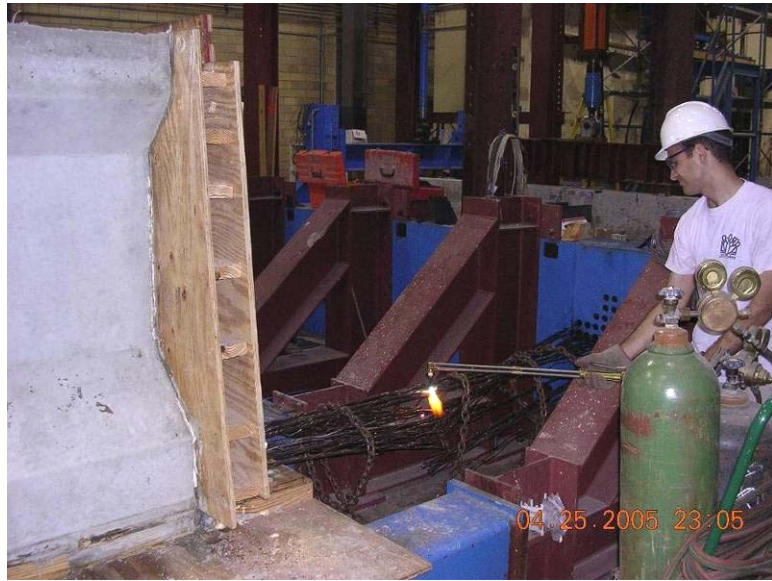
Figure 3.31 Torch-cutting prestressing strands.
