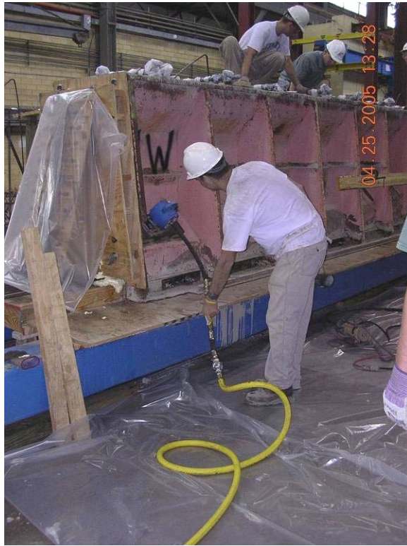
Figure 3.28 Form vibrators used to consolidate concrete.
