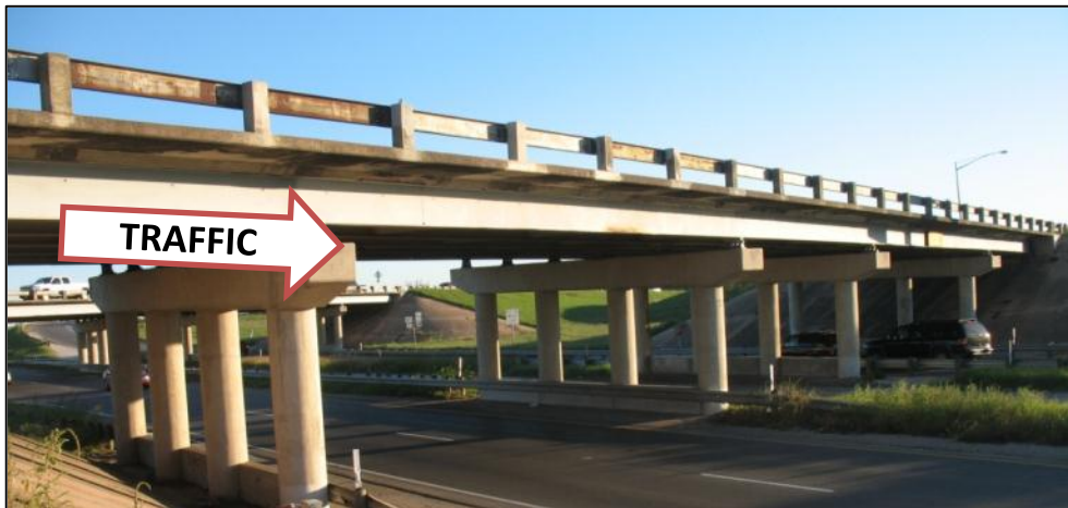
Figure 3.13 TX-71E Bridge over US-183N.
