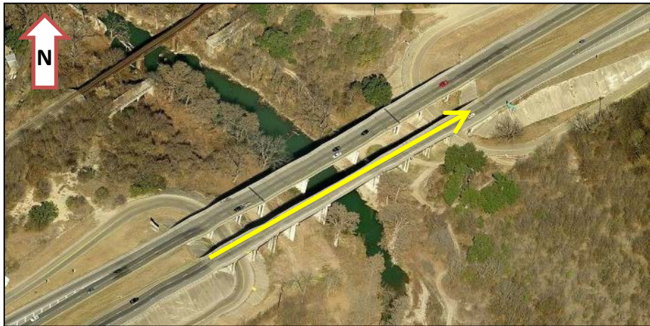
Figure 3.4 Aerial view of Medina River Bridge showing direction of traffic (Google Maps, 2011).
