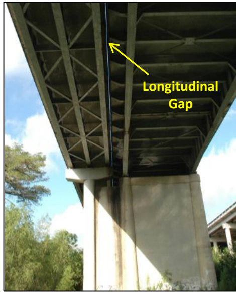
Figure 3.3 Longitudinal gap between original bridge (right) and plate girder bridge constructed in 1971 (left).
