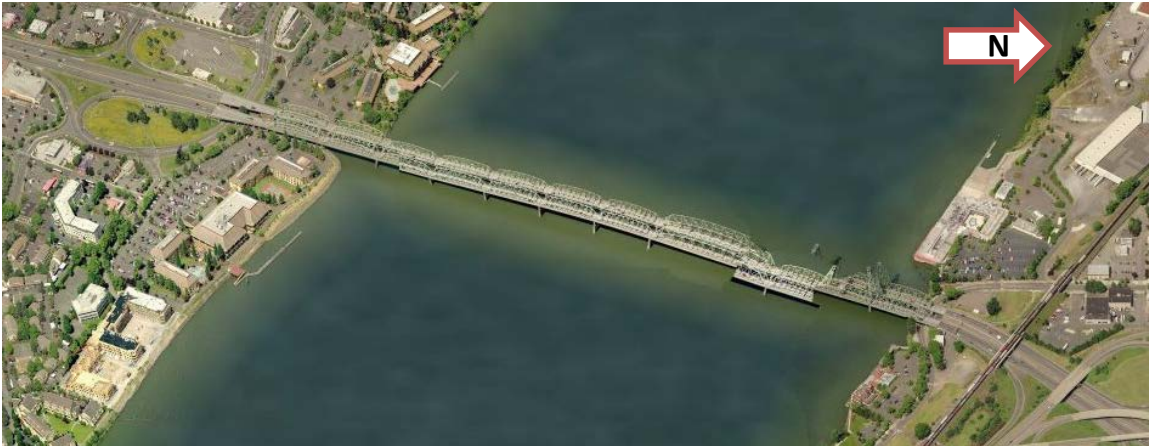
Figure 3.37 Aerial view of I-5 Portland-Vancouver Bridge over Columbia River (Google Maps, 2011).
