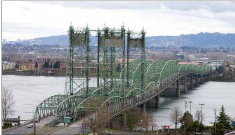
Figure 3.35 I-5 Portland-Vancouver Bridge over Columbia River from north end (Wikipedia, 2011).
