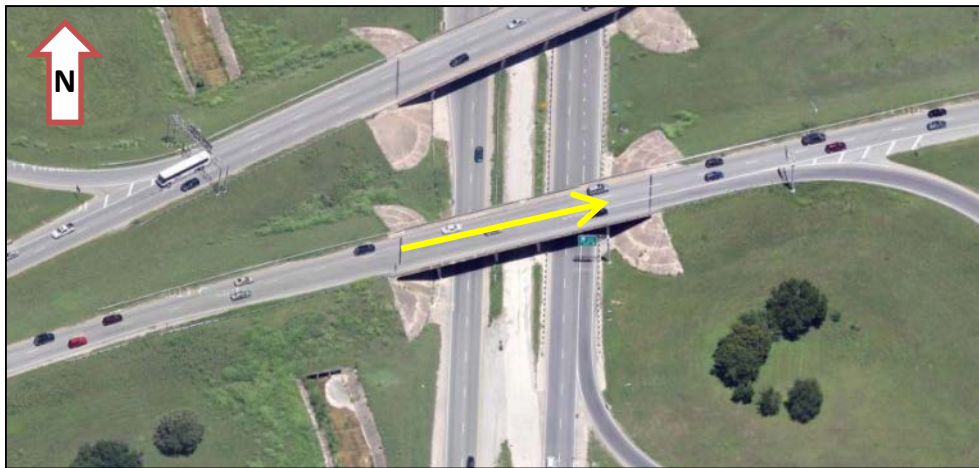
Figure 3.15 Aerial view of TX-71E Bridge showing direction of traffic (Google Maps, 2011).
