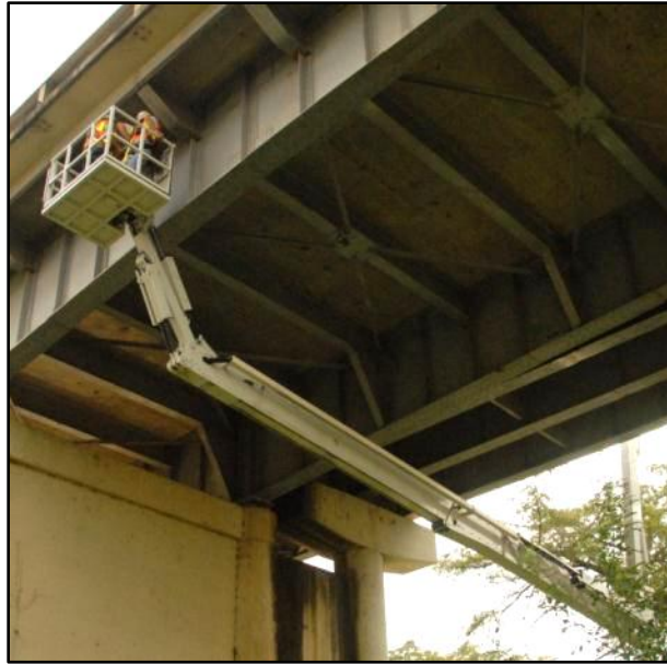
Figure 1.2 Detailed visual inspection of a fracture-critical bridge.
