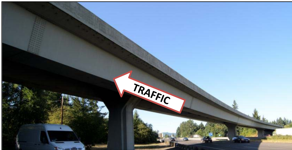
Figure 3.28 I-205W to I-5S Interchange Bridge (Lindenberg, 2011).
