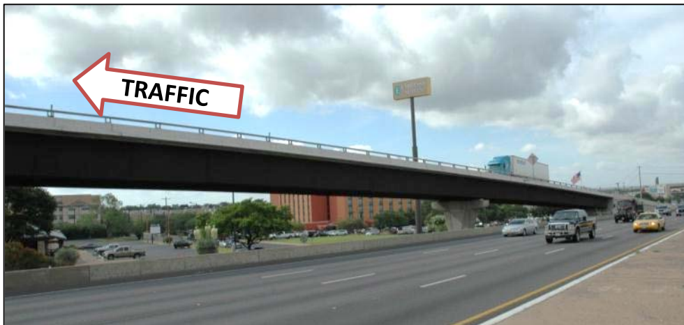
Figure 3.20 I-35N to US-290E Direct Connector Bridge.
