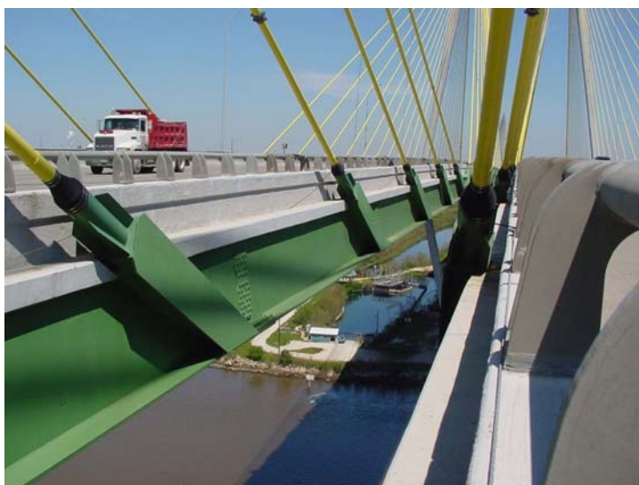
Figure 2-5: Cable Anchorage Deck
