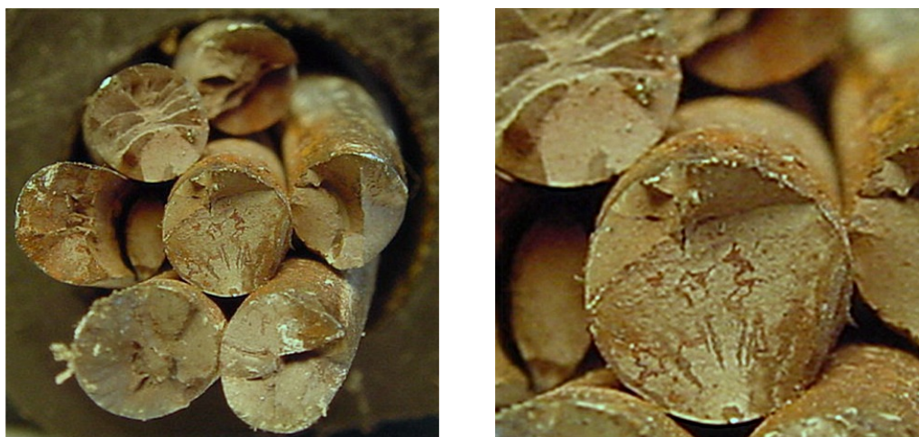
Figure 4-30: Fracture Surfaces – Strand #1 – Tower Anchorage – Specimen #2
