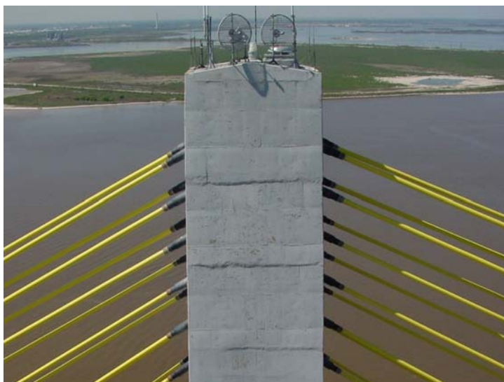
Figure 2-4: Cable Anchorage Tower
