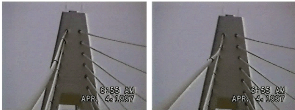
Figure 1-5: Stay Cable Vibrations
