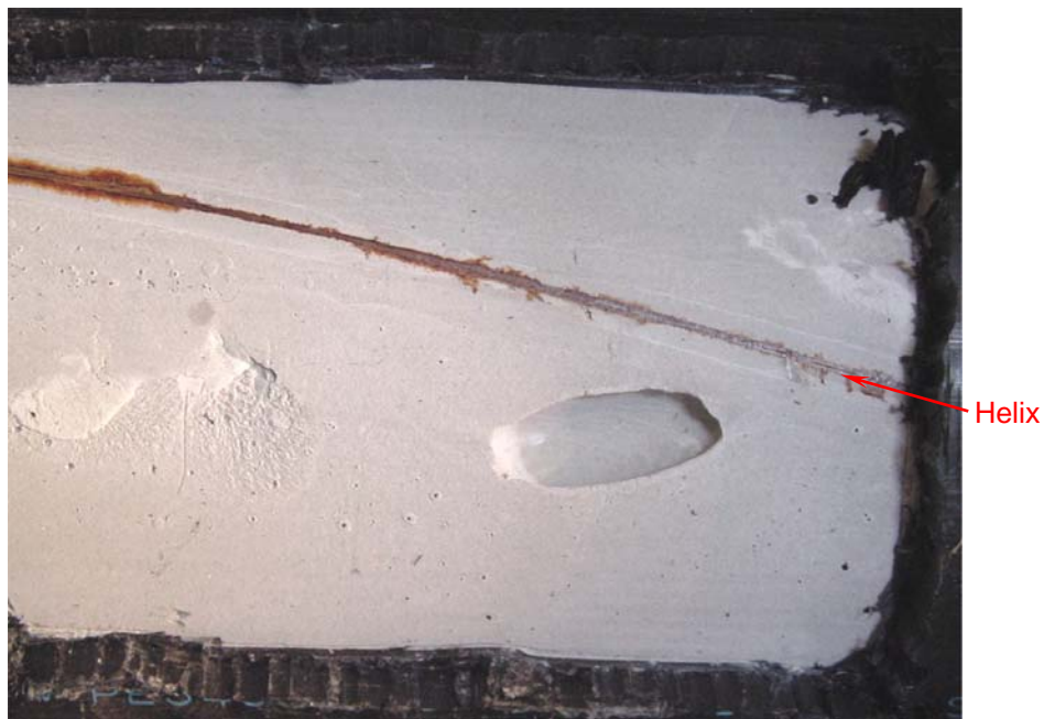
Figure 4-7: Grout Surface Defect and Corrosion on Helix – Specimen #1
