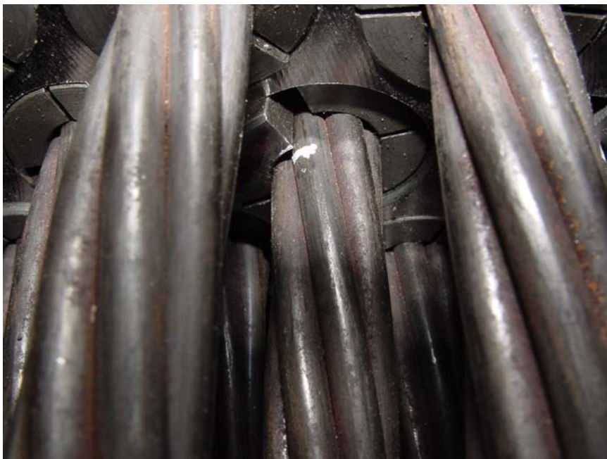
Figure 3-31: Unequally Seated Wedges
