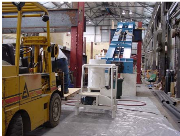
Figure 3-28: Setup for Grouting
