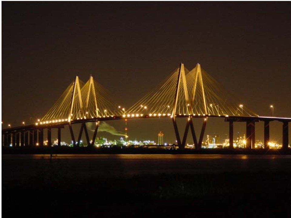
Figure 2-1: Fred Hartman Bridge at Night
