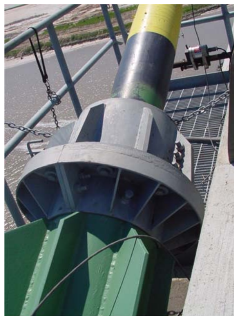
Figure 1-9: Freyssinet Damper
