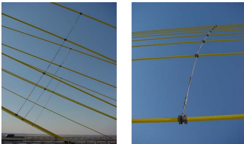
Figure 1-7: Cable Restrainer
