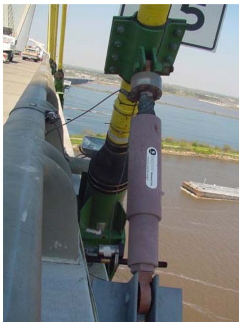
Figure 1-8: Linear Damper
