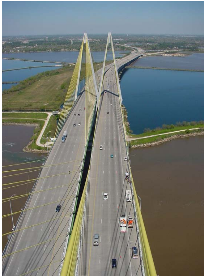
Figure 2-2: Bridge Deck seen from the Tower
