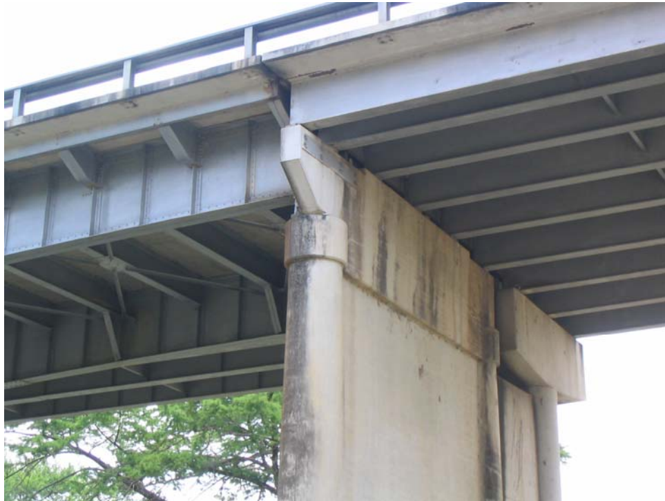
Figure 5-5: Transition from Simple Span to Anchor Span
