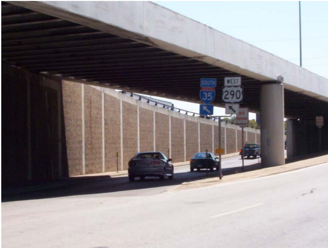
Figure 3-3: Southeast View of Exit Ramp
