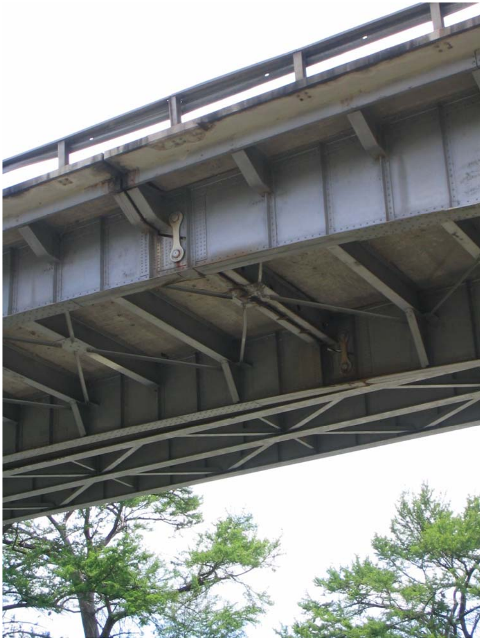
Figure 5-4: Close-Up of the Cantilevered Span and Hinge
