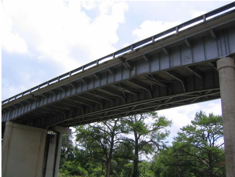
Figure 5-3: Center Span of Medina River Bridge
