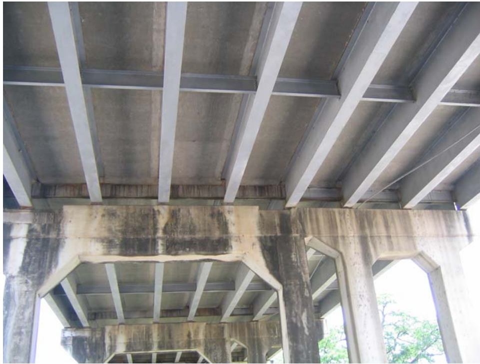
Figure 5-1: Underside of the 48-ft Spans on the Medina River Bridge
