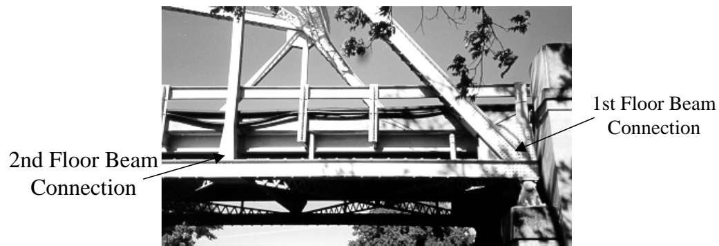
Figure 4.13 Floor Beam to Truss Connections
