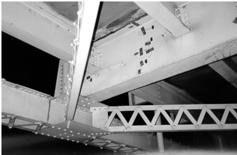
Figure 4.3 Connection of 2nd Floor Beam to Truss
