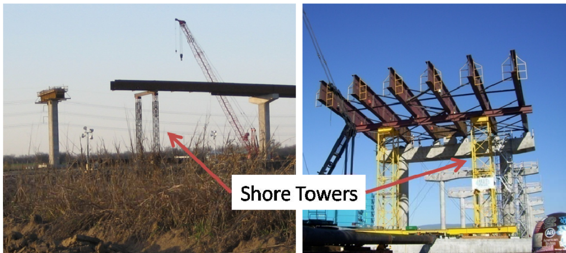
Figure 4.1: Shore Towers under Partially Constructed Bridges
