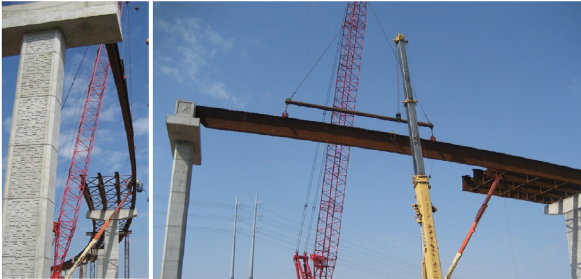
Figure 4.22: Single Girder Segment Lifted for a Particular Cross Section
