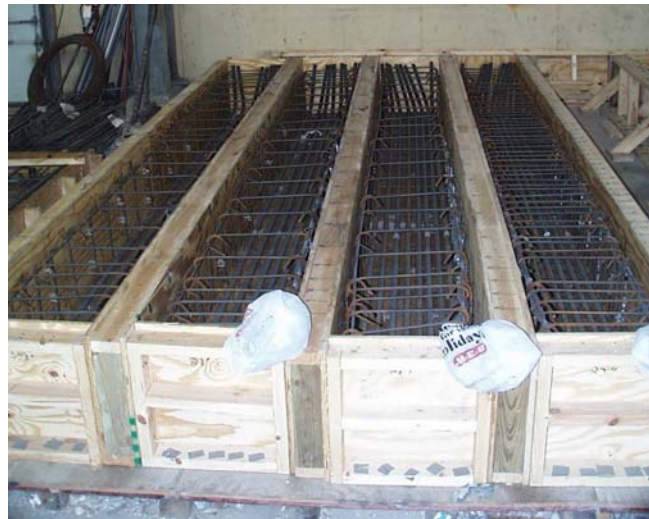
Figure 2.4 Cages placed in forms (set I)
