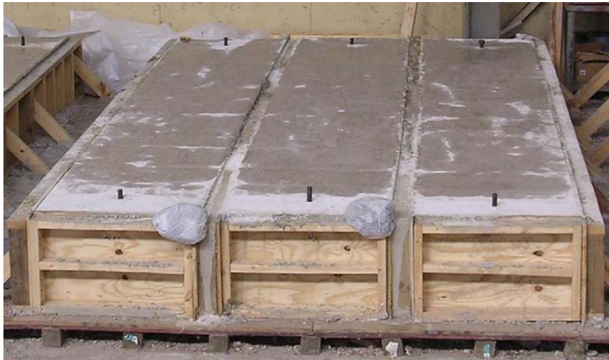
Figure 2.7 Pouring of concrete (set II)
