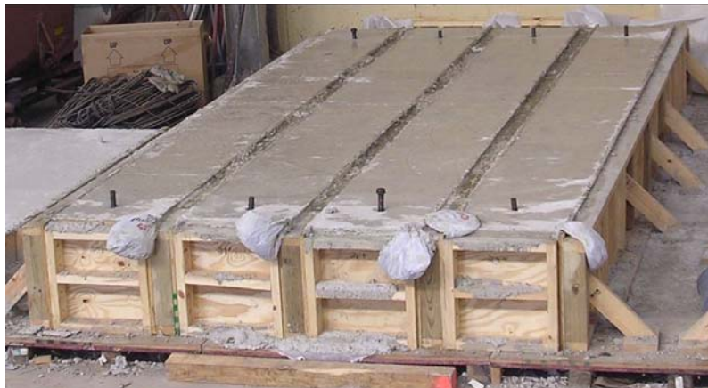
Figure 2.6 Pouring of Concrete (set I)
