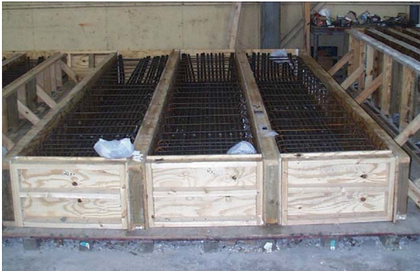
Figure 2.5 Cages placed in forms (set II)
