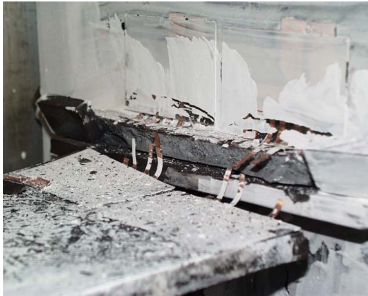
Figure 4.23 Distributed Switches after Failure of Top Beam Flange in the Fourth Shear Link Specimen
