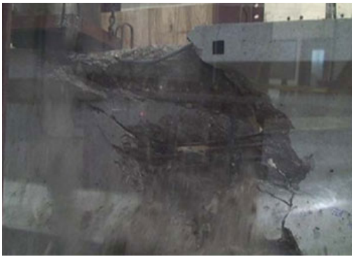
(c) Shear compression failure
