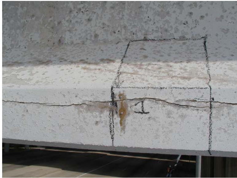
Figure 7.27: Close-up view of Point 1, Beltway 8 structure (6/22/01)
