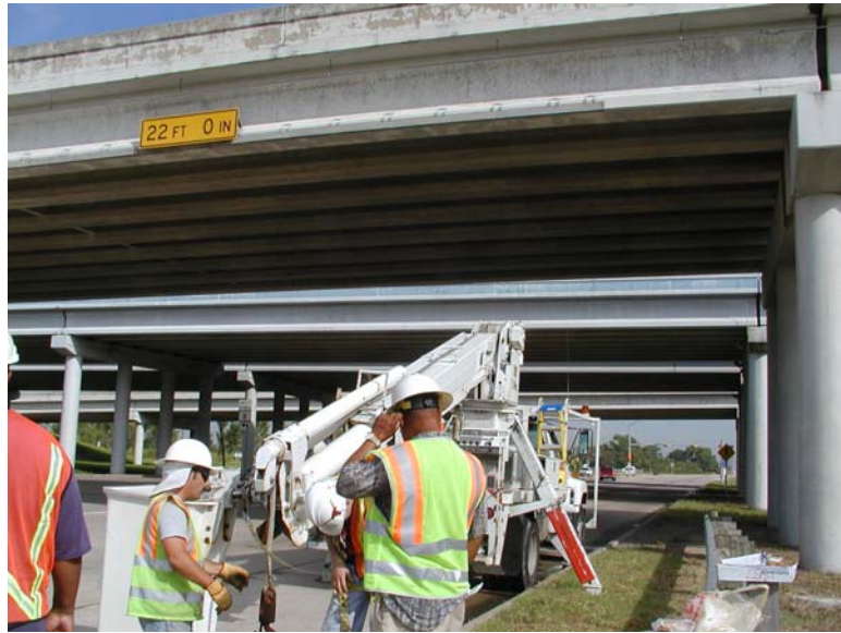
Figure 6.7: Beltway 8 over State Highway 3, Houston, Texas (facing north)
