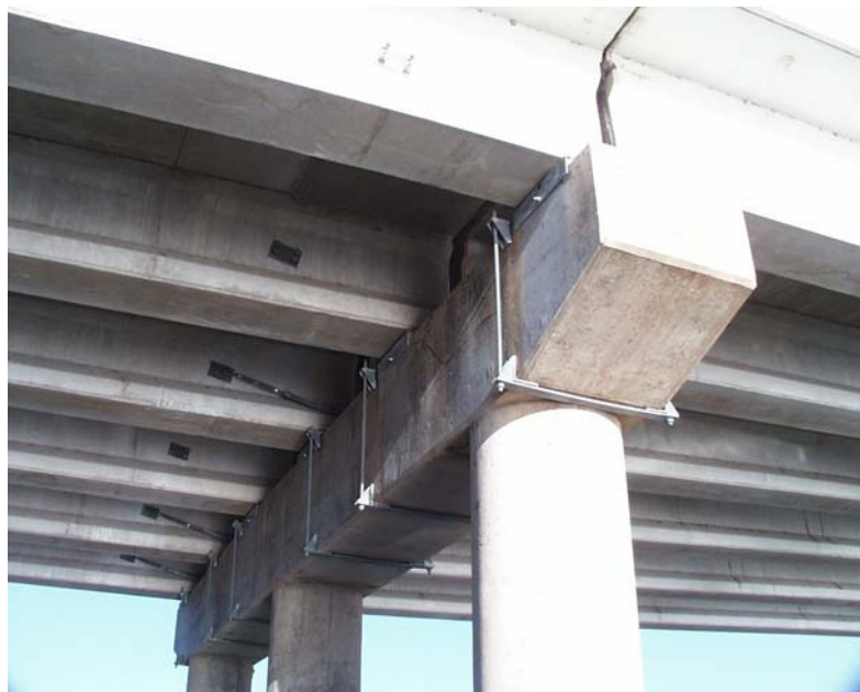
Figure 7.36: Overall view of Bent 5 (facing north)
