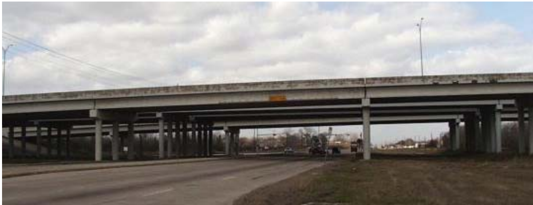
Figure 7.23: Overview of Beltway 8 over State Highway 3 (facing north)
