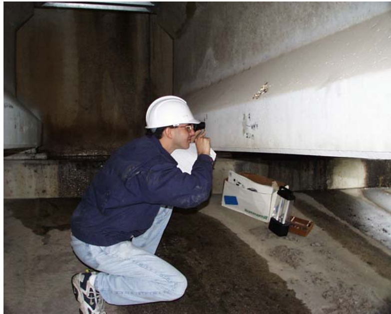
Figure 6.11: Measuring crack widths with optical scope
