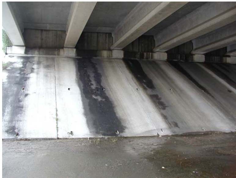
Figure 6.2: Overview of West Abutment of I-10 structure in Beaumont, Texas
