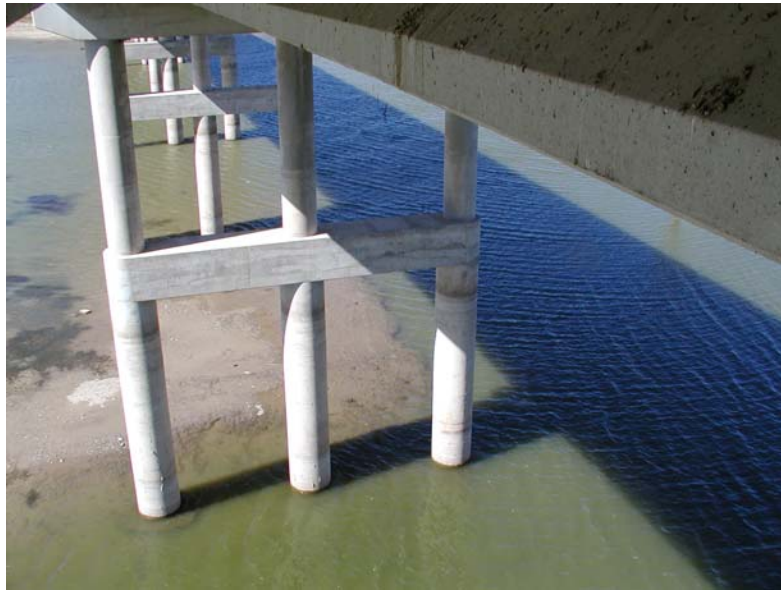
Figure 7.38: Overall view of Bent 9 (facing west)
