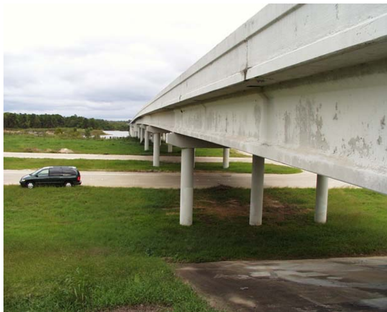
Figure 6.3: US-90 over the San Jacinto River near Houston, Texas
