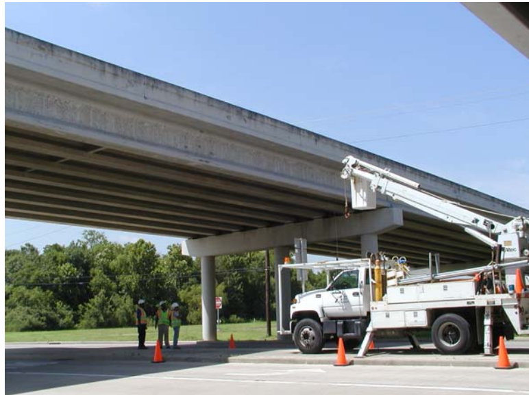
Figure 6.8: Beltway 8 over State Highway 3, Houston, Texas (facing west)
