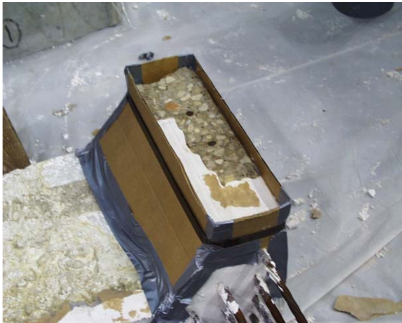
Figure 3.26: Cardboard formwork for top of web
