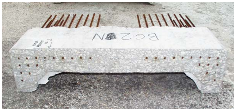
Figure 3.6: Back view of slice cut from Girder BG2N
