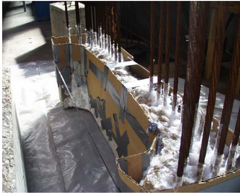
Figure 3.24: Cardboard formwork used for front face
