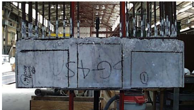
Figure 3.36: Representative areas for bottom face damage indices
