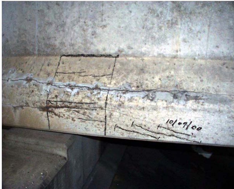
Figure 7.4: Representative areas on I-10 SW Girder 2, south face (10/7/00)
