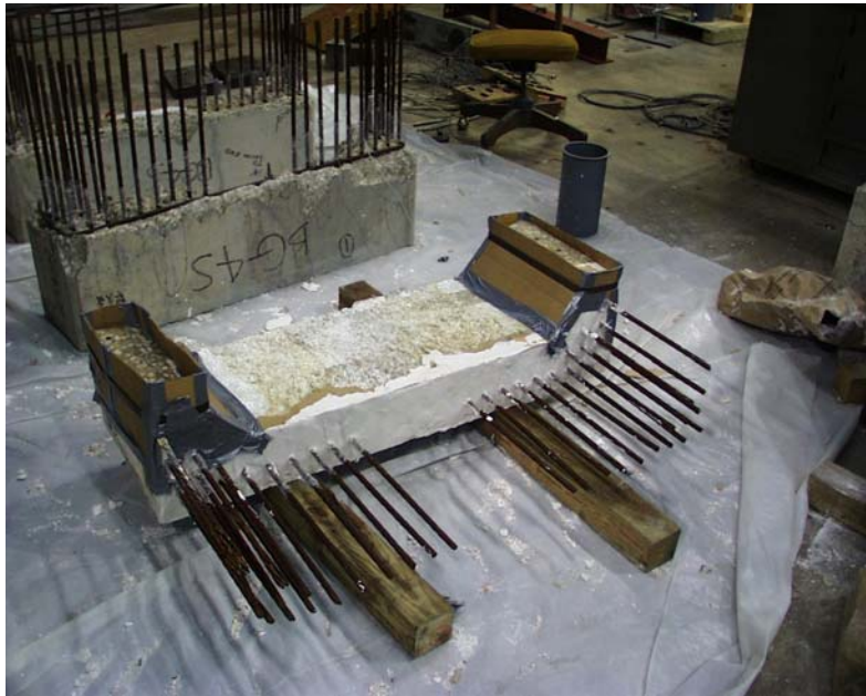
Figure 3.25: Formwork for web sections
