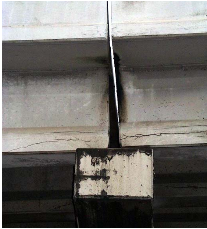
Figure 7.5: Cracks at first bent east of west abutment, I-10 (10/7/00)
