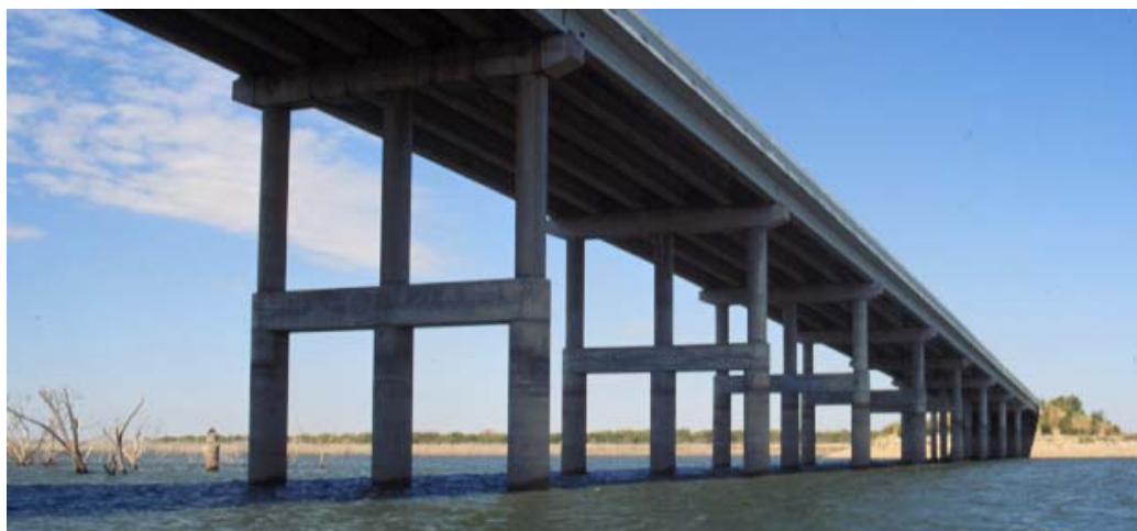
Figure 6.9: FM 1929 over the Lake Ivie Reservoir in Concho, Texas (facing west)
