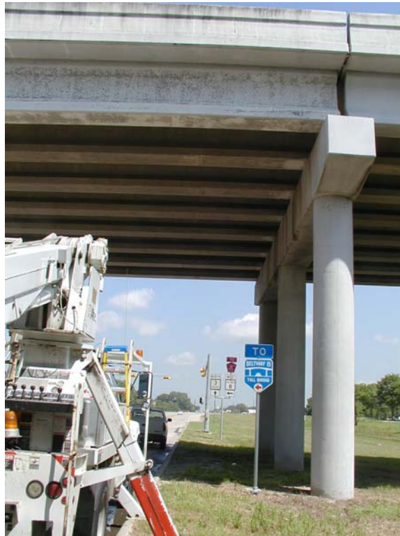
Figure 7.29: Overall view of Point 7, Beltway 8 structure (facing north) (6/22/01)
