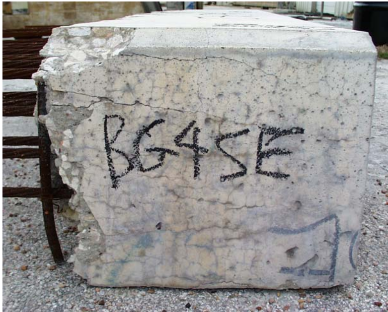
Figure 3.18: Cracking on left face of Slice BG4S1
