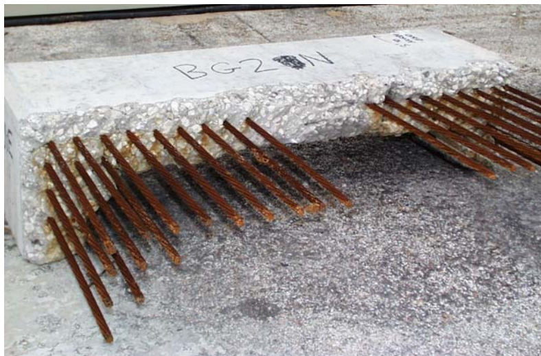
Figure 3.5: Front view of slice cut from Girder BG2N
