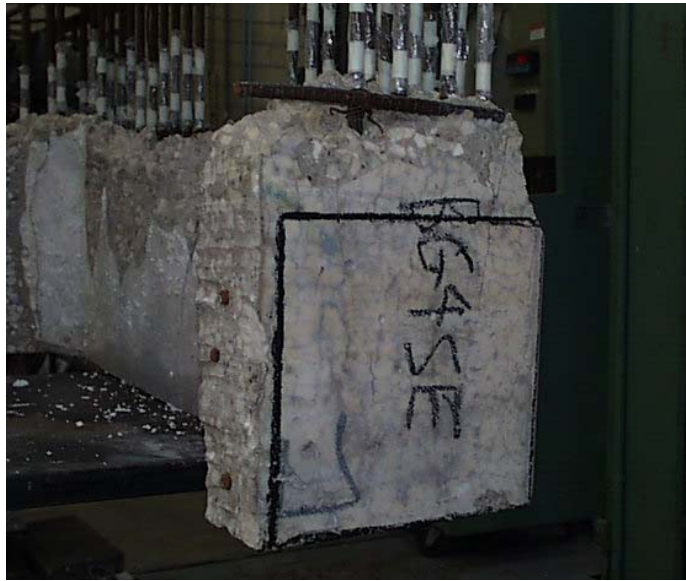
Figure 3.37: Representative square for left side damage index
