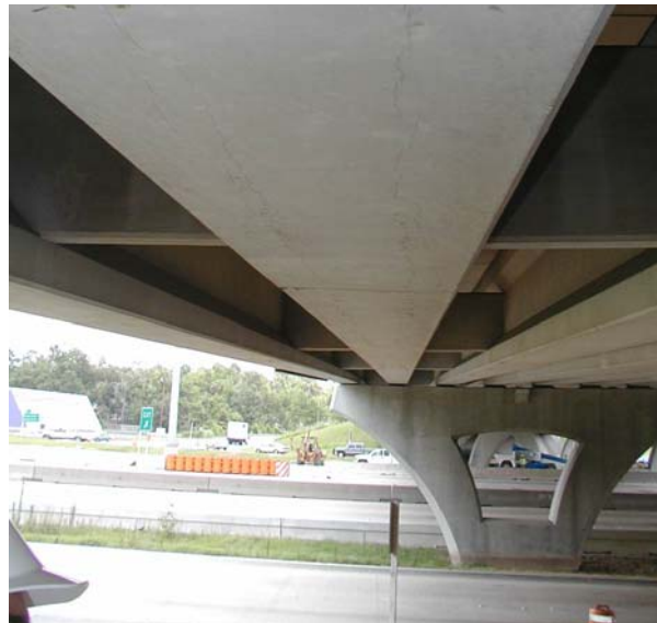
Figure 6.6: Underside of Robinson Road over I-45 (facing east)
