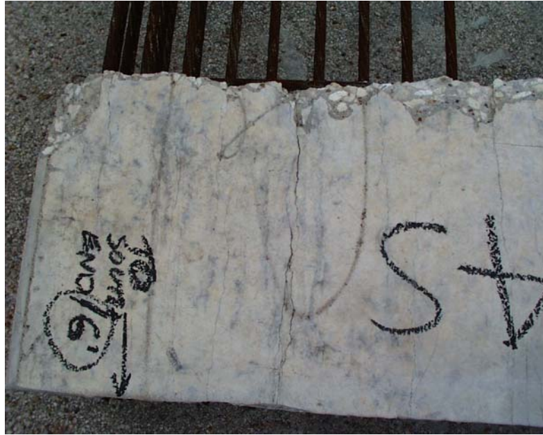
Figure 3.17: Cracking on bottom face of Slice BG4S1
