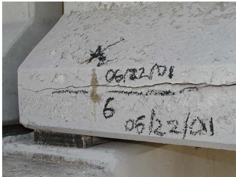
Figure 7.28: Close-up view of Point 6, Beltway 8 structure (6/22/01)
