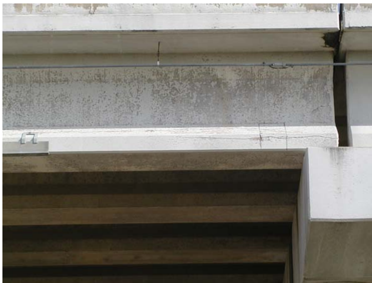
Figure 7.26: Overall view of Point 1, Beltway 8 structure (facing north) (6/22/01)
