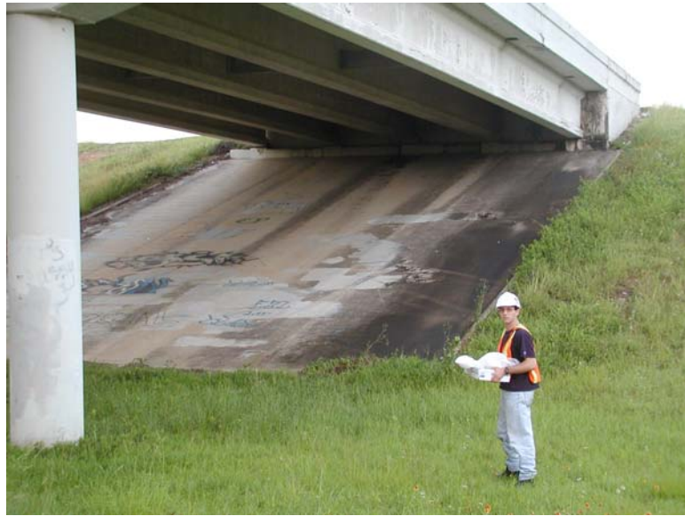
Figure 6.4: West Abutment of US-90W bridge over the San Jacinto River
