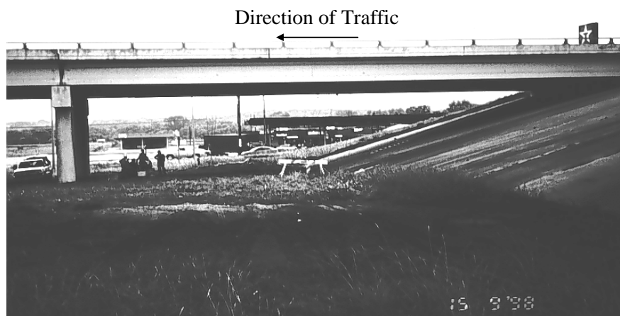
Figure 2.10 Side View of the Instrumented Span at the Nolanville Bridge
