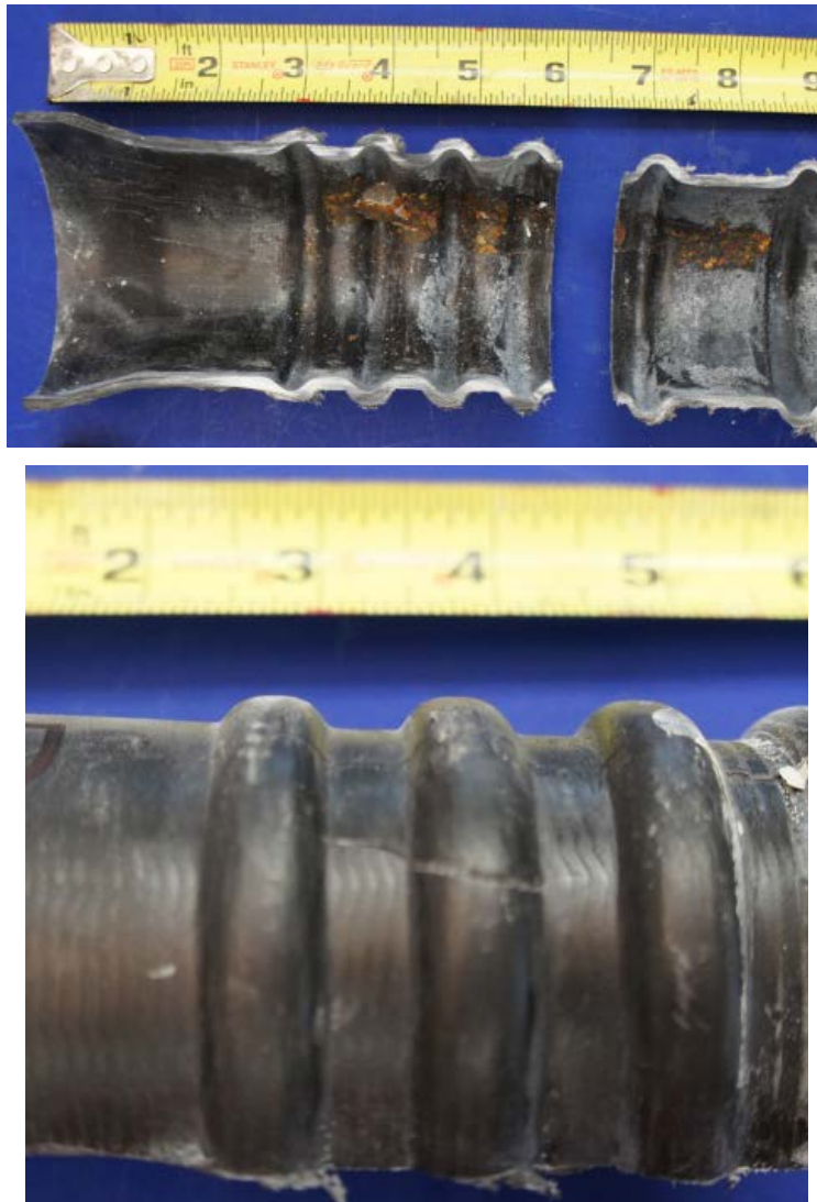
Figure 6.134: Rust Stains on Duct (Top) and Crack in Duct (Bottom) Located at the Dead End Grout Vent of Specimen 7.2
