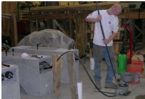
Figure 2.12: Grouting in Progress 1
