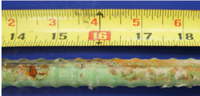
Figure 6.132: Moderate Corrosion and Crack in Epoxy Coating along Longitudinal Rib of South Epoxy Coated Longitudinal Bar of Specimen 7.2
