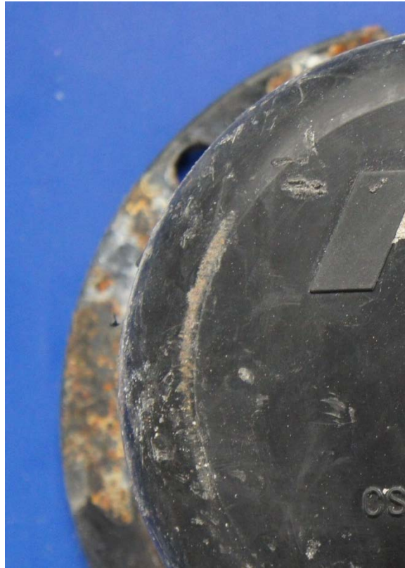
Figure 6.173: Rust Stains on Lip of Live End Group Cap from Specimen 7.4
