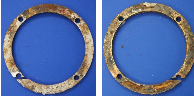
Figure 6.140: Severe Corrosion and Pitting on Steel Ring from the Dead End of Specimen 7.2
