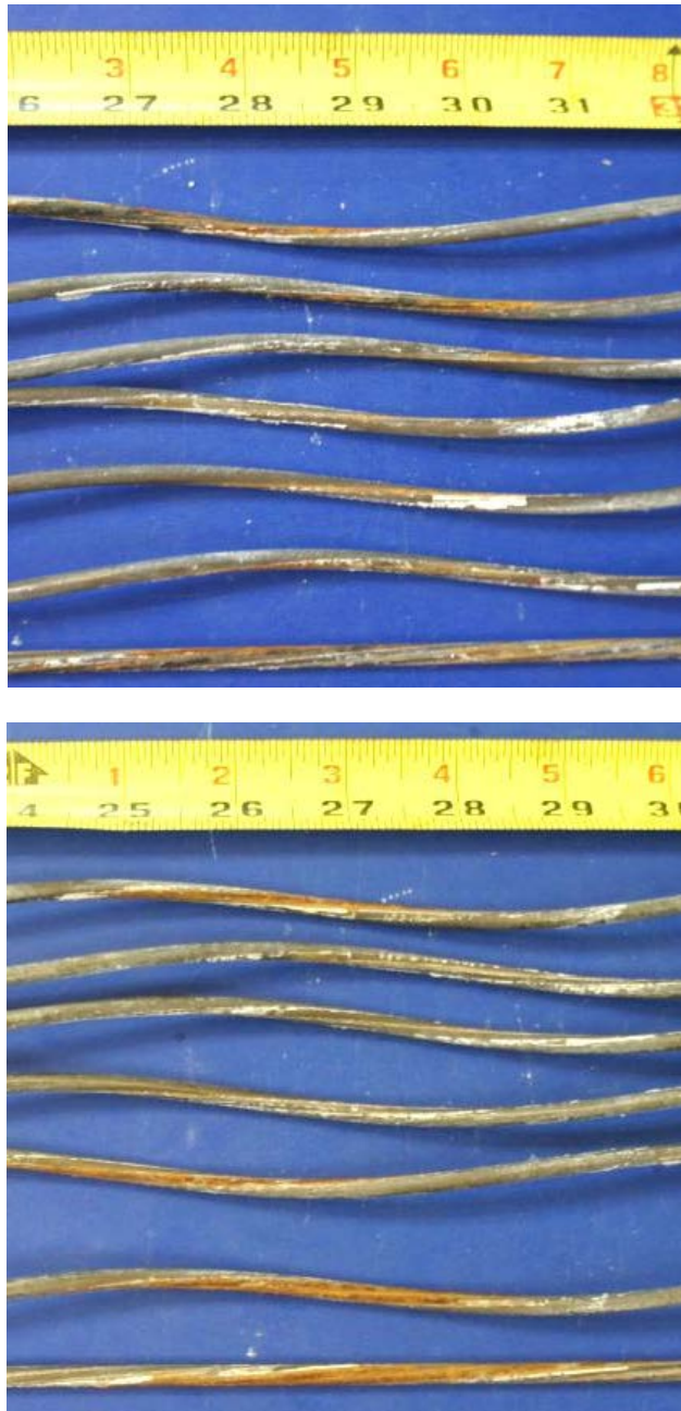
Figure 6.53: Moderate Corrosion on Outer and Inner Wires of Strands from the North (Top) and South (Bottom) Tendon of Specimen 2.3
