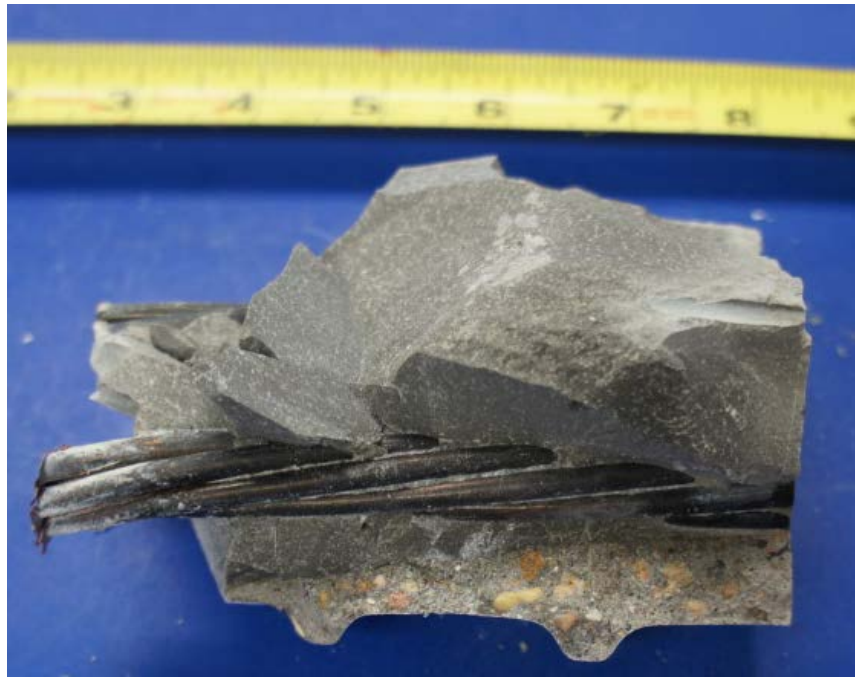
Figure 6.69: Concrete in Grout from the Dead End of the North Tendon of Specimen 3.3
