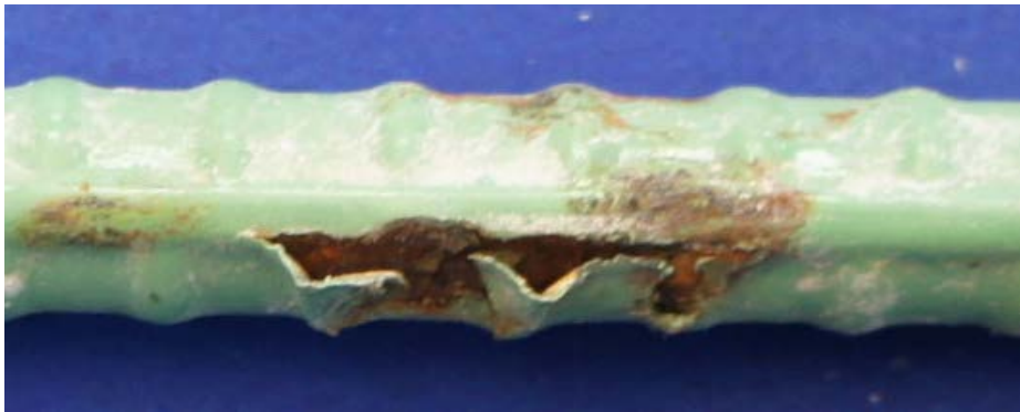
Figure 6.154: Pitting on Transverse Bar #3 from Specimen 7.3
