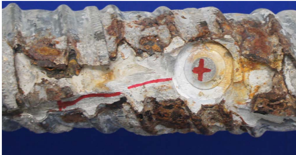
Figure 6.77: Staining on Gout from Specimen 4.1
