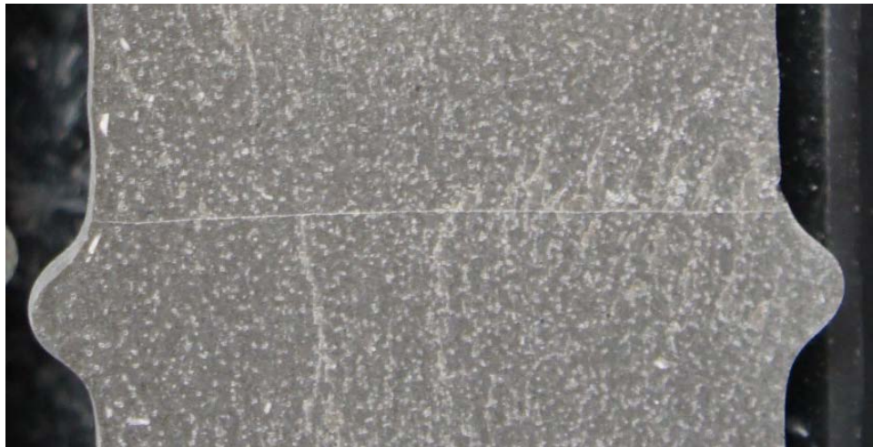
Figure 6.156: Small Transverse Crack in Grout from Specimen 7.3
