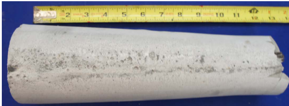
Figure 6.145: Small Voids in Grout from Dead End Tendon Section of Specimen 7.2
