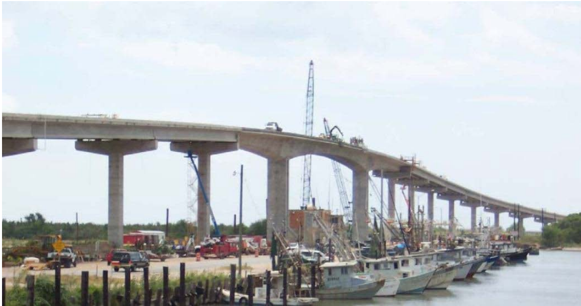
Figure 8.1: FM 2031 Bridge over GIWW in Matagorda, Texas 2
