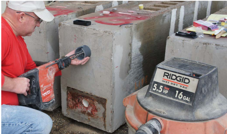
Figure 4.8: Concrete Powder Extraction with Hammer Drill
