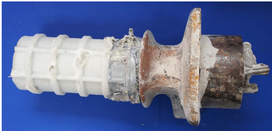
Figure 2.10: GTI Two-Way Plastic Duct Slipped Over the Anchorage Plate Cone
