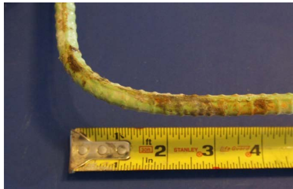
Figure 6.40: Moderate Corrosion on the Corner of Transverse Bar #4 from Specimen 1.4
