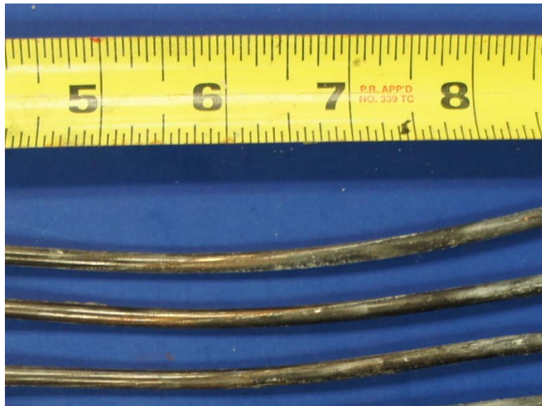
Figure 6.66: Very Dark Brown Discoloration of Copper Cladding on Strand from Specimen 3.3
