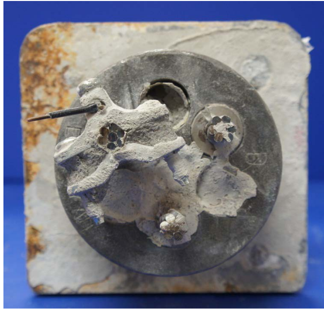
Figure 6.104: Light Surface Corrosion where Epoxy had Debonded from Exposed Face of North Live End Anchorage Plate from Specimen 5.1
