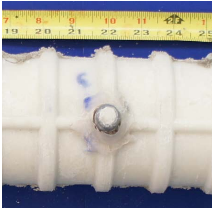
Figure 6.64: Silicone Debonded from Grout Vent of South Duct from Specimen 3.3
