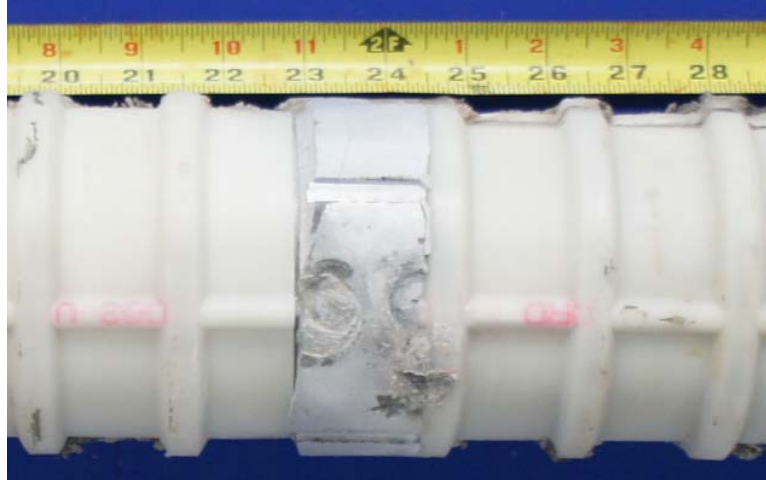
Figure 6.120: Top Outer Surface at Midspan of North Duct from Specimen 5.3
