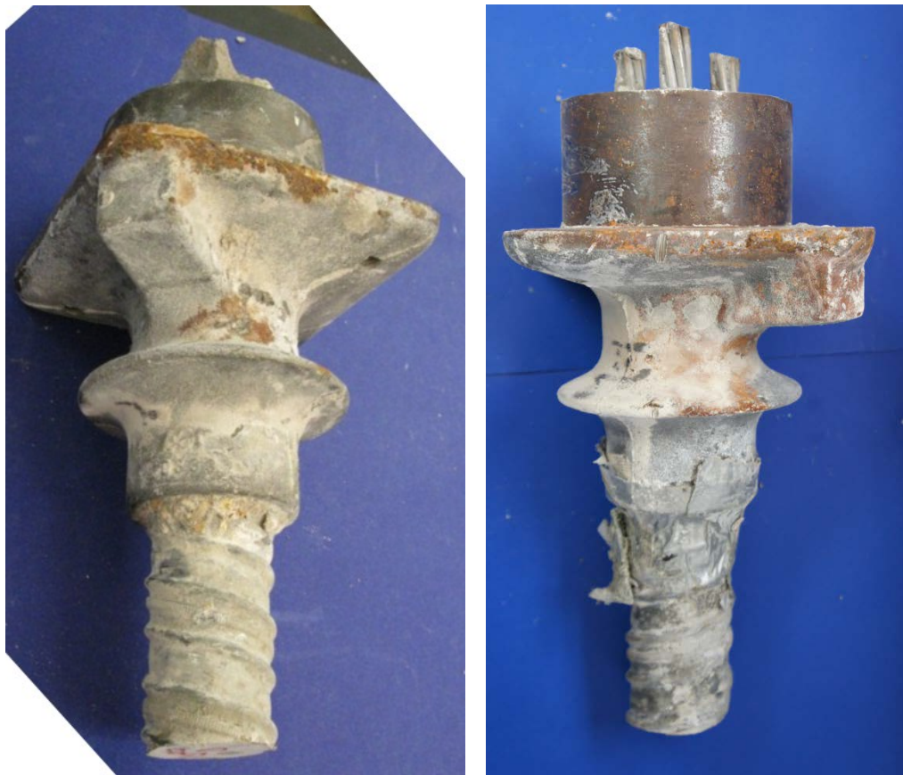
Figure 7.25: Typical Anchorage from 4 Year 2 (Left) and 6 Year (Right) Autopsy Periods
