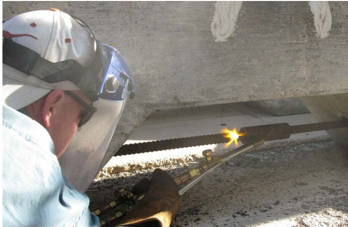
Figure 6.2: Cutting Dywidag Bar to Unload Specimen
