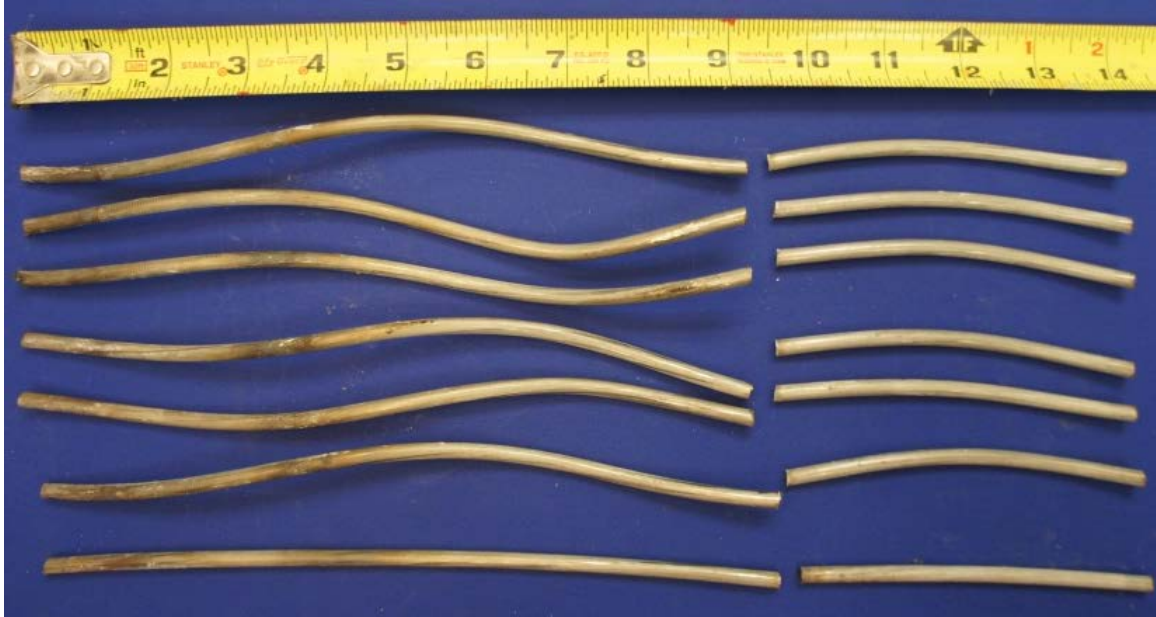
Figure 6.81: Discoloration of Stainless Steel Wires from the South Tendon in the Dead End Anchorage of Specimen 4.1
