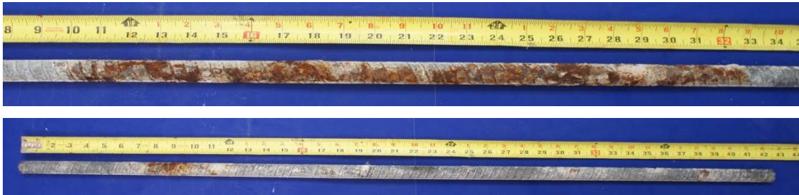
Figure 6.133: Corrosion Damage to North (Top) and South (Bottom) Uncoated Longitudinal Bars from Specimen 7.2
