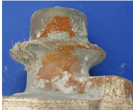
Figure 6.114: Light Corrosion on the Embedded Portion of the North Dead Anchorage Plate from Specimen 5.2
