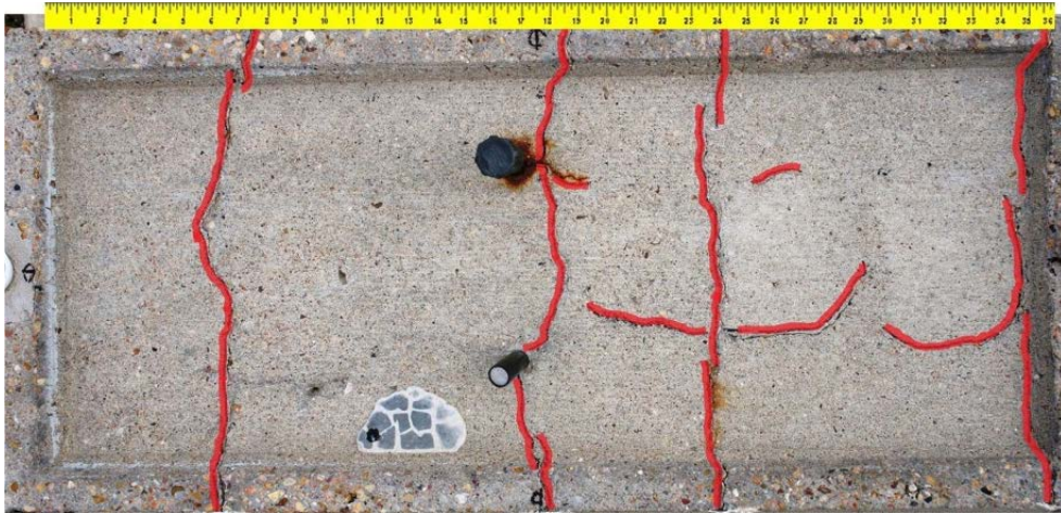
Figure 6.38: Specimen 1.4 Crack Map of Ponding Area
