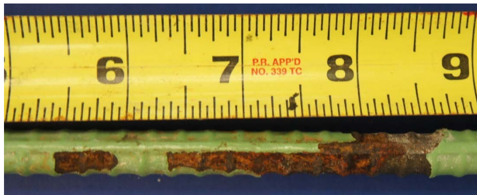
Figure 6.88: Crack in Epoxy Coating along the Longitudinal Rib (Top) and Moderate Corrosion at the Crack along the Longitudinal Rib (Bottom) on #6 Transverse Bar from Specimen 4.3
